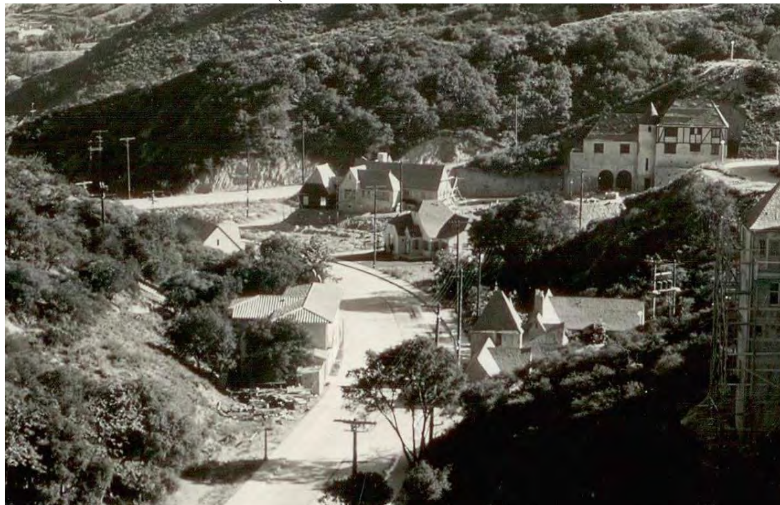
UNDER CONSTRUCTION (ACROSS FROM TURRET AND DOUBLE ARCHES)
