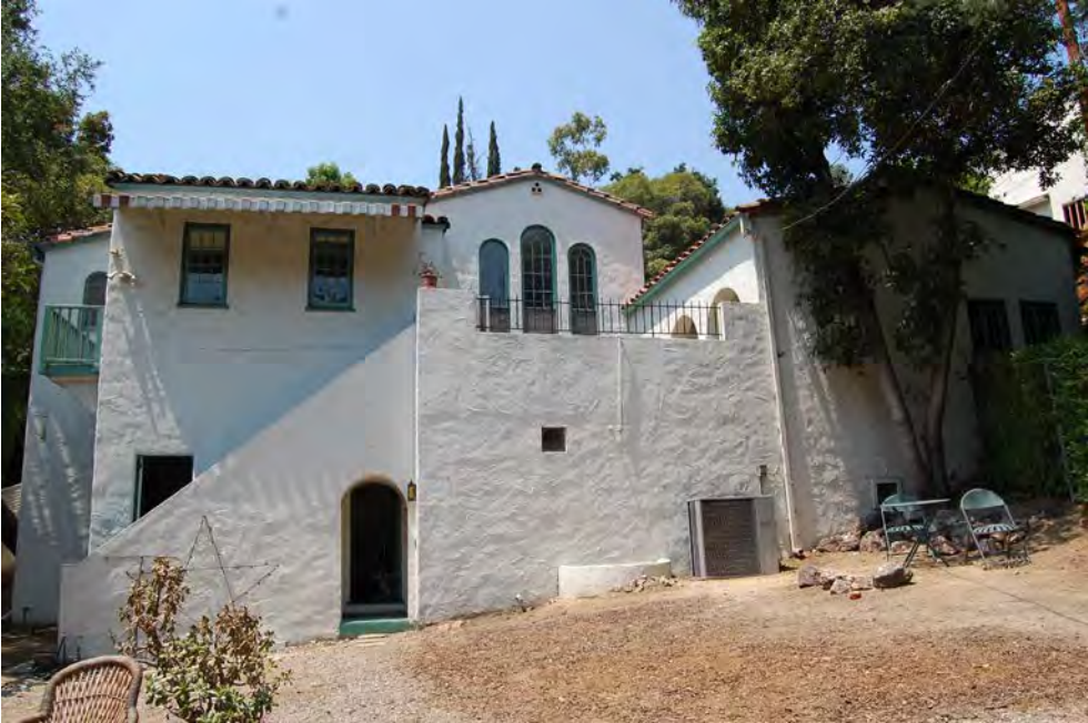
REAR ELEVATION—FACING SOUTH
