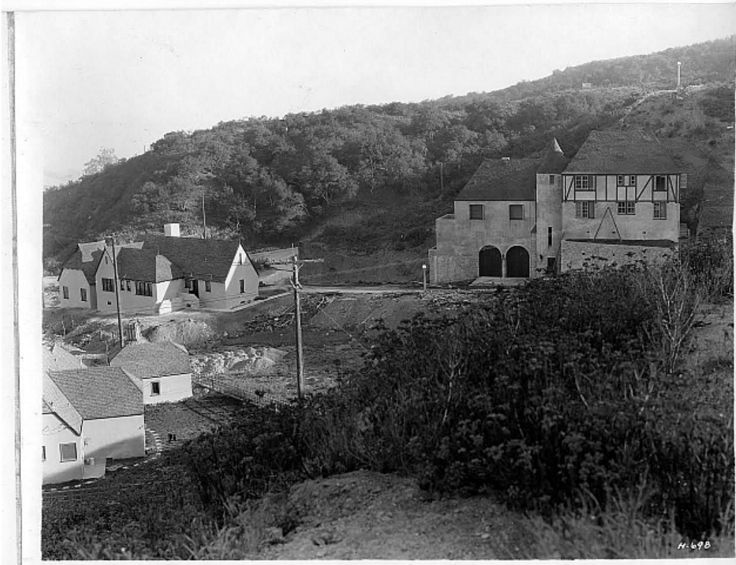
PROPERTY JUST PRIOR TO CONSTRUCTION (EMPTY LOT IN CENTER)
