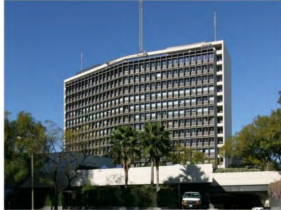
FIGURE 37. Union Oil Headquarters, 1958
