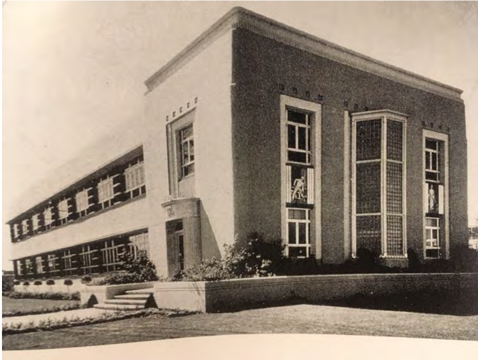
FIGURE 11. ALCOA Headquarters, Vernon
