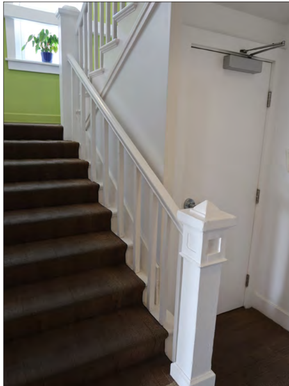
Image 22: First to second floor stairwell, view northeast (Chattel, 2017)
