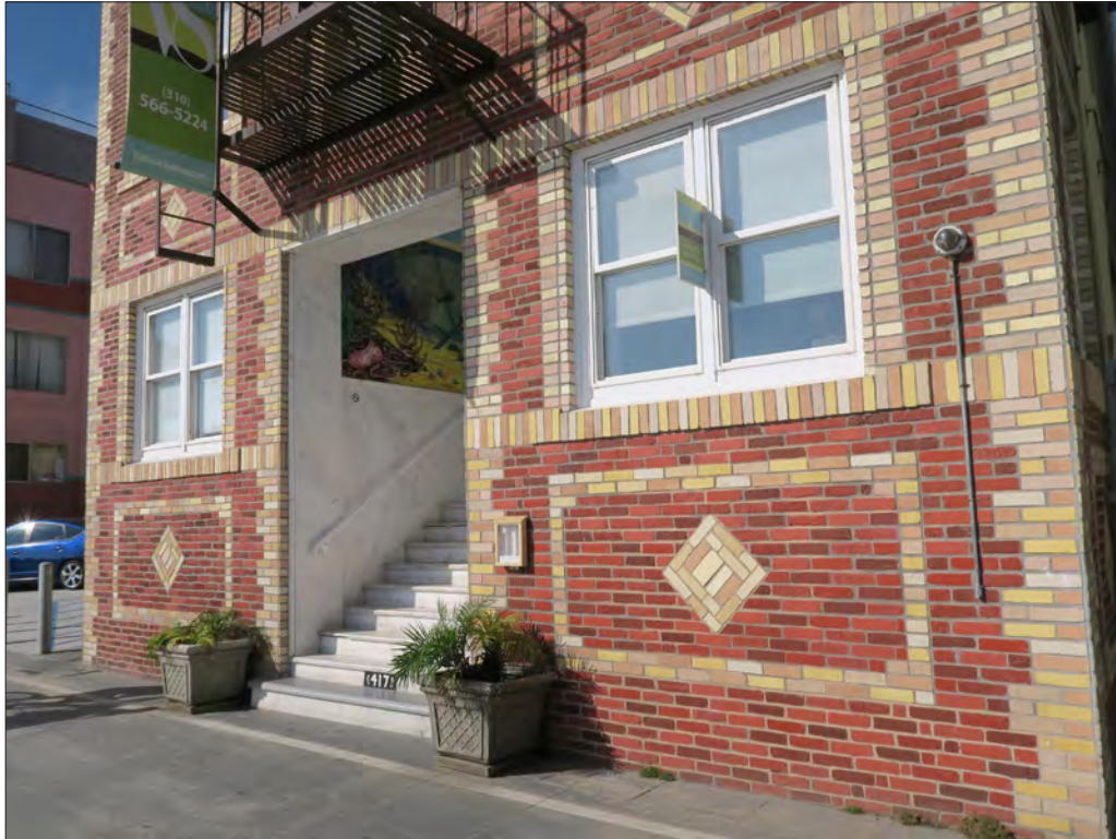
Image 9: West elevation, recessed central entryway, view northeast (Chattel, 2017)
