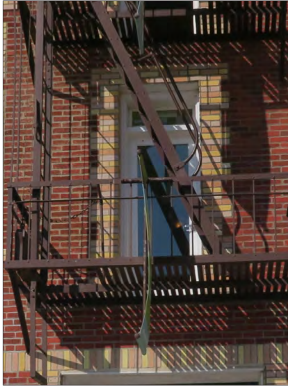
Image 11: West elevation, wood door to fire escape, view northwest (Chattel, 2017)
