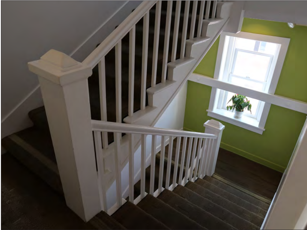
Image 23: Second to first floor stairwell, view north (Chattel, 2017)
