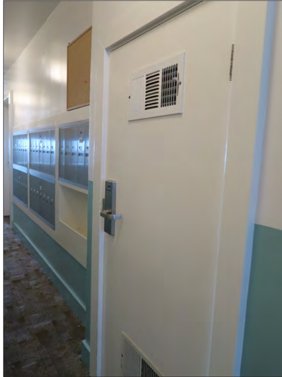
Image 21: First floor , mechanical closet door (Chattel, 2017)
