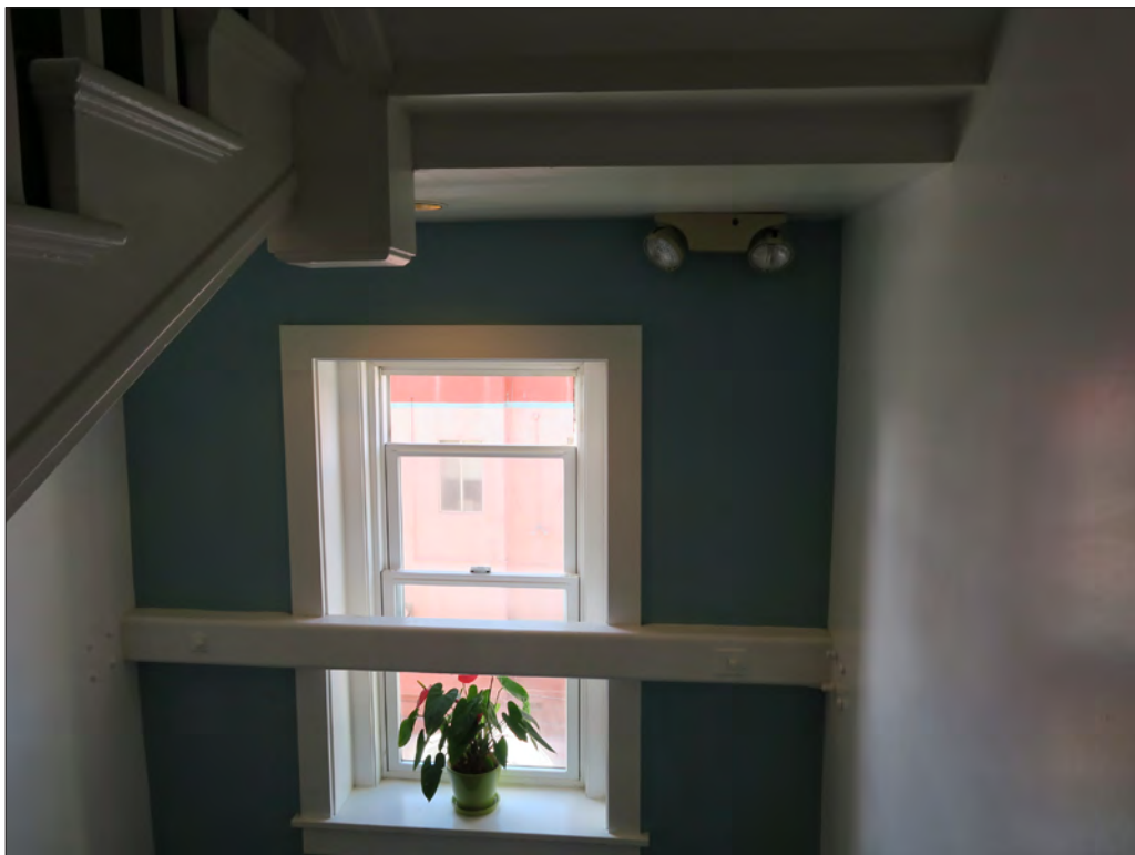
Image 36: Typical seismic reinforcement in stairwell (Chattel, 2017)
