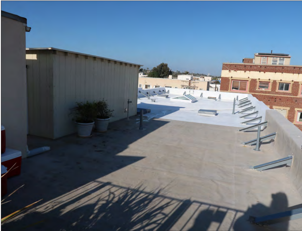
Image 35: Roof, view east (Chattel, 2017)
