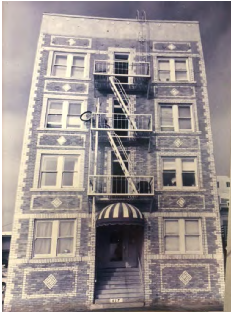
Image 44: Subject property, west elevation, cornice removed (Carl Lambert, 1997)
