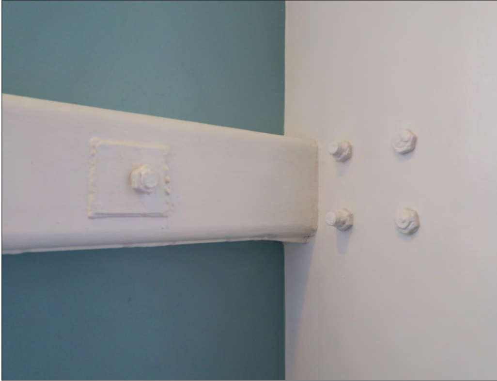
Image 37: Typical detail of seismic reinforcement in stairwell (Chattel, 2017)
