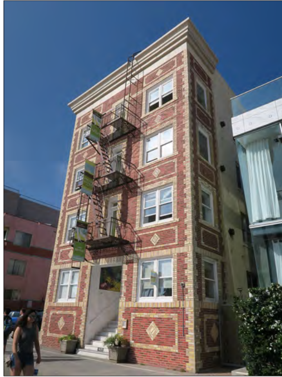
Image 3: West elevation, southwest corner, view northwest (Chattel, 2017)
