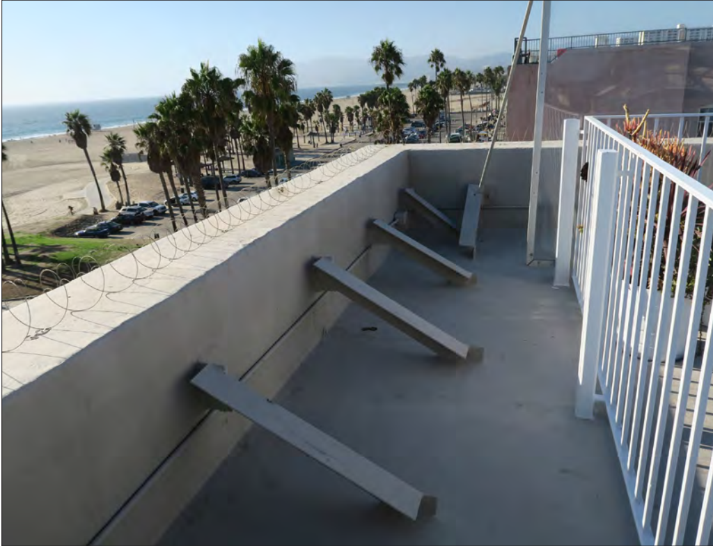
Image 33: Roof, parapet, view north (Chattel, 2017)
