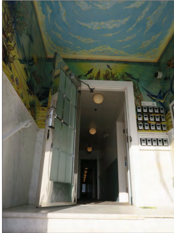
Image 13: West elevation, recessed central entryway, view northeast (Chattel, 2017)
