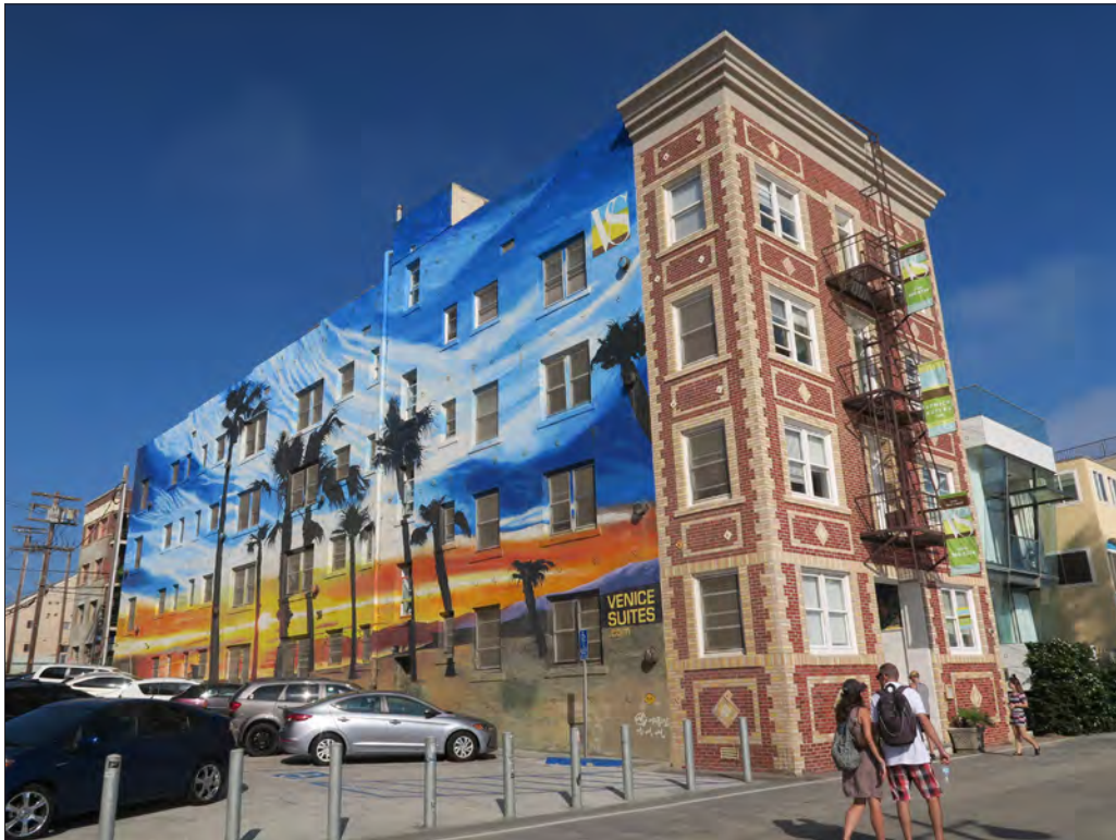
Image 4: North elevation, view southeast (Chattel, 2017)
