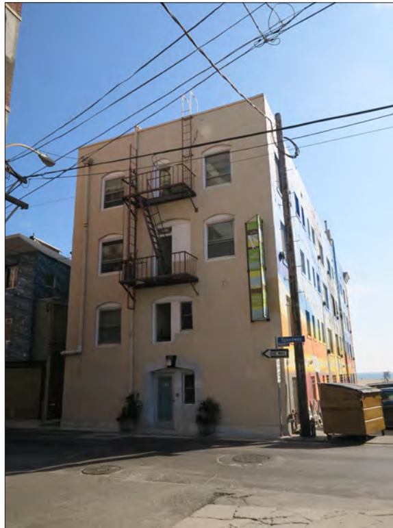
Image 6: East elevation, view southwest (Chattel, 2017)
