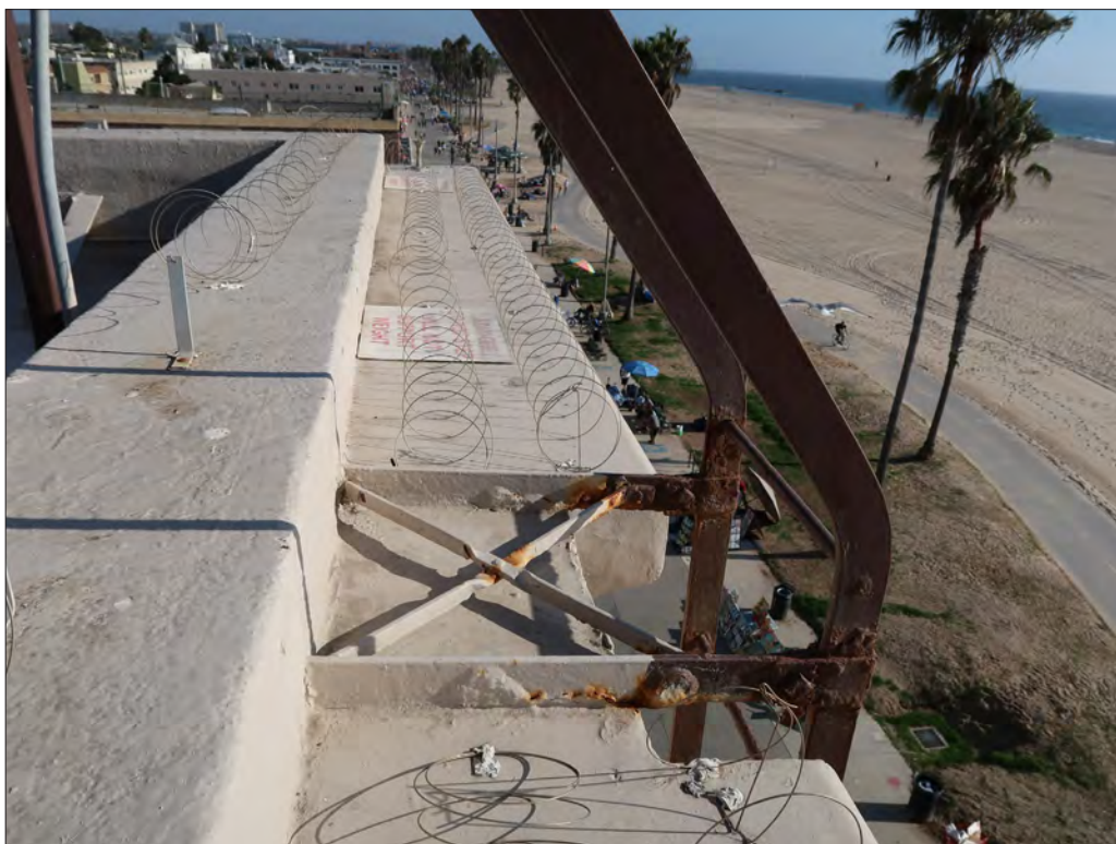
Image 34: Roof, parapet and fire escape, view south (Chattel, 2017)
