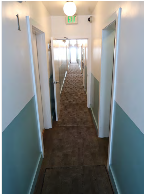
Image 14: First floor, typical hallway, view east (Chattel, 2017)
