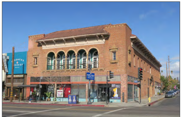
Current view of building. Note shortened parapets (ARG, 2018)
