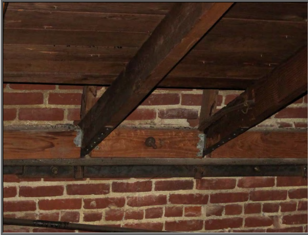
Photo 9: Retrofit wall anchorage connection at roof rafters.
