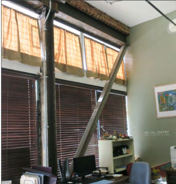
Interior of storefront, 5577 North Figueroa Street; note steel bracing installed during seismic retrofit (ARG, 2018)
