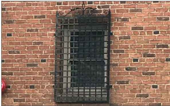
Wood double-hung window with metal grille, northeast elevation (ARG, 2018)
