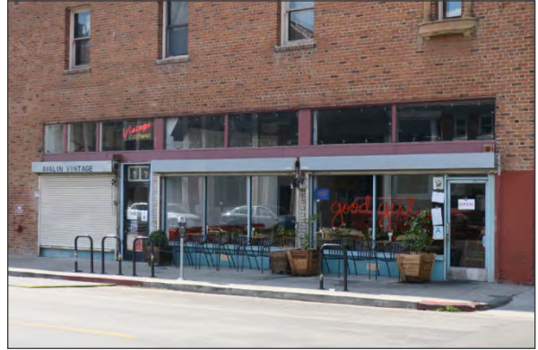
Current view of storefronts at west end of northeast elevation (ARG, 2018)
