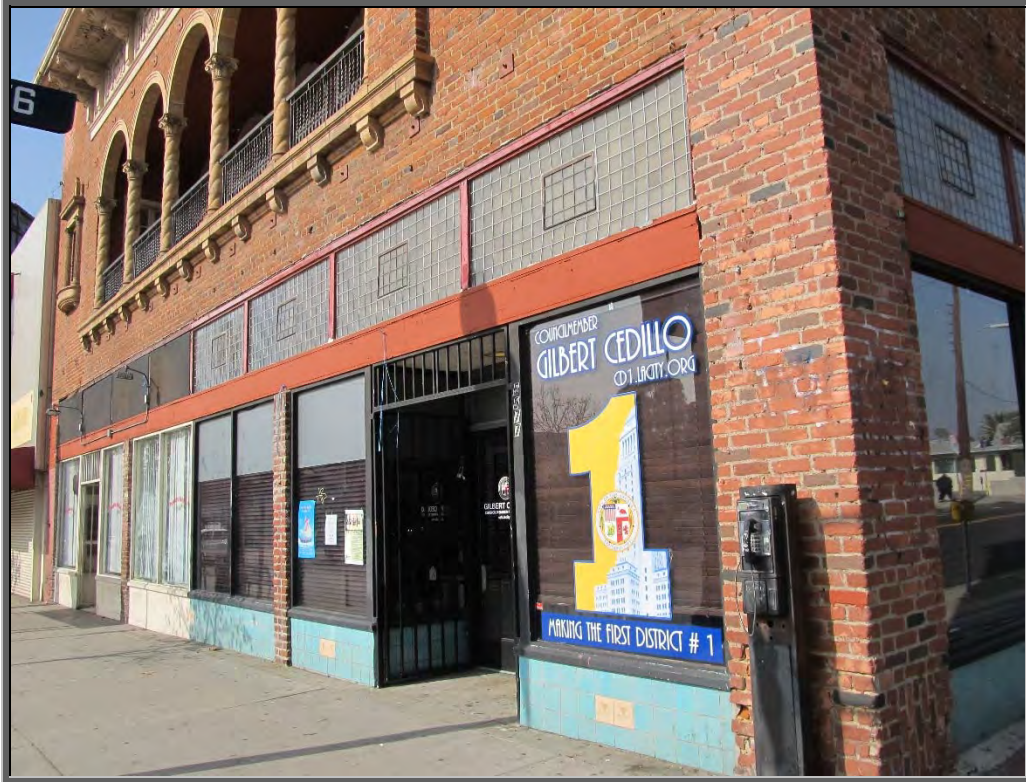
Photo 1: South storefront elevation.
