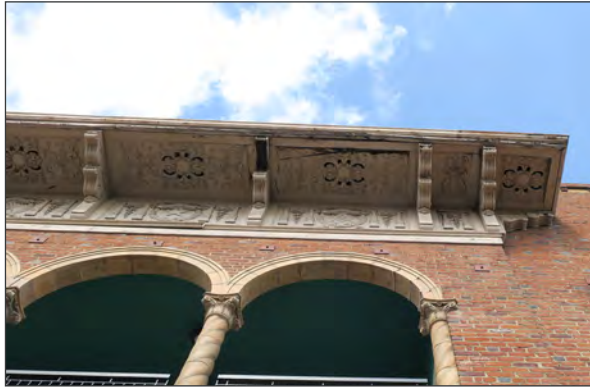
Detail of cornice and frieze (ARG, 2018)
