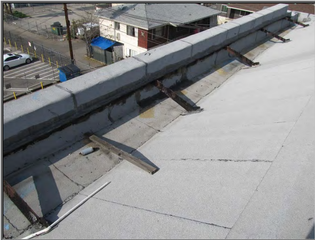
Photo 6: Retrofit parapet bracing.
