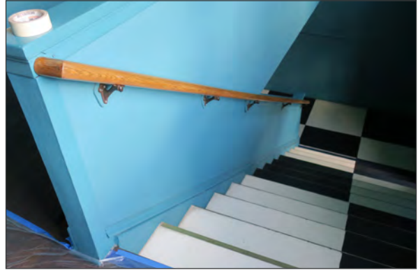
Detail of main entry stairs. Note vinyl treads and wood handrail (ARG, 2018)
