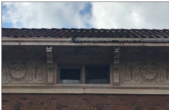
Paired wood casement windows at third floor frieze, northeast elevation (ARG, 2018)
