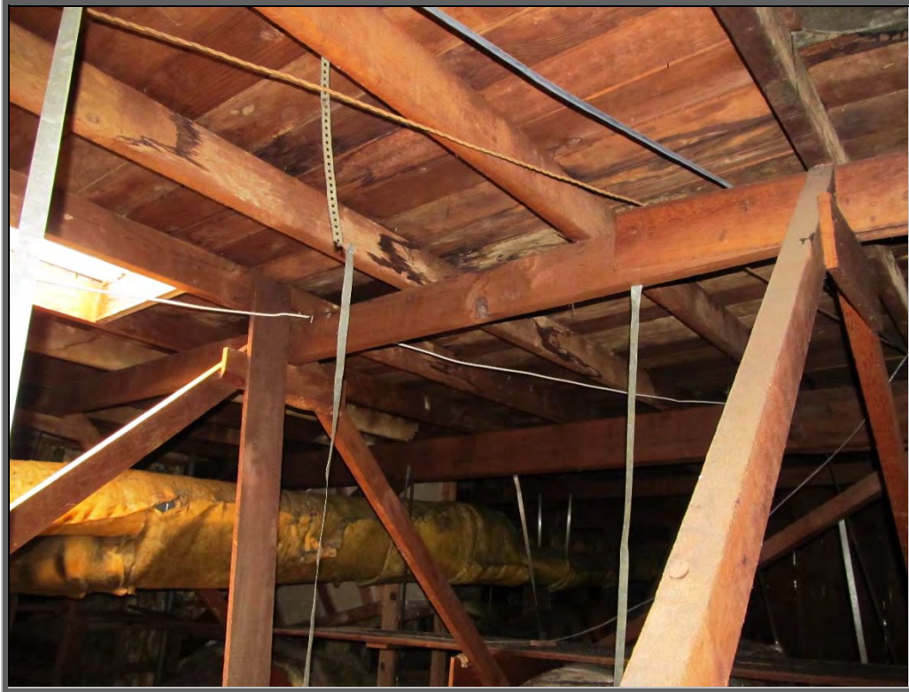
Photo 7: Main roof framing.
