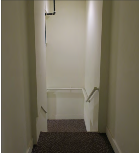
Stairs at southwest end of third story corridor (ARG, 2018).
