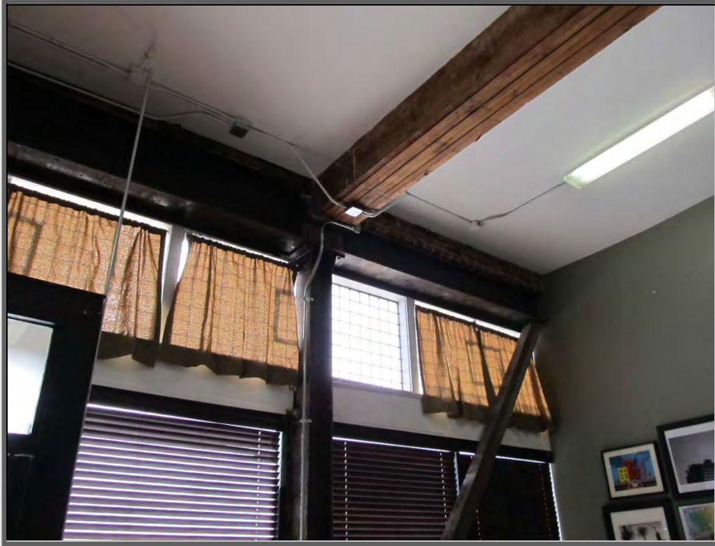
Photo 13: Storefront framing and retrofit braced frame.
