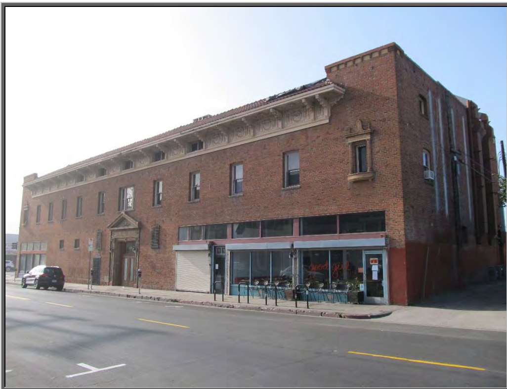
Photo 2: East exterior elevation.
