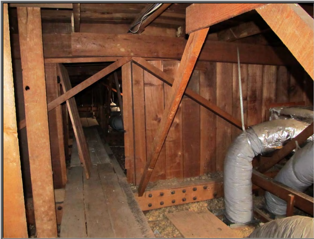
Photo 8: Typical bow-string roof truss and interior straight-sheathed shear wall.
