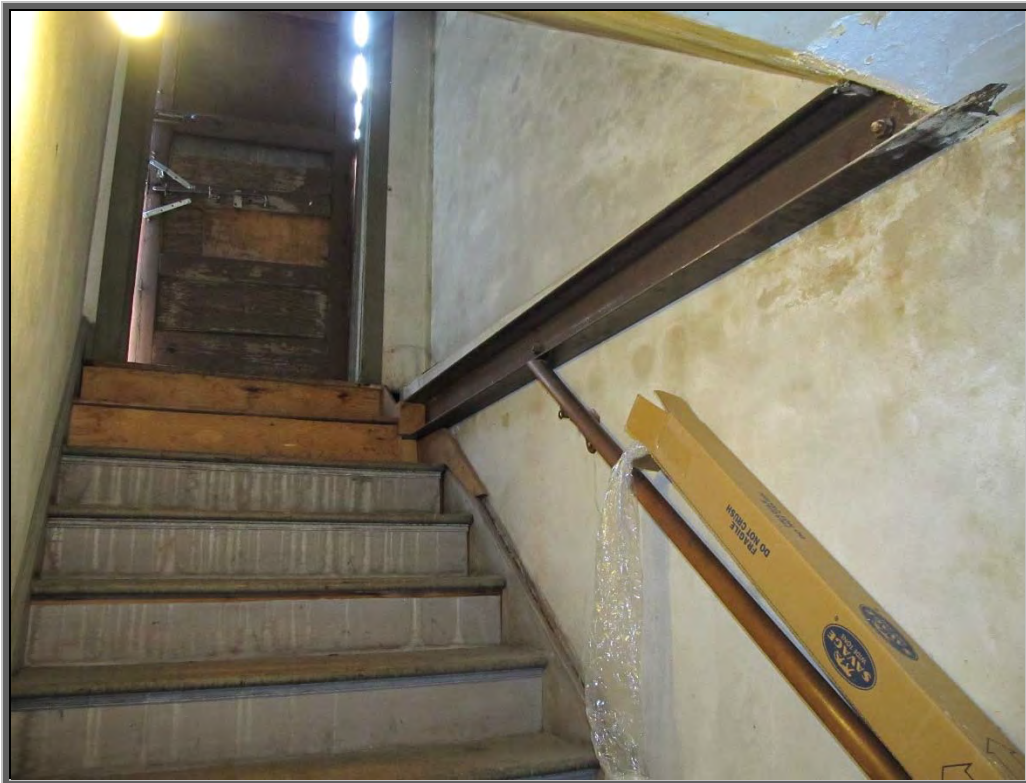
Photo 10: Retrofit steel channel wall anchorage connection within stairwell.
