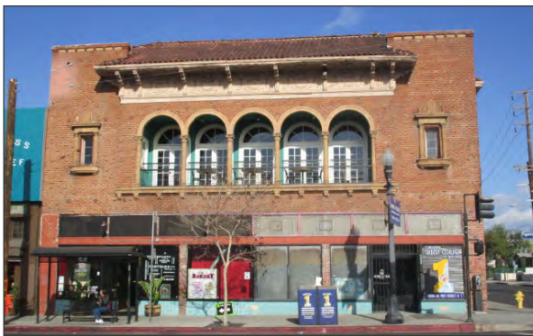
Current storefronts at southeast elevation; note original transoms remaining (ARG, 2018)
