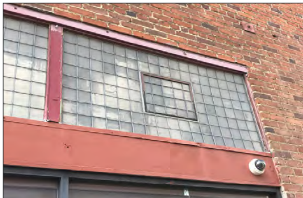
View of typical original leaded glass transom (ARG, 2018)
