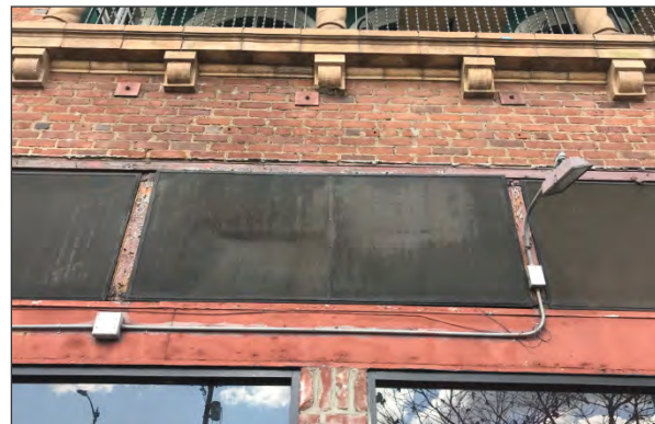
Portion of transoms at southeast elevation covered with painted plywood (ARG, 2018)
