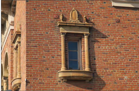
Terra cotta window surround on second story (ARG, 2018)
