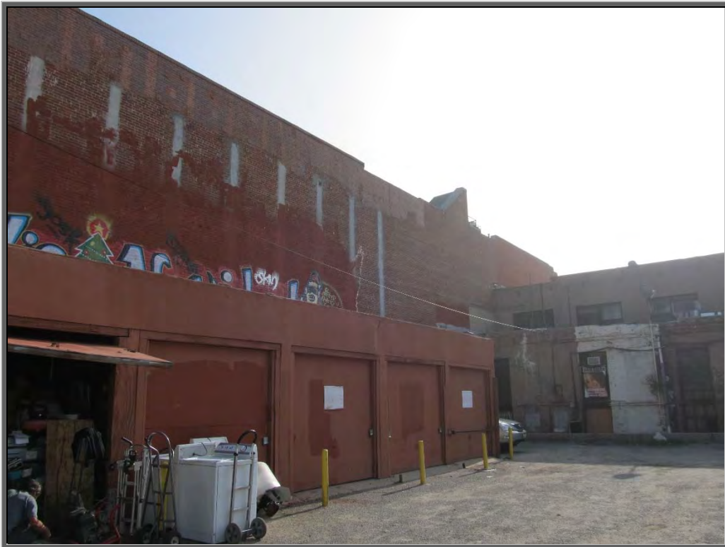
Photo 4: West exterior elevation.
