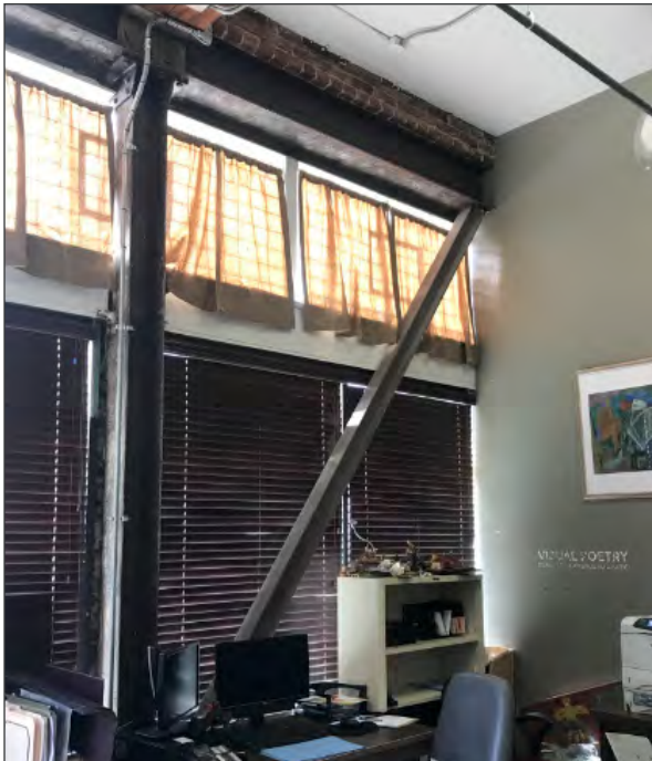
Steel framed brace at storefront, southeast elevation (ARG, 2018)
