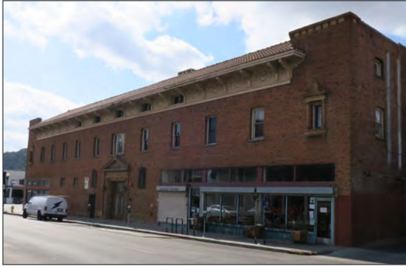
Northeast elevation, view south (ARG, 2018)
