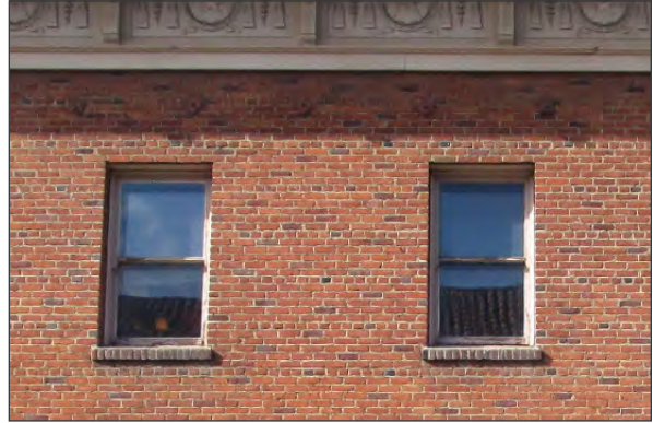
Typical original wood double-hung window at northeast elevation (ARG, 2018)
