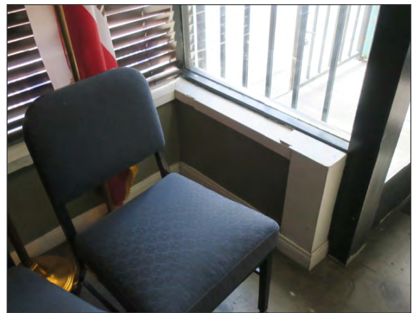
Interior view of storefront bulkhead/entry, 5577 North Figueroa Street (ARG, 2018)
