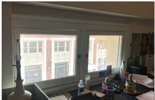
Interior view of paired wood casement windows (ARG, 2018)
