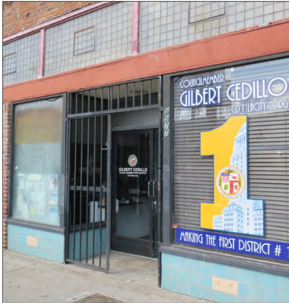
Entrance to 5577 North Figueroa Street; note aluminum storefront framing, gates and ceramic tile (ARG, 2018)
