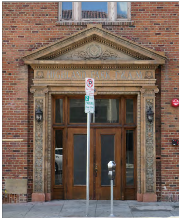
Articulated entrance on northeast elevation. These doors lead to upper-story spaces (ARG, 2018)
