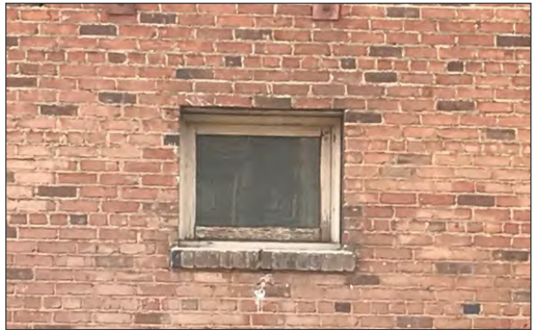
Wood awning window, northeast elevation (ARG, 2018)
