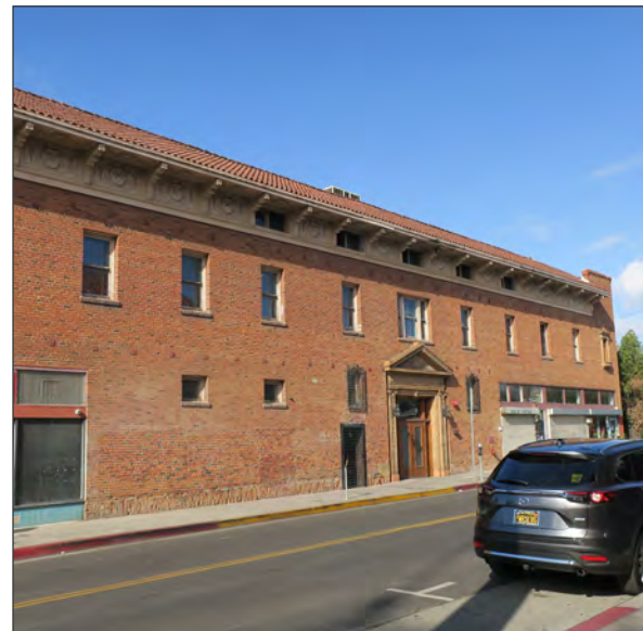
Current view of the northeast elevation (ARG, 2018)
