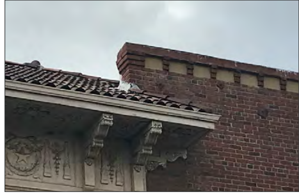
Built-in gutter at tiled roofs, view from street (ARG, 2018)
