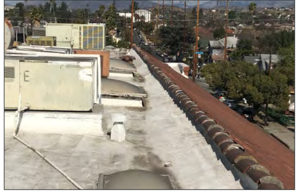
Membrane roof, view northwest. Note skylights and rooftop HVAC units (ARG, 2018)
