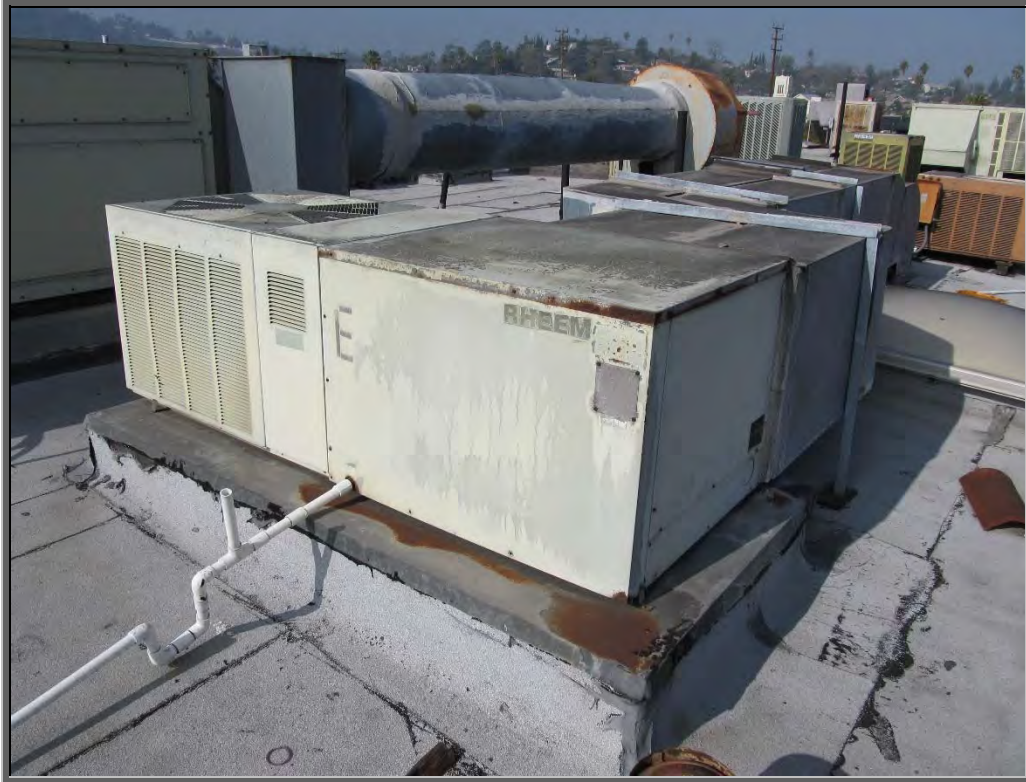
Photo 19: Marginal anchorage at existing rooftop units.
