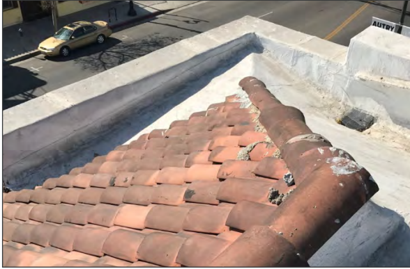
Tile roof at east corner of building (ARG, 2018)
