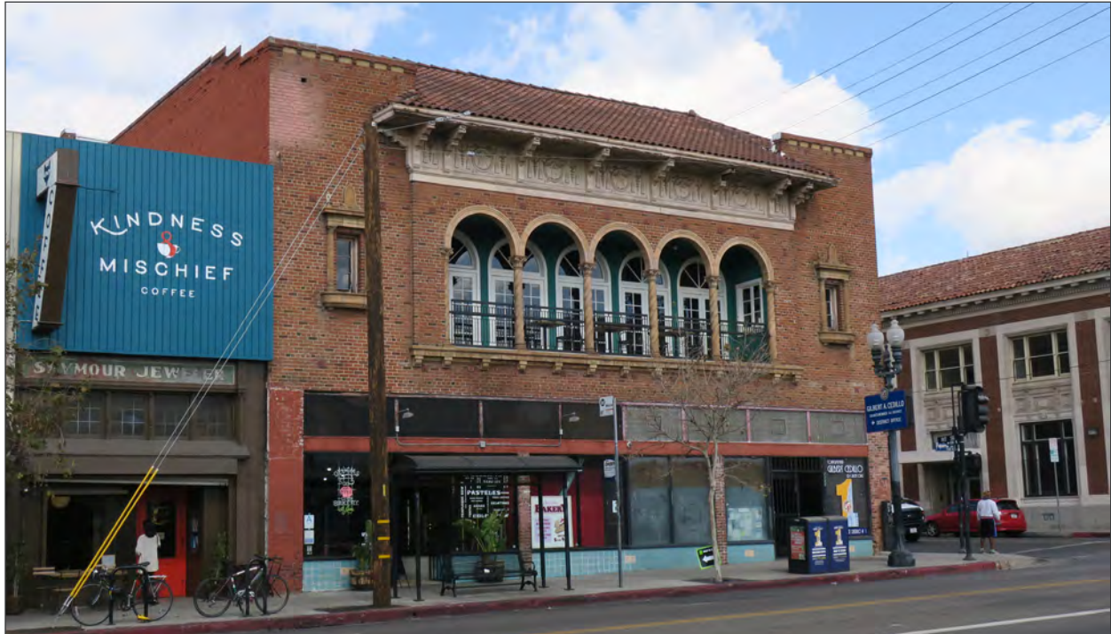
Primary (southeast) elevation as seen from Figueroa Street, view north (ARG, 2018)
