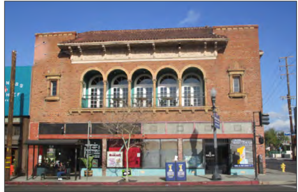
Brick exterior walls on primary (southeast) elevation (ARG, 2018)
