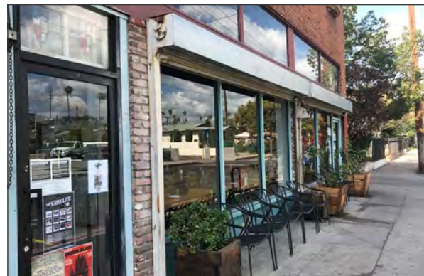
Storefronts on northeast elevation as seen from Avenue 56, view northwest (ARG, 2018)
