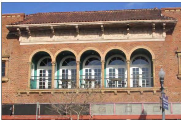
Balcony doors at southeast elevation (ARG, 2018)
