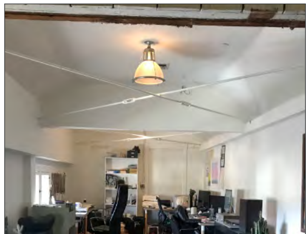
Tie rods at third floor interior (ARG, 2018)
