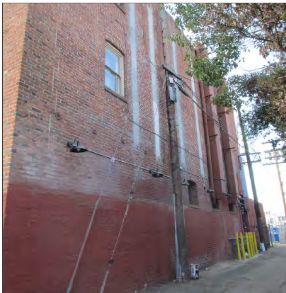
Northwest elevation. Note paint at ground level (ARG, 2018)
