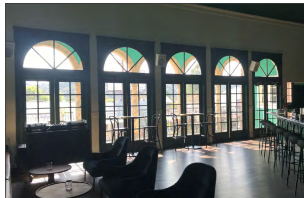
Interior view of balcony doors and transoms (ARG, 2018)
