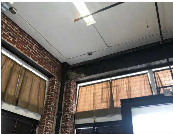
Interior view of storefront transoms, 5577 North Figueroa Street (ARG, 2018)
