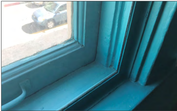
View of typical interior pane, added for sound control (ARG, 2018)
