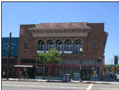
Primary, south elevation along North Figueroa St., view north
