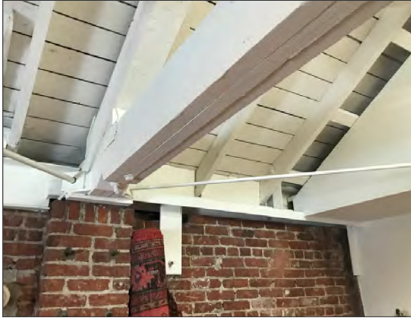
Wood bowstring truss and framing at third story interior (ARG, 2018)
