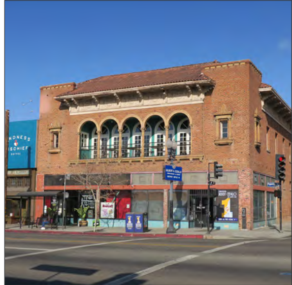
Current view of the primary (southeast) elevation (ARG, 2018)
