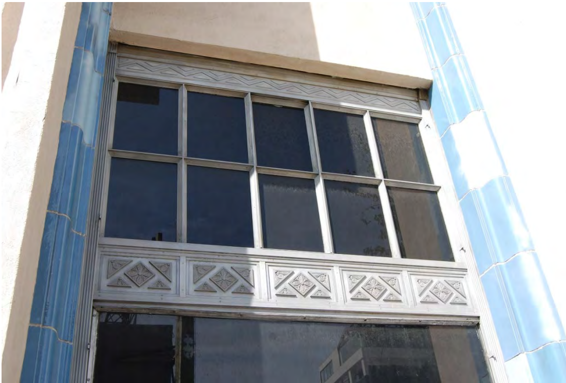
Hollywood Citizen-News Building, 1545-1551 N. Wilcox Window detail, primary (east) façade.
