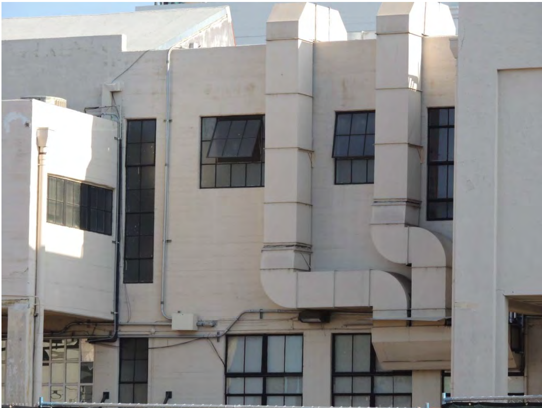
Hollywood Citizen-News Building, 1545-1551 N. Wilcox Façade detail, south façade.
