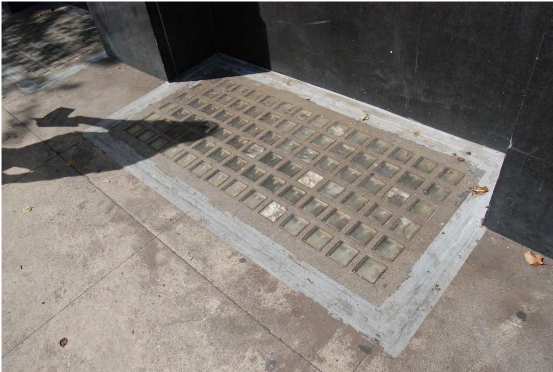
Hollywood Citizen-News Building, 1545-1551 N. Wilcox Sidewalk skylights, primary (east façade).
