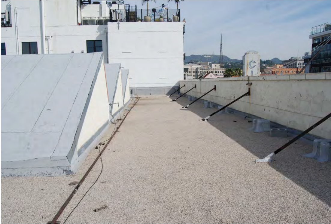
Hollywood Citizen-News Building, 1545-1551 N. Wilcox Sawtooth skylights, view looking north.
