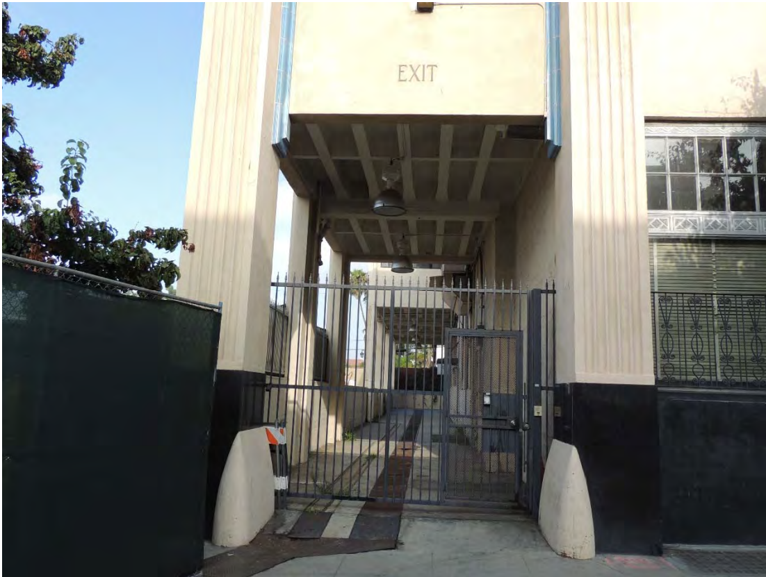
Hollywood Citizen-News Building, 1545-1551 N. Wilcox South entrance portal, primary (east) façade.
