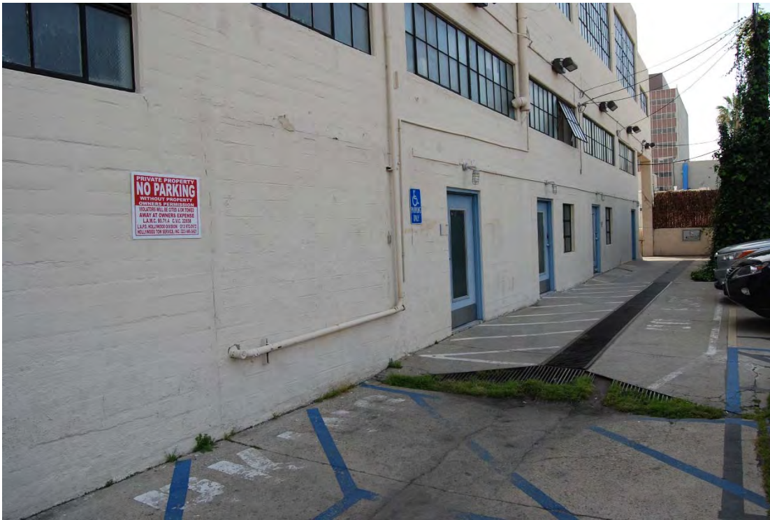
Hollywood Citizen-News Building, 1545-1551 N. Wilcox Façade detail, west façade.
