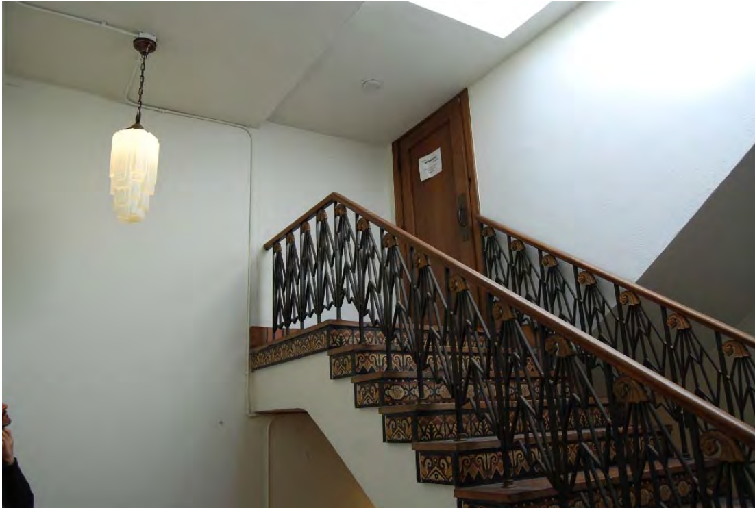
Hollywood Citizen-News Building, 1545-1551 N. Wilcox Editorial lobby (Wilcox Lobby), second floor.
