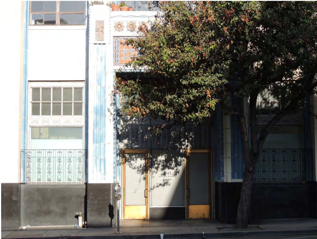
Hollywood Citizen-News Building, 1545-1551 N. Wilcox Primary entrance, primary (east) façade.
