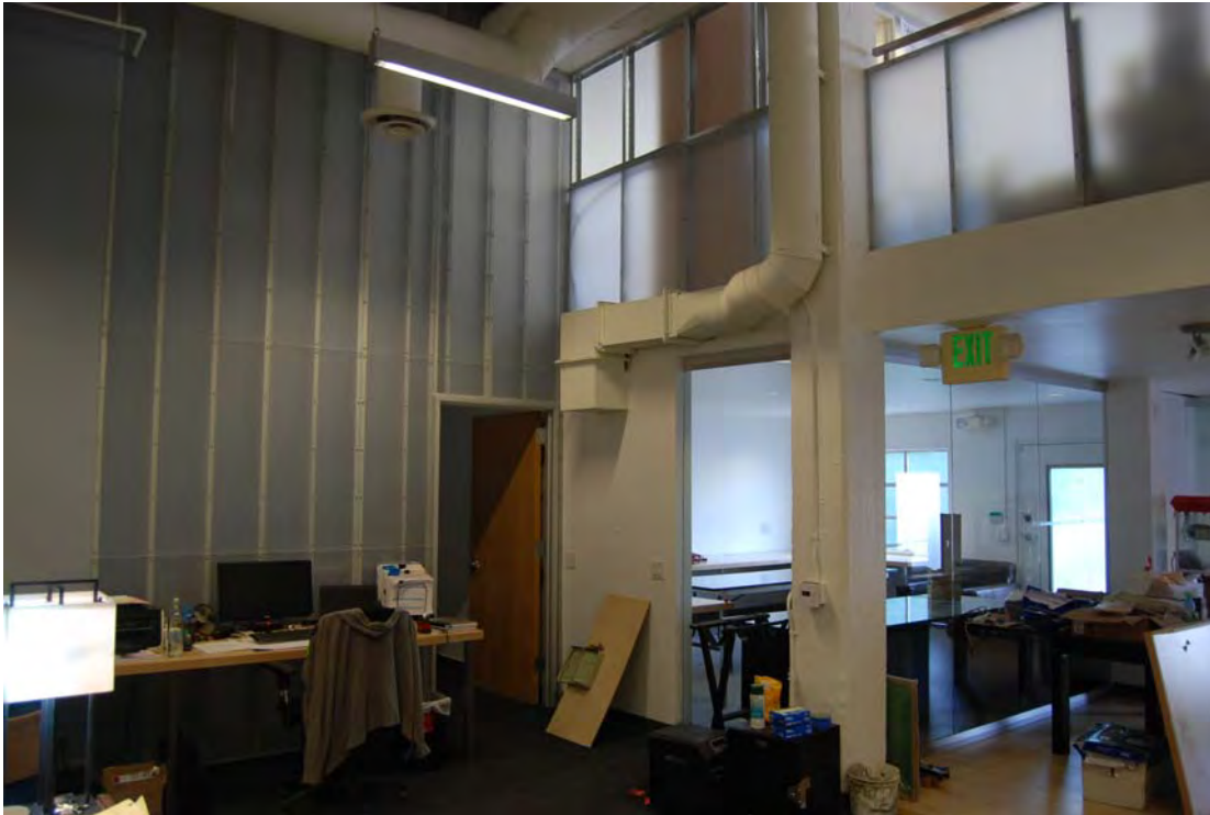
Hollywood Citizen-News Building, 1545-1551 N. Wilcox Offices, first floor.
