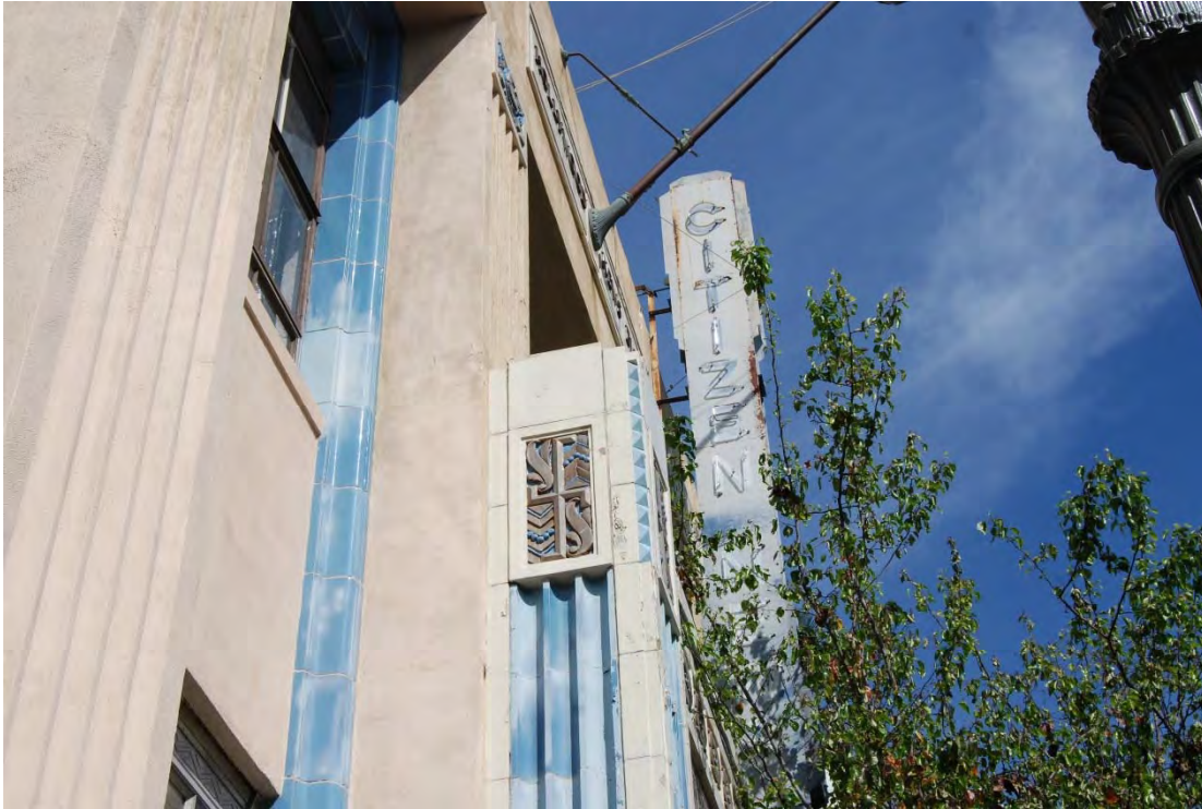
Hollywood Citizen-News Building, 1545-1551 N. Wilcox Citizen News blade sign, primary (east) façade.
