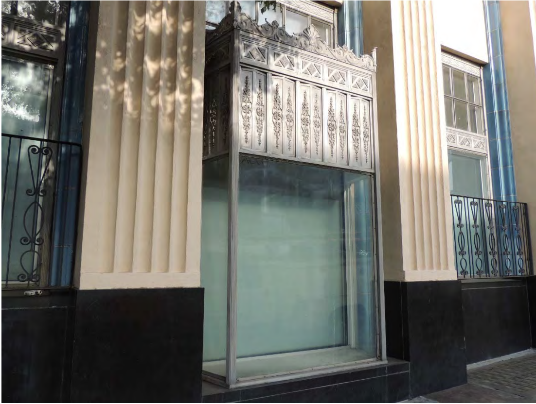
Hollywood Citizen-News Building, 1545-1551 N. Wilcox Window detail, primary (east) façade.
