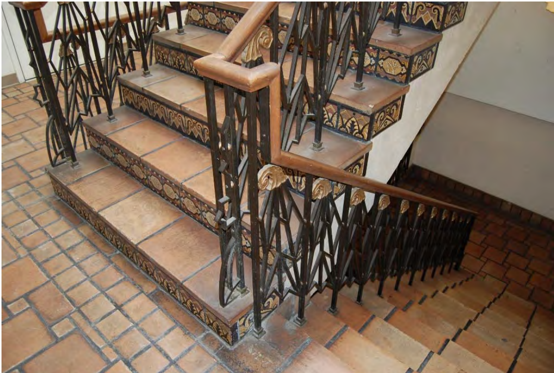
Hollywood Citizen-News Building, 1545-1551 N. Wilcox Editorial lobby (Wilcox Lobby), staircase detail.
