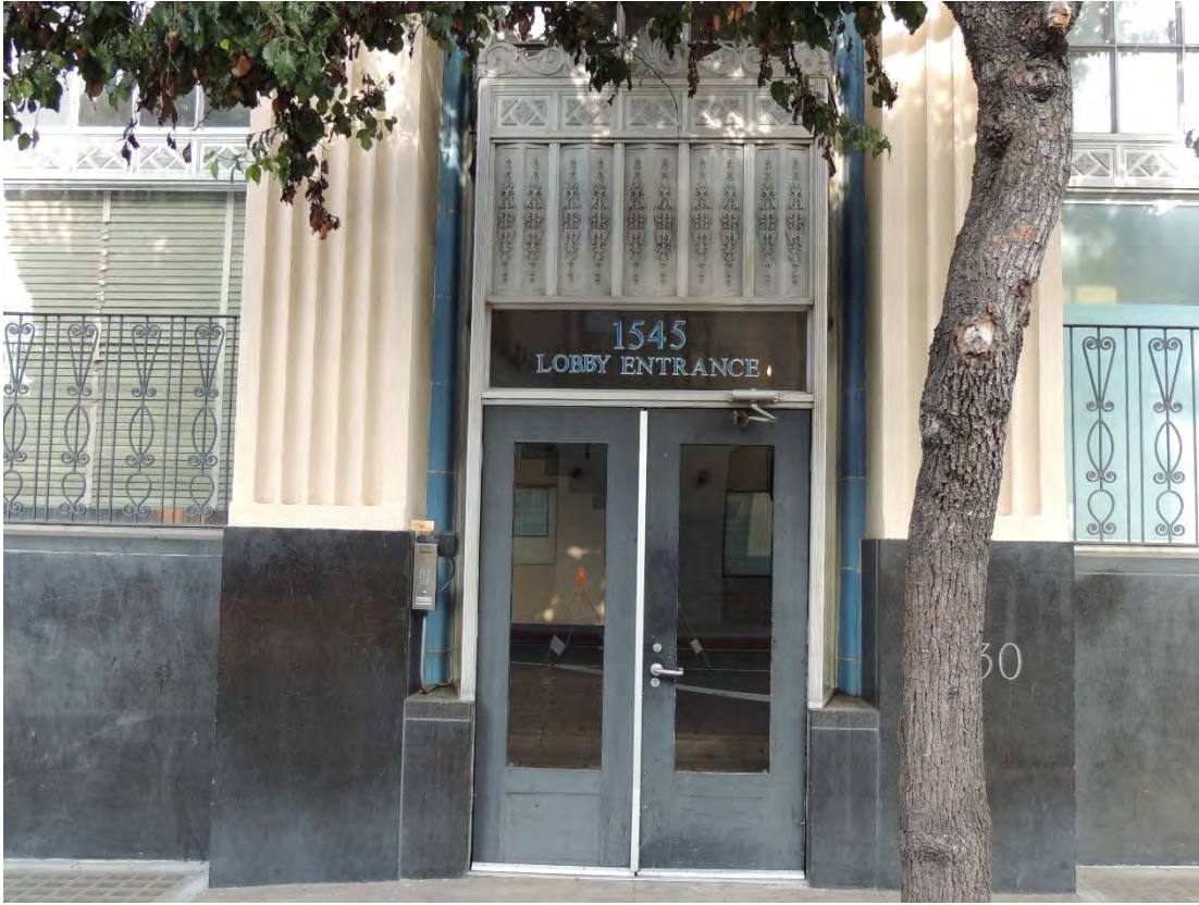
Hollywood Citizen-News Building, 1545-1551 N. Wilcox Secondary entrance, primary (east) façade.
