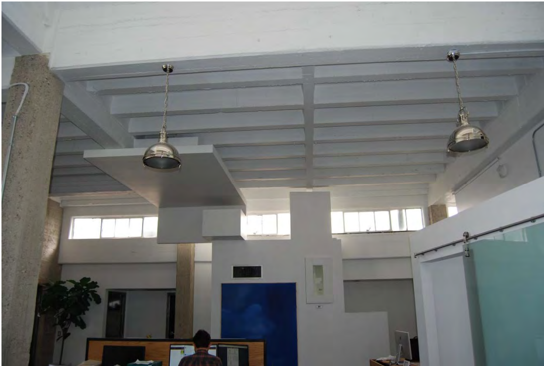
Hollywood Citizen-News Building, 1545-1551 N. Wilcox Offices, second floor.
