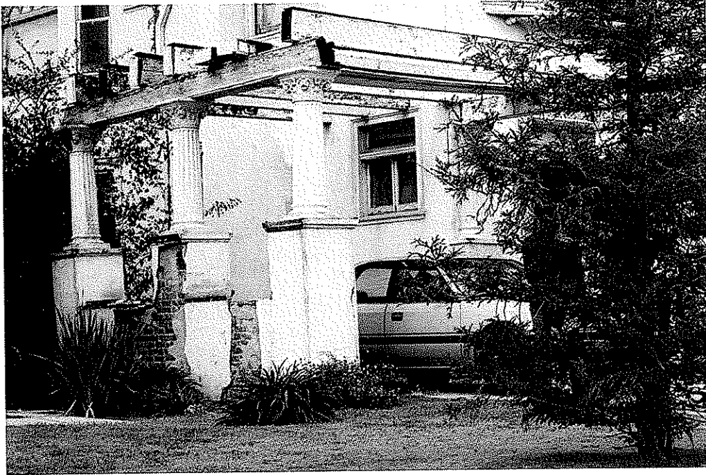
Deteriorating pergola at south elevation, viewed to northwest.
