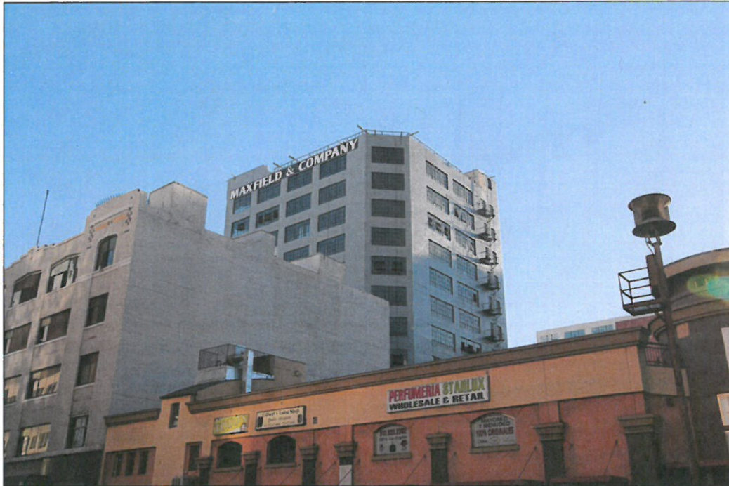
Photo 7: Maxfield Building, 819 S. Santee Street, exterior view southeast of north and west elevations, during current adaptive reuse project (Chattel, 2014)
