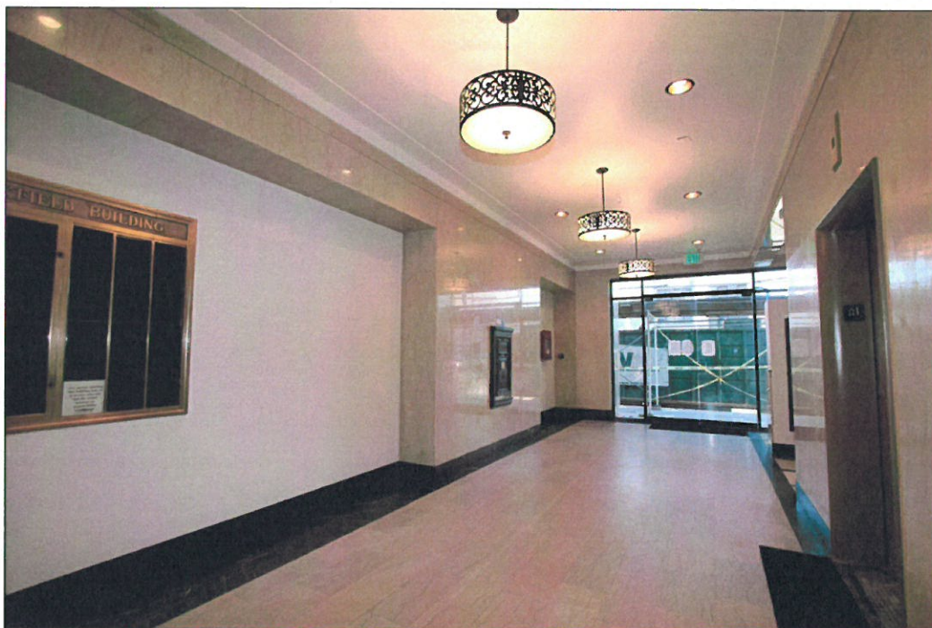
Photo 14: Maxfield Building, 819 S. Santee Street, interior view east of main lobby, during current adaptive reuse project (Chattel, 2014)
