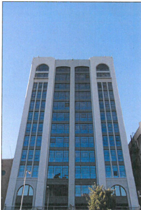
Photo 4: Maxfield Building, 819 S. Santee Street, exterior view west of east façade, during current adaptive reuse project (Chattel, 2014)
