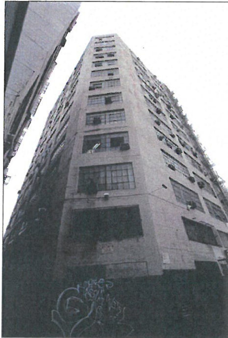
Photo 4: Maxfield Building, 819 S. Santee Street, exterior view southeast of north and west elevations (Chattel, Inc., December 4, 2012)
