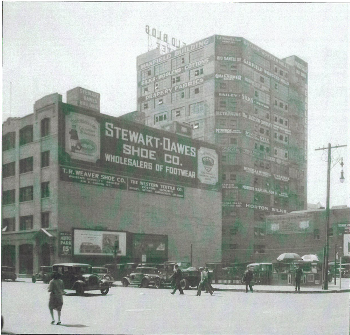
Figure 11: Maxfield Building (at center), north and west elevations, (USC Libraries Special Collections, 1931)
