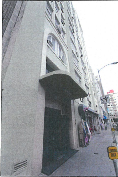
Photo 3: Maxfield Building, 819 S. Santee Street, exterior detail view northwest of east façade (Chattel, Inc., December 4, 2012)
