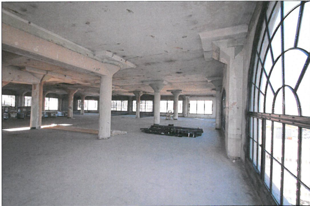
Photo 16: Maxfield Building, 819 S. Santee Street, interior view of typical upper floor open loft, during current adaptive reuse project (Chattel, 2014)
