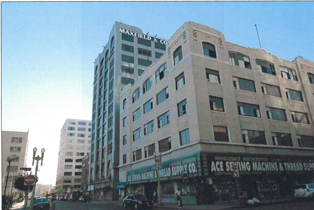
Photo 5: Maxfield Building, 819 S. Santee Street, exterior view southwest of east façade and north elevation, during current adaptive reuse project (Chattel, 2014)
