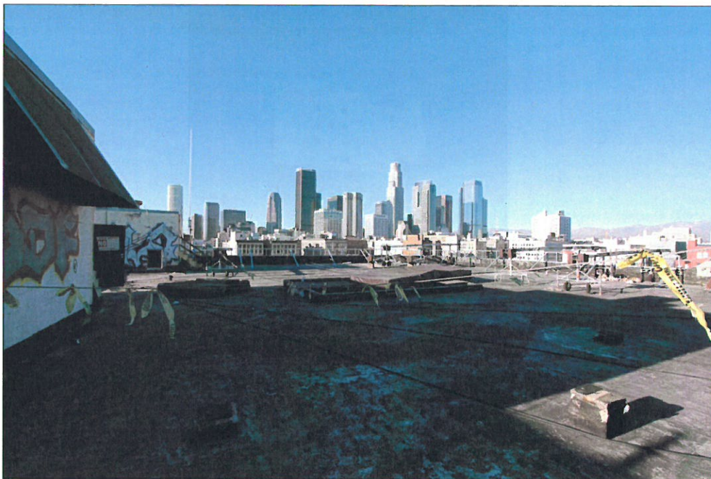
Photo 10: Maxfield Building, 819 S. Santee Street, exterior view west of roof, during current adaptive reuse project (Chattel, 2014)
