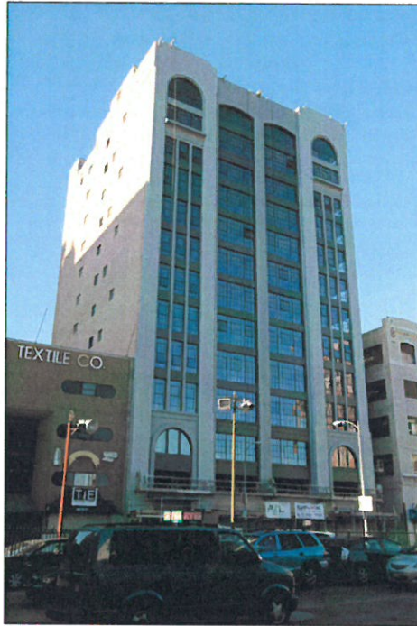
Photo 1: Maxfield Building, 819 S. Santee Street, exterior view northwest of east façade and south elevation, during current adaptive reuse project (Chattel, 2014)
