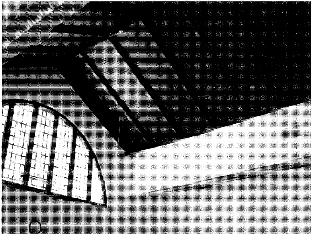
York Boulevard Church of Christ, sanctuary ceiling, 4904-08 York Boulevard, June 30, 2013
