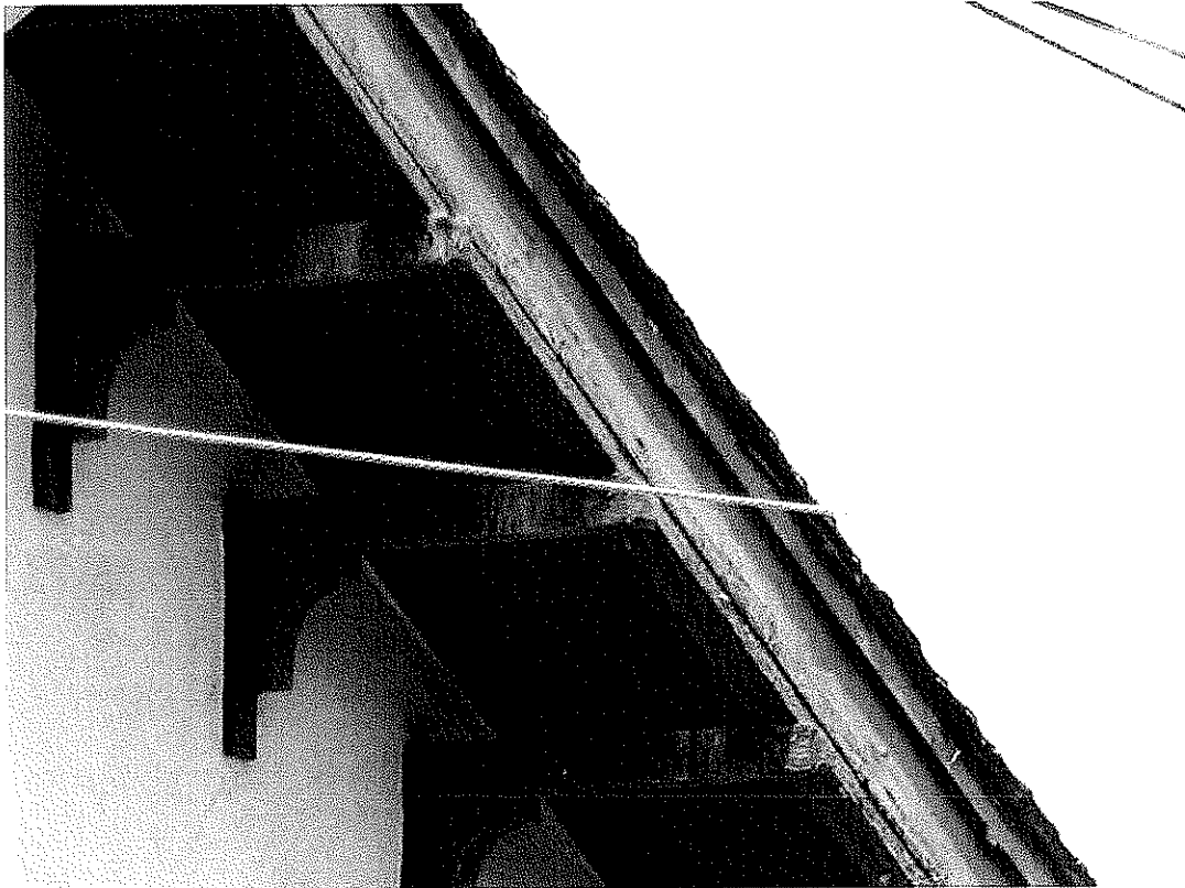
York Boulevard Church of Christ, roof brackets, December 5, 2013
