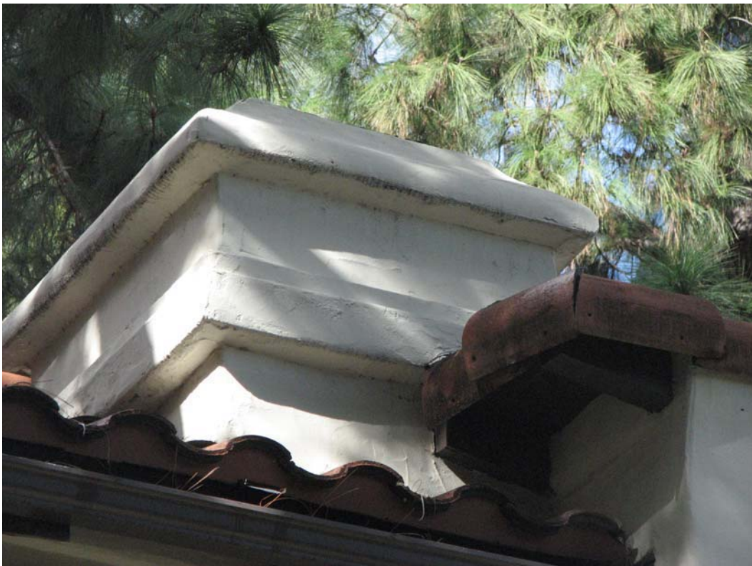
Clarence G. Badger Residence, chimney, 7128 Woodrow Wilson Drive, January 28, 2008 (Charles J. Fisher photo)
