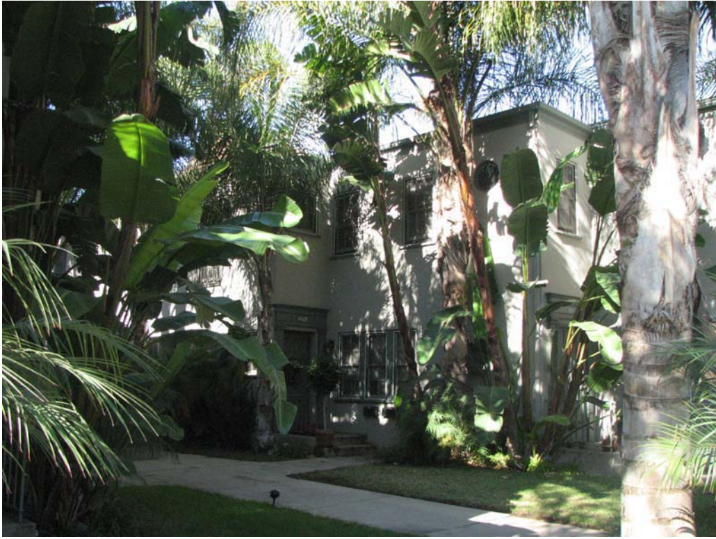
Glen View Garden Apartments, 1801-17 N. New Hampshire Avenue, December 27, 2007 (Charles J. Fisher photo)
