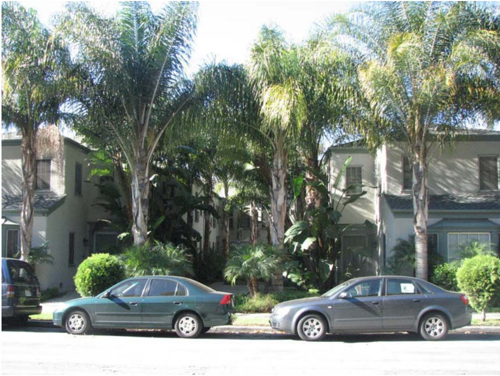
Glen View Garden Apartments, 1801-17 N. New Hampshire Avenue, December 27, 2007 (Charles J. Fisher photo)
