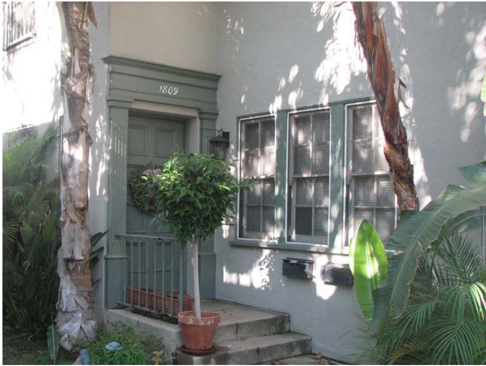
Glen View Garden Apartments, 1801-17 N. New Hampshire Avenue, December 27, 2007 (Charles J. Fisher photo)
