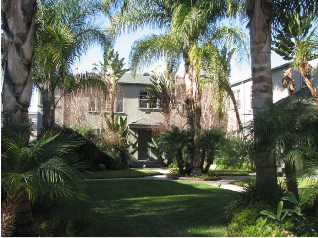
Glen View Garden Apartments, 1801-17 N. New Hampshire Avenue, December 27, 2007 (Charles J. Fisher photo)
