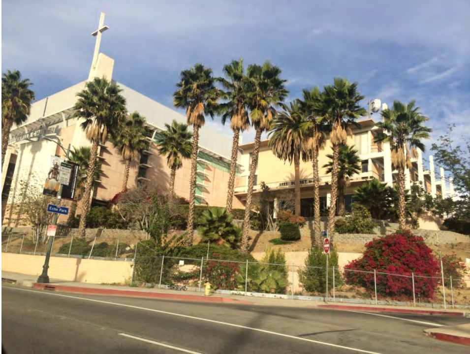
44. Metropolitan Water District Headquarters Campus, Sanctuary Addition, south and east elevations
