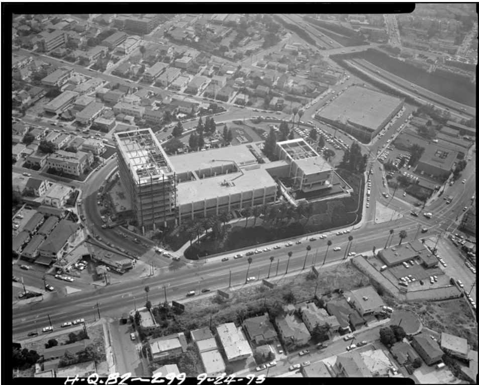
62. Aerial view looking northeast with garage, 1975
