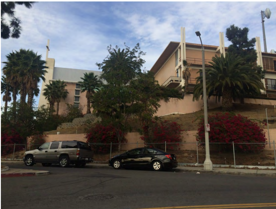
25. Metropolitan Water District Headquarters Campus, Original Beaudry Building south and east elevations
