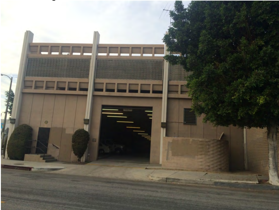
47. Metropolitan Water District Headquarters Parking Structure at Beaudry Street and Figueroa Terrace
