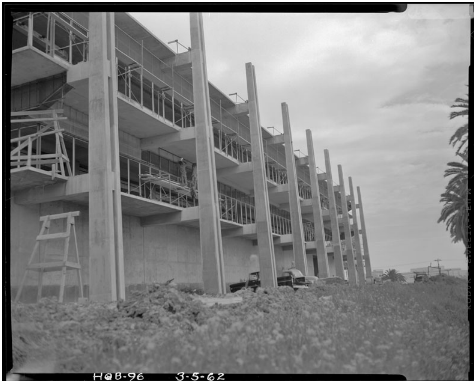
6. Metropolitan Water District Headquarters Campus under construction, Original Building Sunset wing, c. 1962
