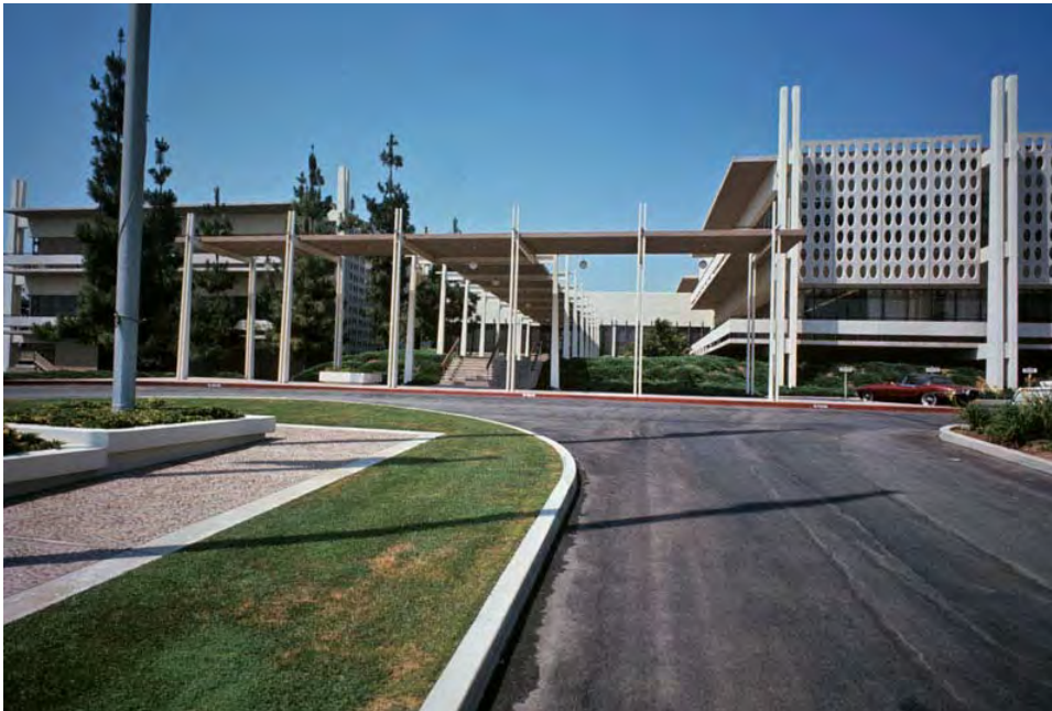
20. Metropolitan Water District Headquarters Campus, main entrance with entry pergola, Alpine Street, looking west, c1970s
