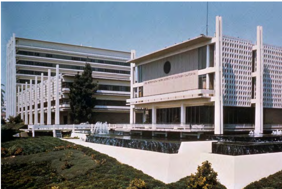
18. Metropolitan Water District Headquarters Campus, Original Beaudry Building, Original Building Sunset wing, High Rise Building, south and east elevations, c.1974
