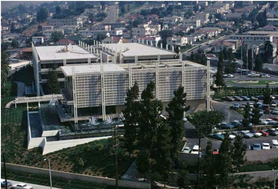
11. Metropolitan Water District Headquarters Campus, Original Beaudry Building and Original Building Sunset wing, looking east, c. 1962
