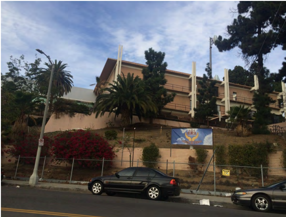
24. Metropolitan Water District Headquarters Campus, Sanctuary Addition, south elevation and Original Beaudry Building south and east elevations
