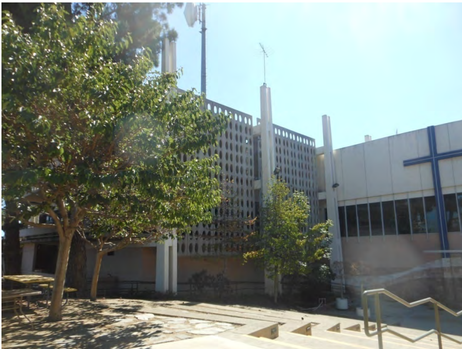
31. Metropolitan Water District Headquarters Campus, Original Beaudry Building, west elevation and Sanctuary Addition, north elevation
