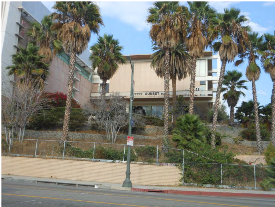
23. Metropolitan Water District Headquarters Campus, Beaudry Building, south elevation and Sanctuary east elevation.
