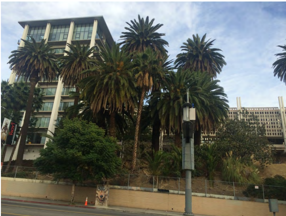
39. Metropolitan Water District Headquarters Campus, High Rise Building, south elevation
