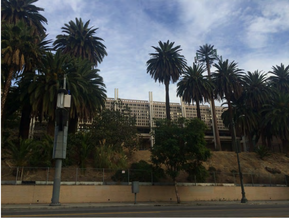
40. Metropolitan Water District Headquarters Campus, Original Sunset wing, south elevation
