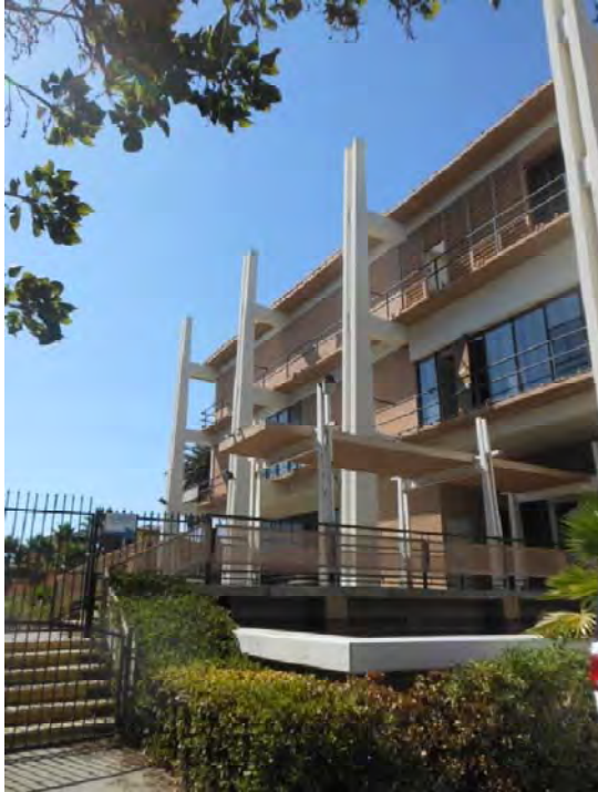
26. Metropolitan Water District Headquarters Campus, Original Beaudry Building east elevation
