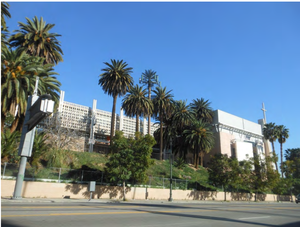
41. Metropolitan Water District Headquarters Campus, High Rise Building and Original Building Sunset wing, south elevations
