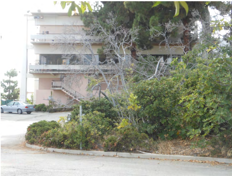
29. Metropolitan Water District Headquarters Campus, Original Beaudry Building, east elevation
