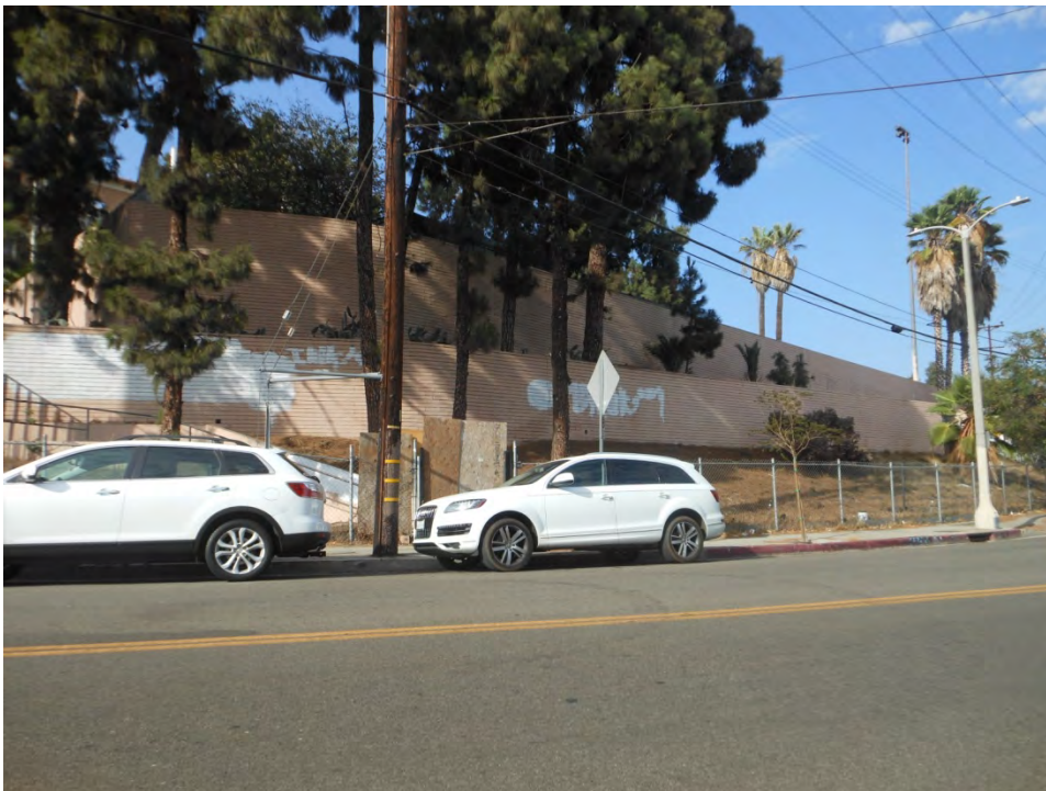
27. Retaining wall, Beaudry Avenue
