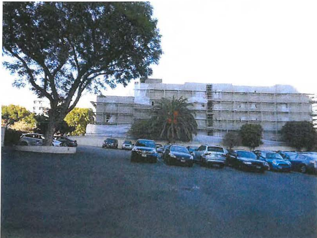
12. 7107 Hollywood Boulevard, rear parking lot looking south.
