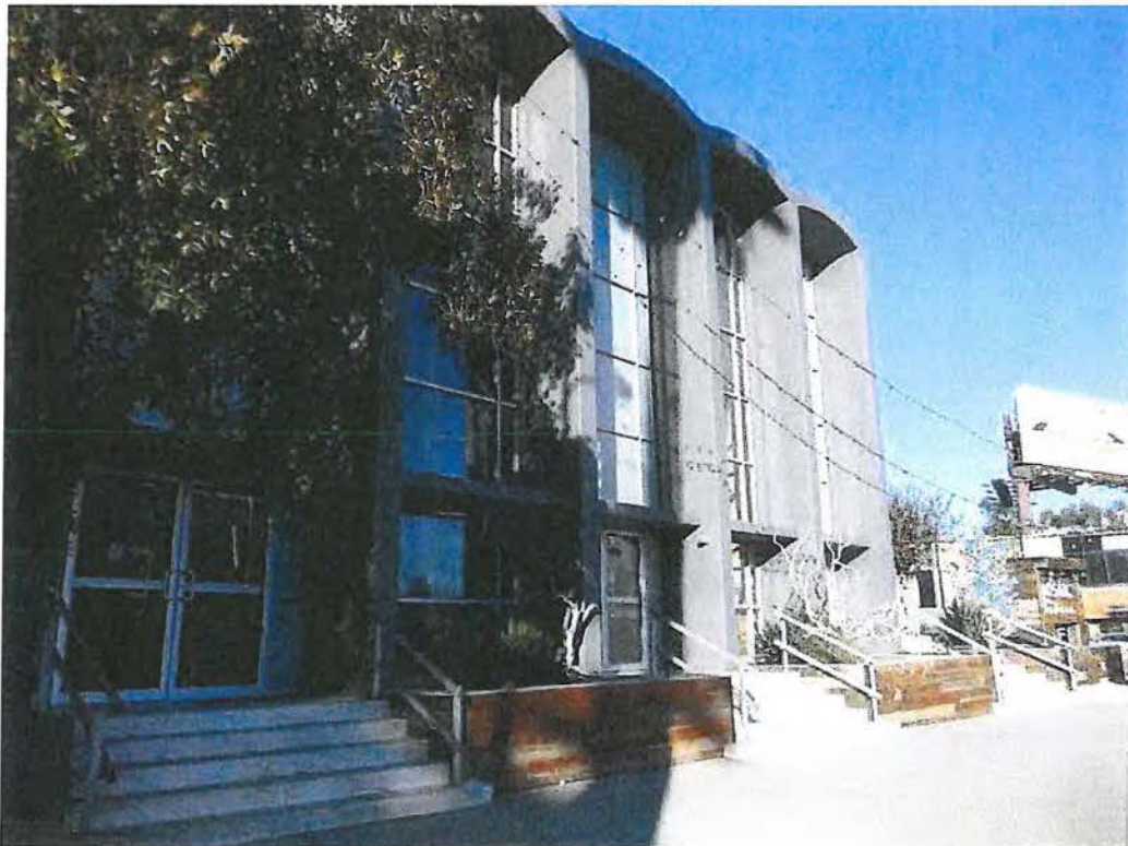
6. 7107 Hollywood Boulevard, south elevation.
