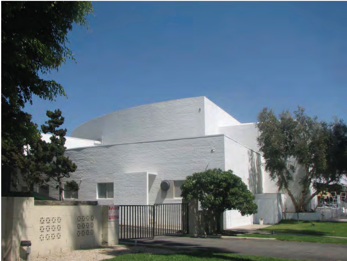
Fifth Church of Christ Scientist, West facade, 7107 Hollywood Boulevard, April 6, 2015 (Photograph by Charles J. Fisher)
