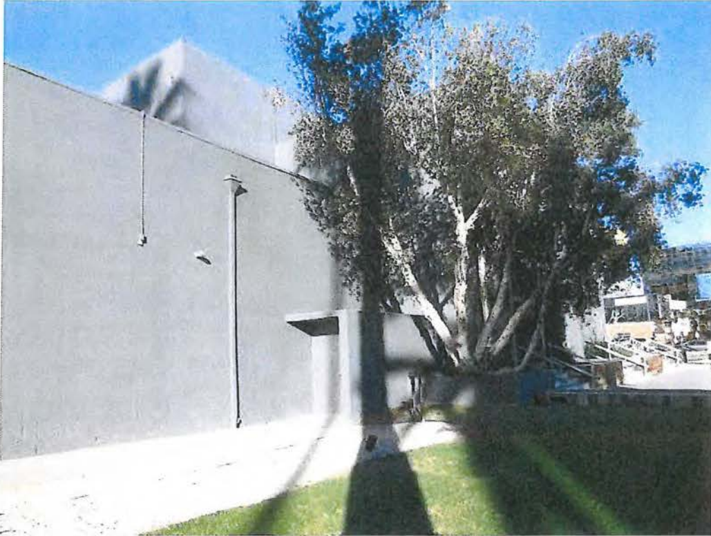
7. 7107 Hollywood Boulevard, west end of south elevation.
