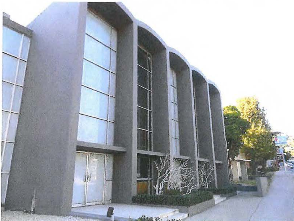
18. 7107 Hollywood Boulevard, east entrance.
