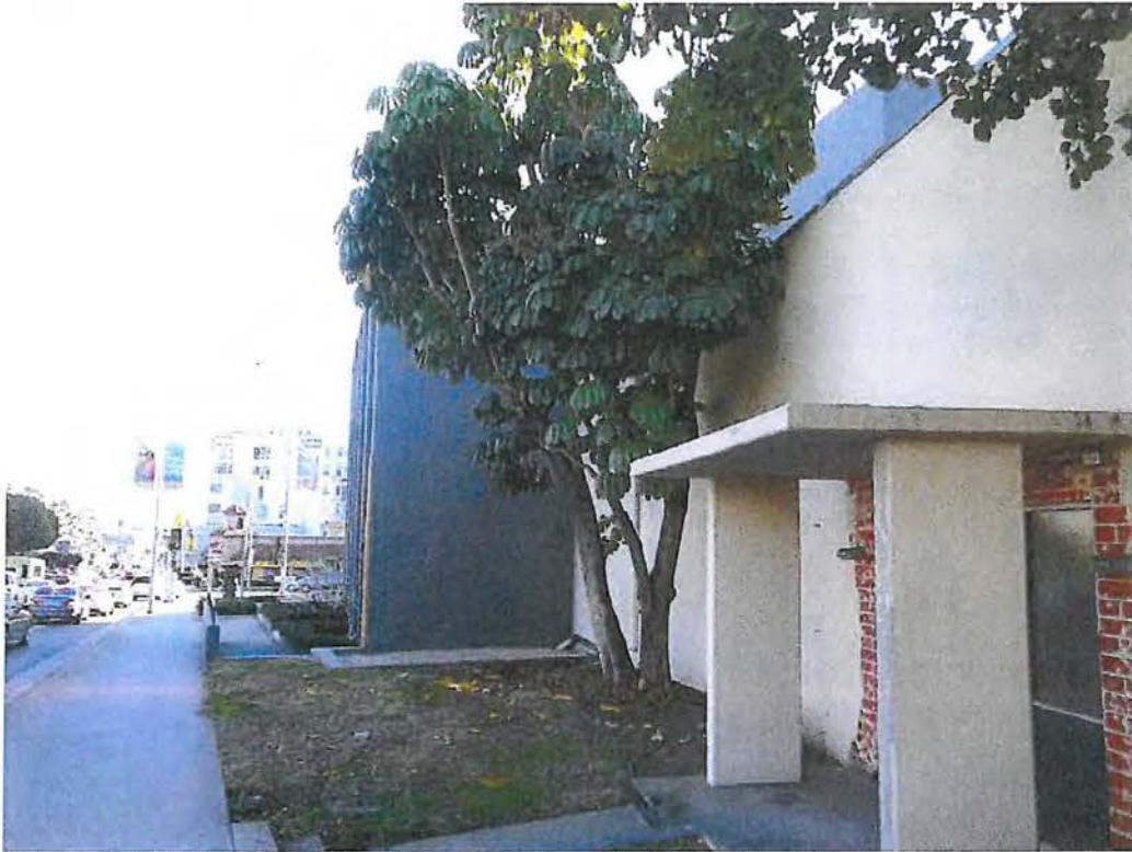
17. 7107 Hollywood Boulevard, north end of east elevation.
