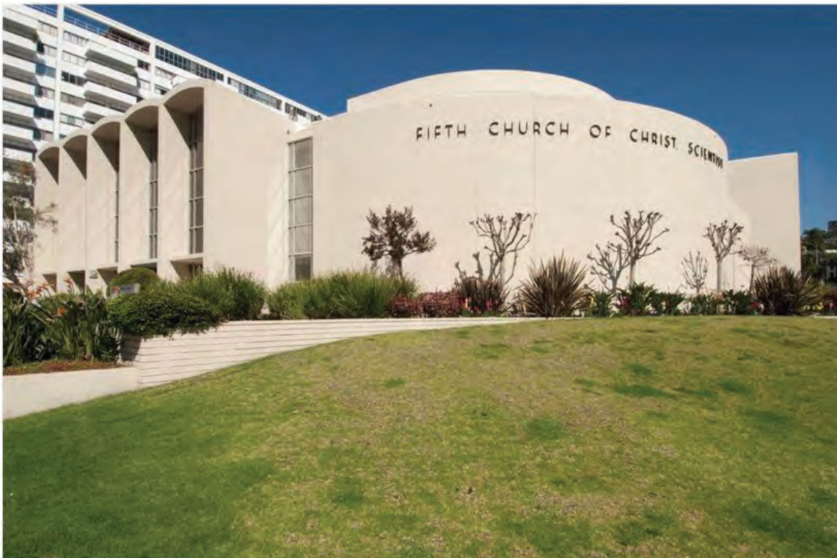
Fifth Church of Christ Scientist before sale, 7107 Hollywood Boulevard, April 2011 (Photograph by Larry Underhill)
