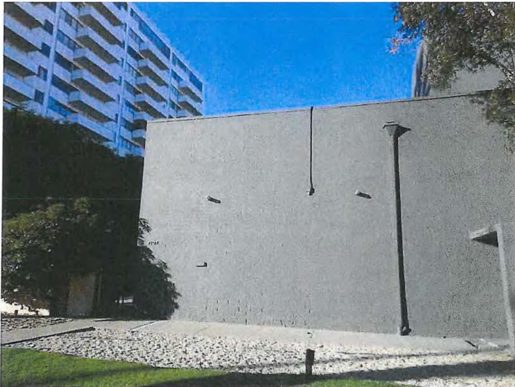
8. 7107 Hollywood Boulevard, west end of south elevation.
