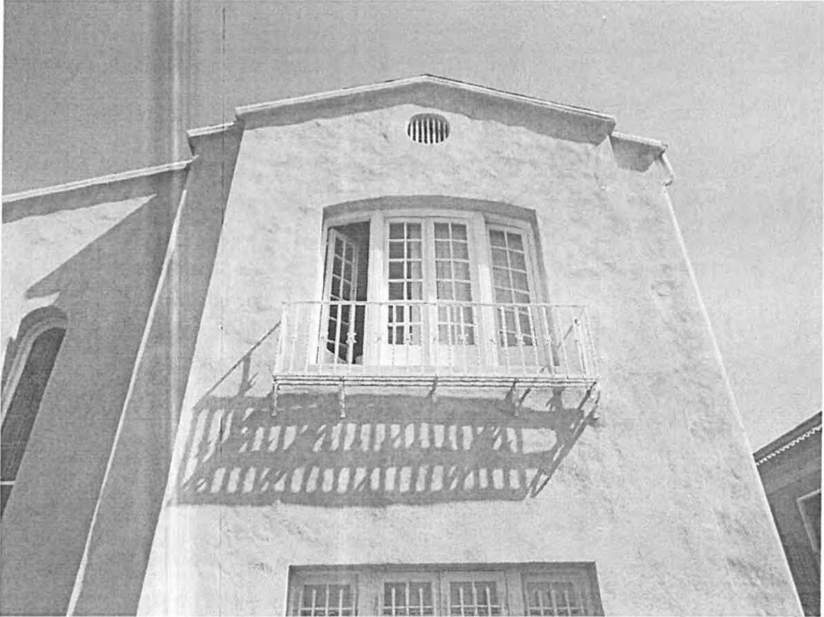
674 Crenshaw, west left front façade, second floor, camera facing east
