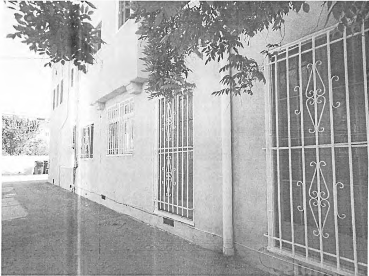
674 Crenshaw, north left side façade, second floor, camera facing southeast
