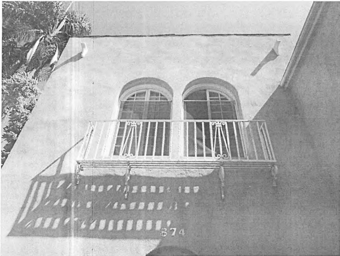
674 Crenshaw, second floor west façade left, camera facing east
