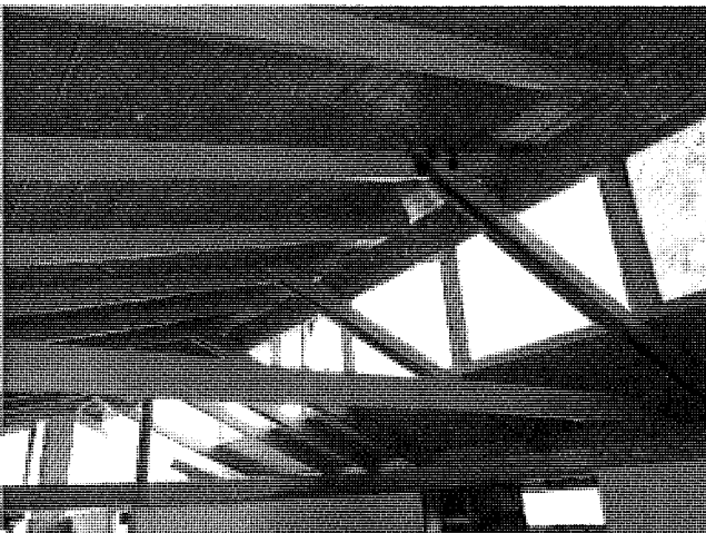
Vaulted ceiling in living room.
