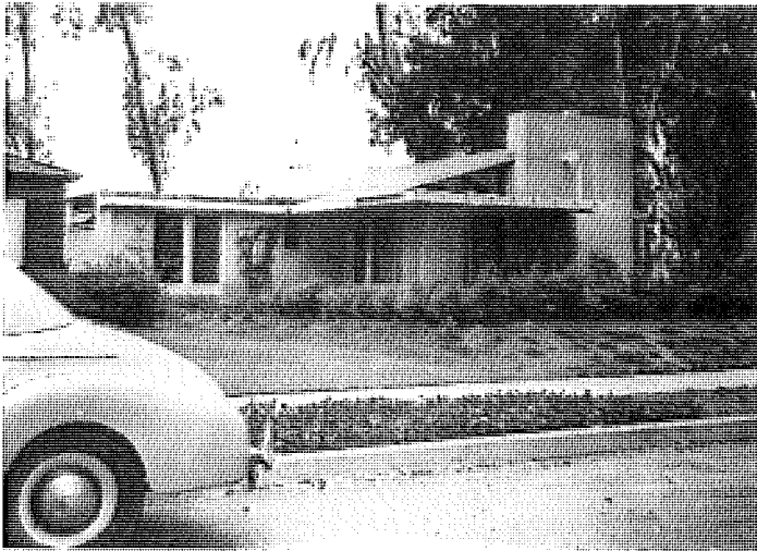
Photo of newly built Presburger House circa 1947. Original doors and windows are visible. Photo courtesy of the Presburger Family Archives
