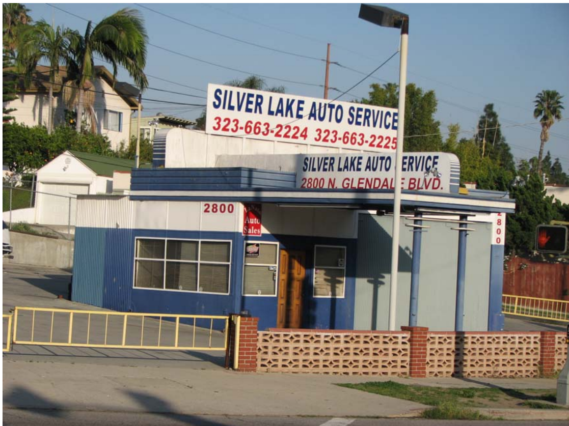
Richfield Service Station in present condition, 2800 Glendale Boulevard, Mar 14, 2008 (Charles J. Fisher photo)
