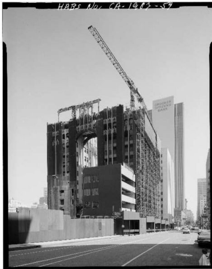
Richfield Tower, demolition photo, April 1969
