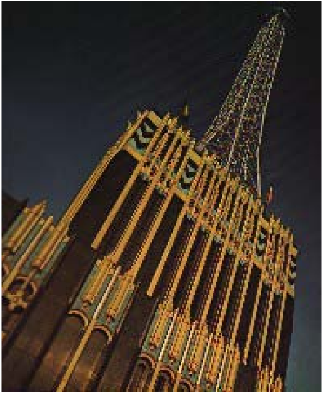
Richfield Tower showing various terra cotta colors and gold leaf trim
