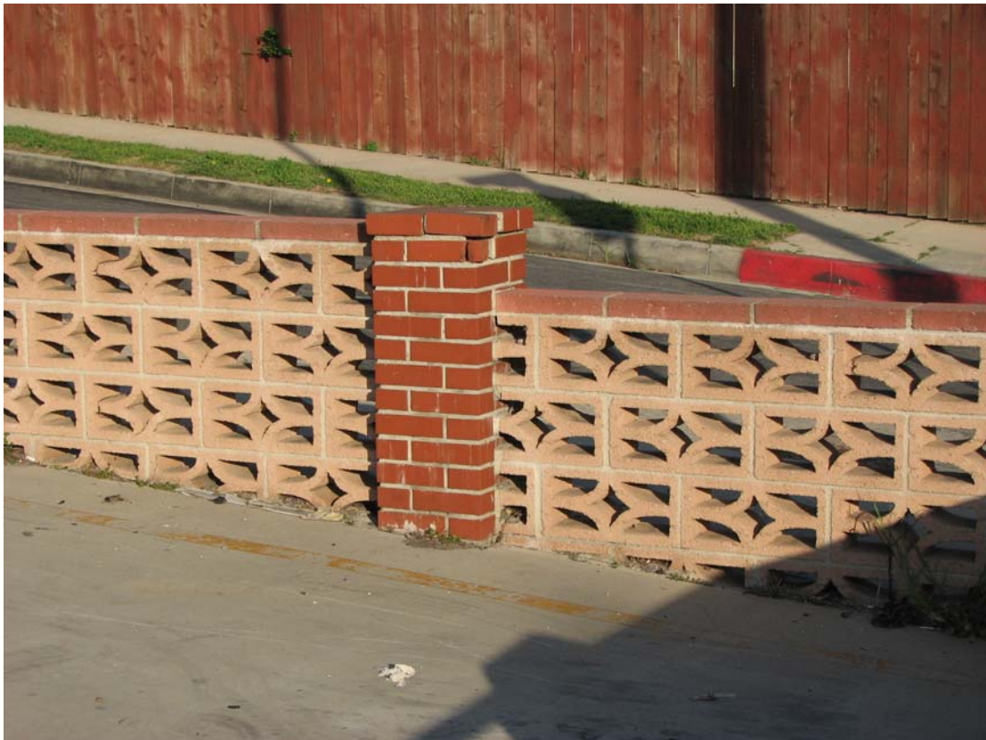
Richfield Service Station, perimeter wall on property, 2800 Glendale Boulevard, Mar 14, 2008 (Charles J. Fisher photo)
