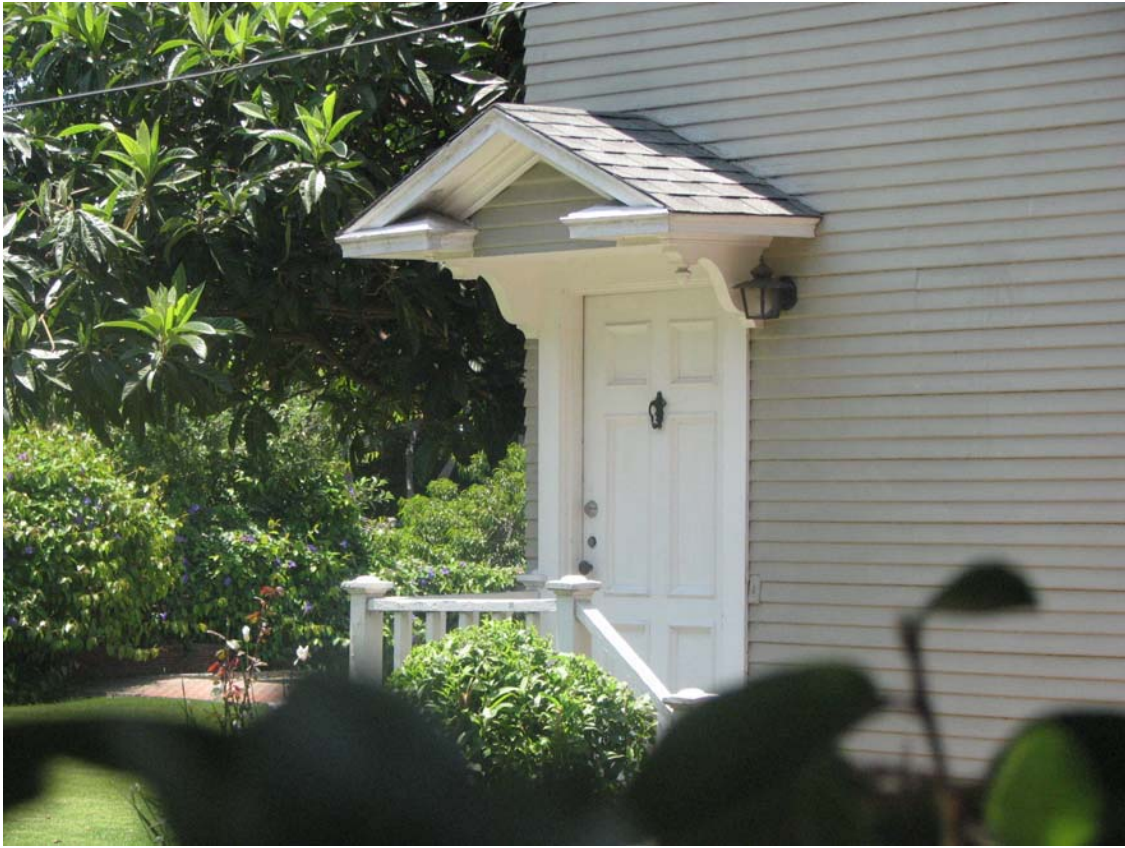
Heerman Estate, utility room entry, carriage barn, 525 S Van Ness Avenue (Photograph by Charles J. Fisher)
