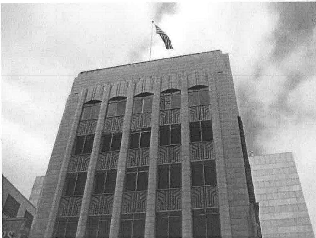
F & W Grand Silver Building, 537-41 S. Broadway, July 23, 2015 (Photograph by Charles J. Fisher)
