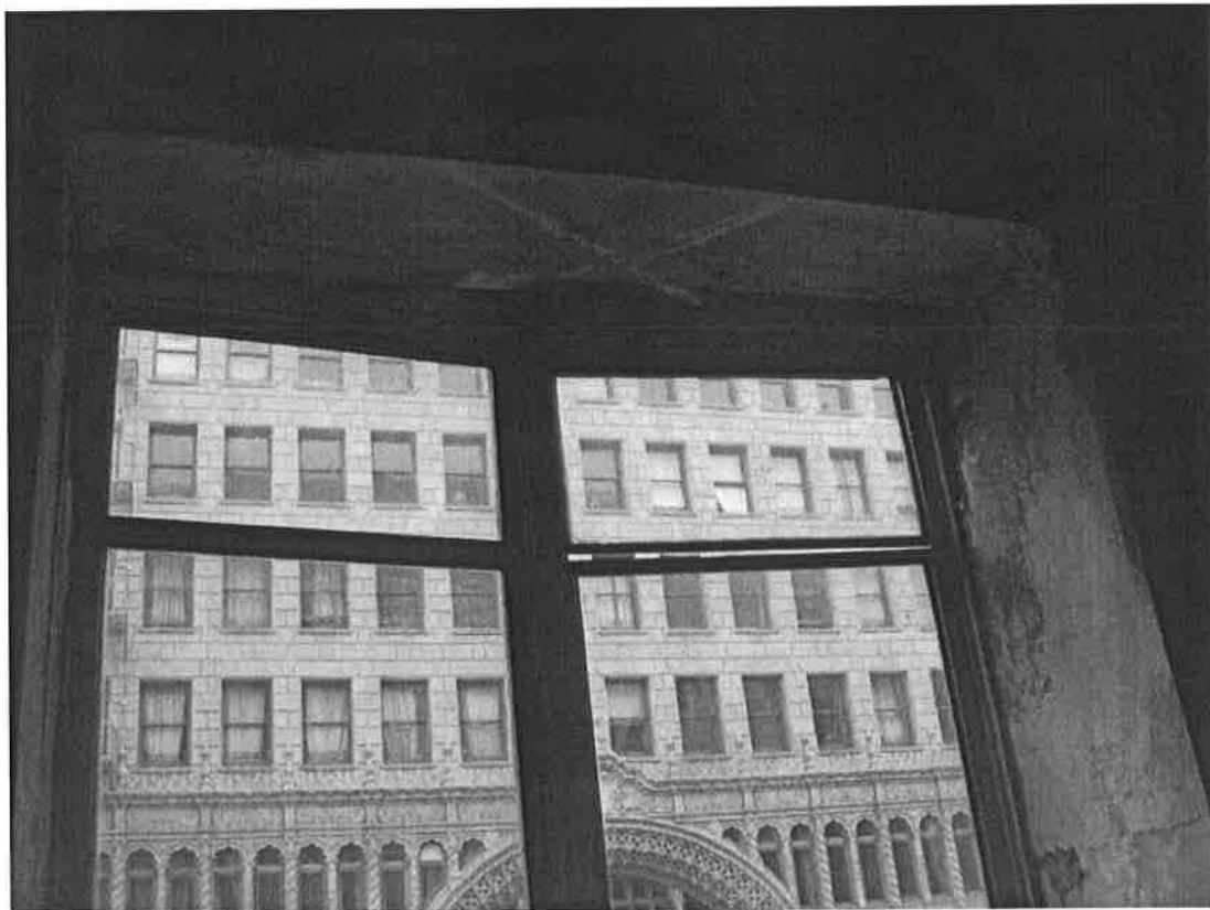
F & W Grand Silver Building, interior of window, 537-41 S. Broadway, July 23, 2015 (Photograph by Charles J. Fisher)
