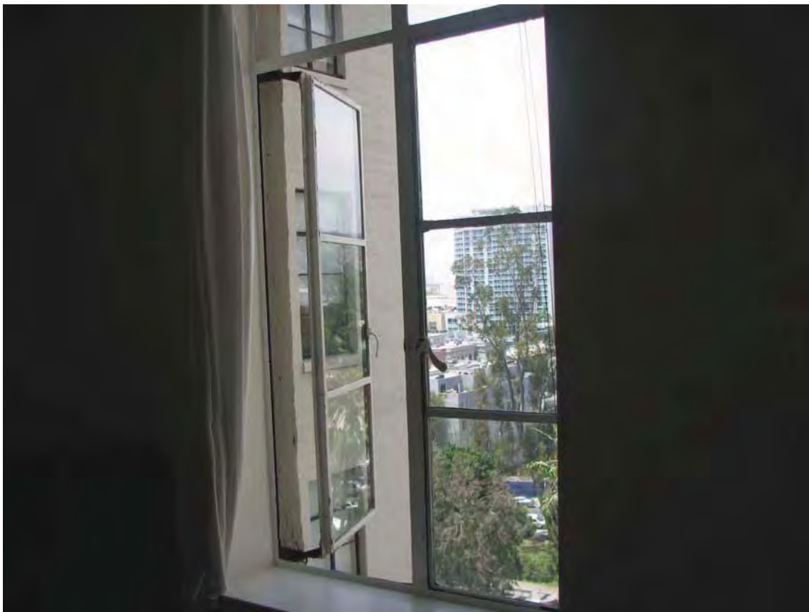
Montecito, typical steel casement window, 6650 W Franklin Avenue, May 29, 2017 (Photograph by Charles J. Fisher)
