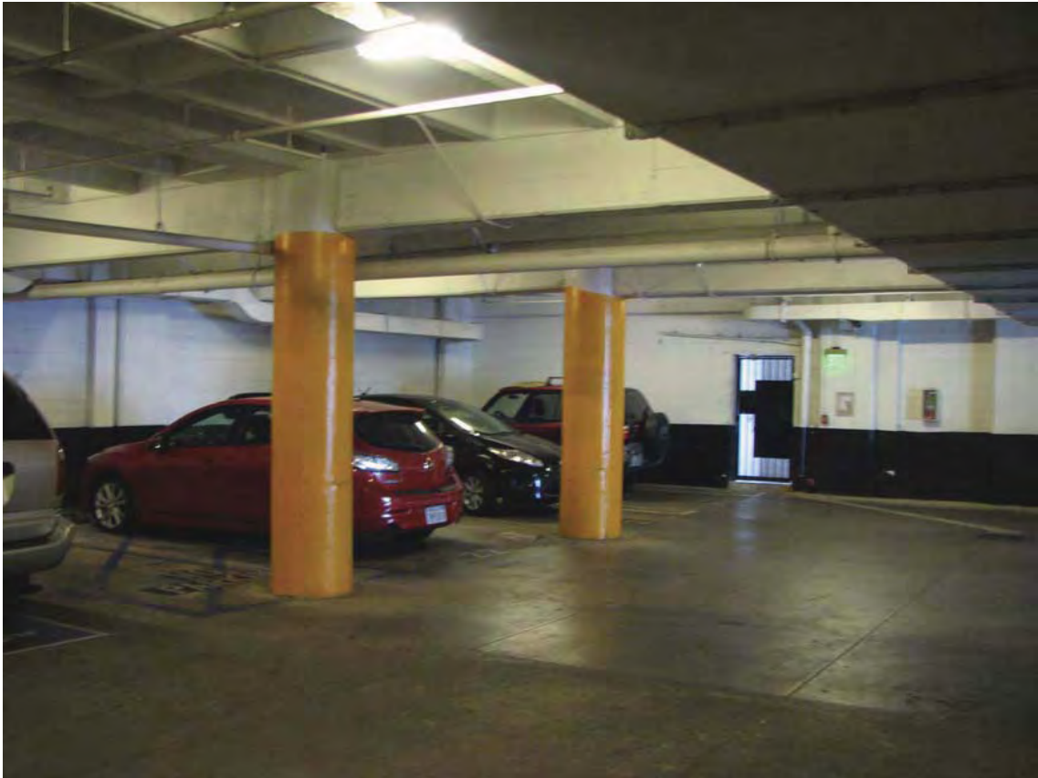
Montecito, basement garage, 6650 W Franklin Avenue, May 29, 2017 (Photograph by Charles J. Fisher)
