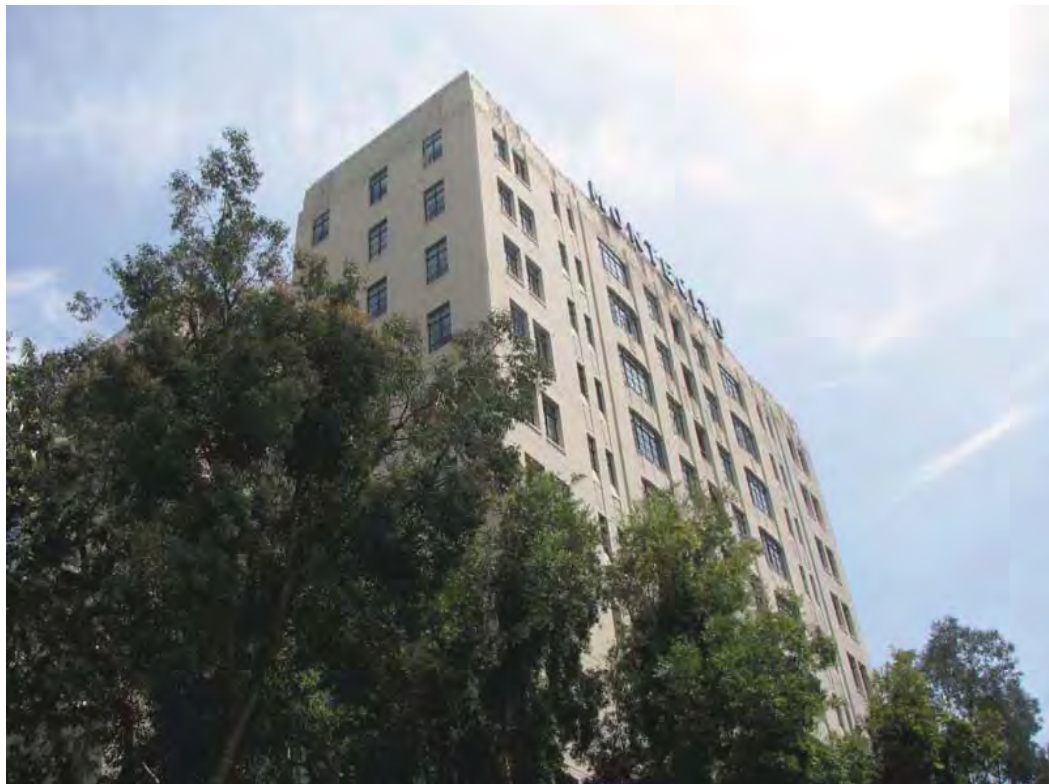
Montecito, South facade, 6650 W Franklin Avenue, May 29, 2017 (Photograph by Charles J. Fisher)
