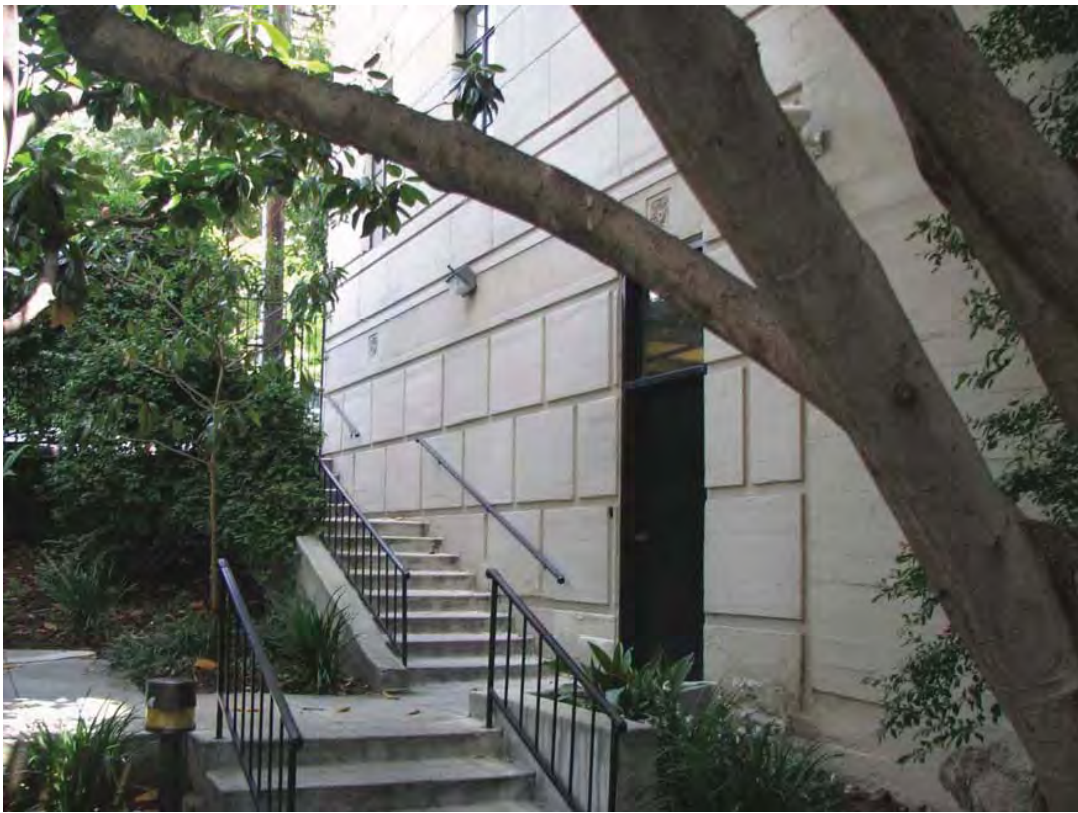
Montecito, West wall facing garden, 6650 W Franklin Avenue, May 29, 2017 (Photograph by Charles J. Fisher)
