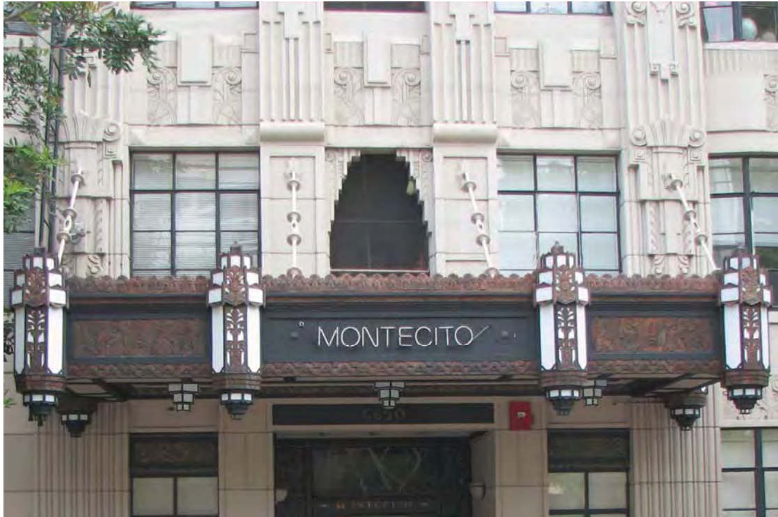
Montecito, marquee and detailing, 6650 W Franklin Avenue, May 29, 2017 (Photograph by Charles J. Fisher)
