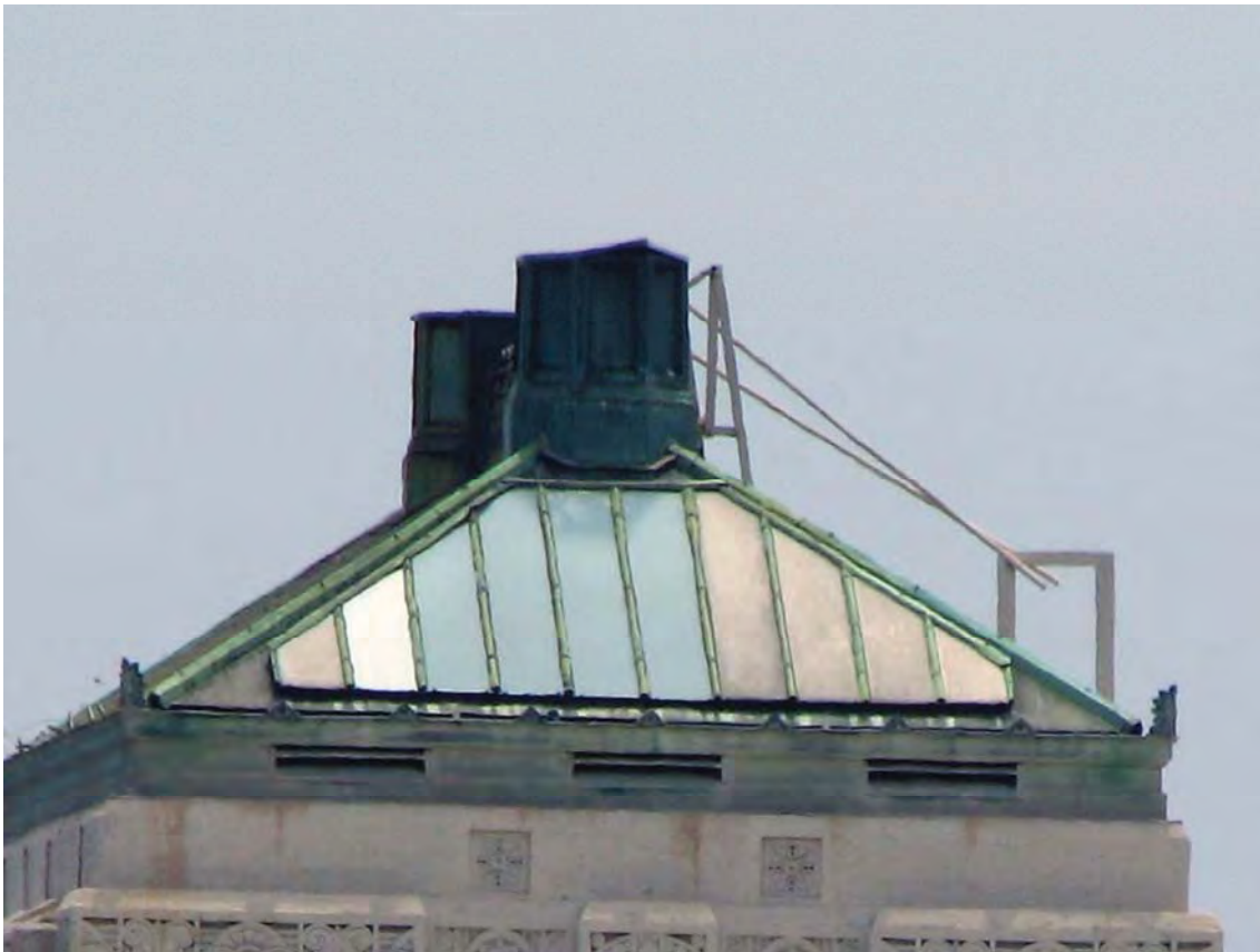
Montecito, penthouse roof, 6650 W Franklin Avenue, May 29, 2017 (Photograph by Charles J. Fisher)
