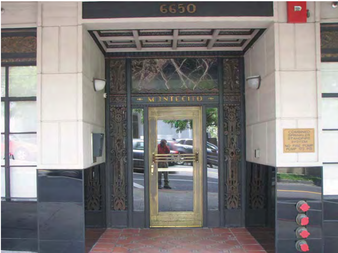
Montecito, main entrance, 6650 W Franklin Avenue, May 29, 2017 (Photograph by Charles J. Fisher)
