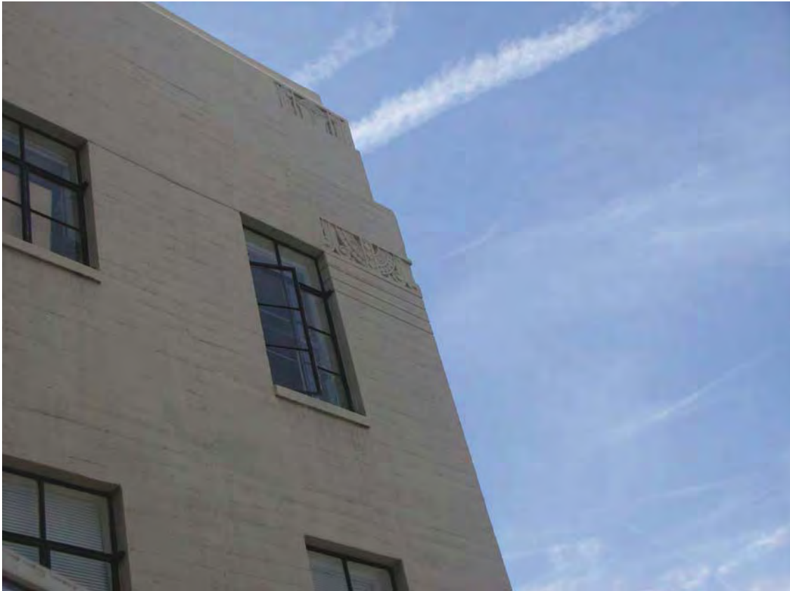
Montecito, exterior wall on West facade, 6650 W Franklin Avenue, May 29, 2017 (Photograph by Charles J. Fisher)
