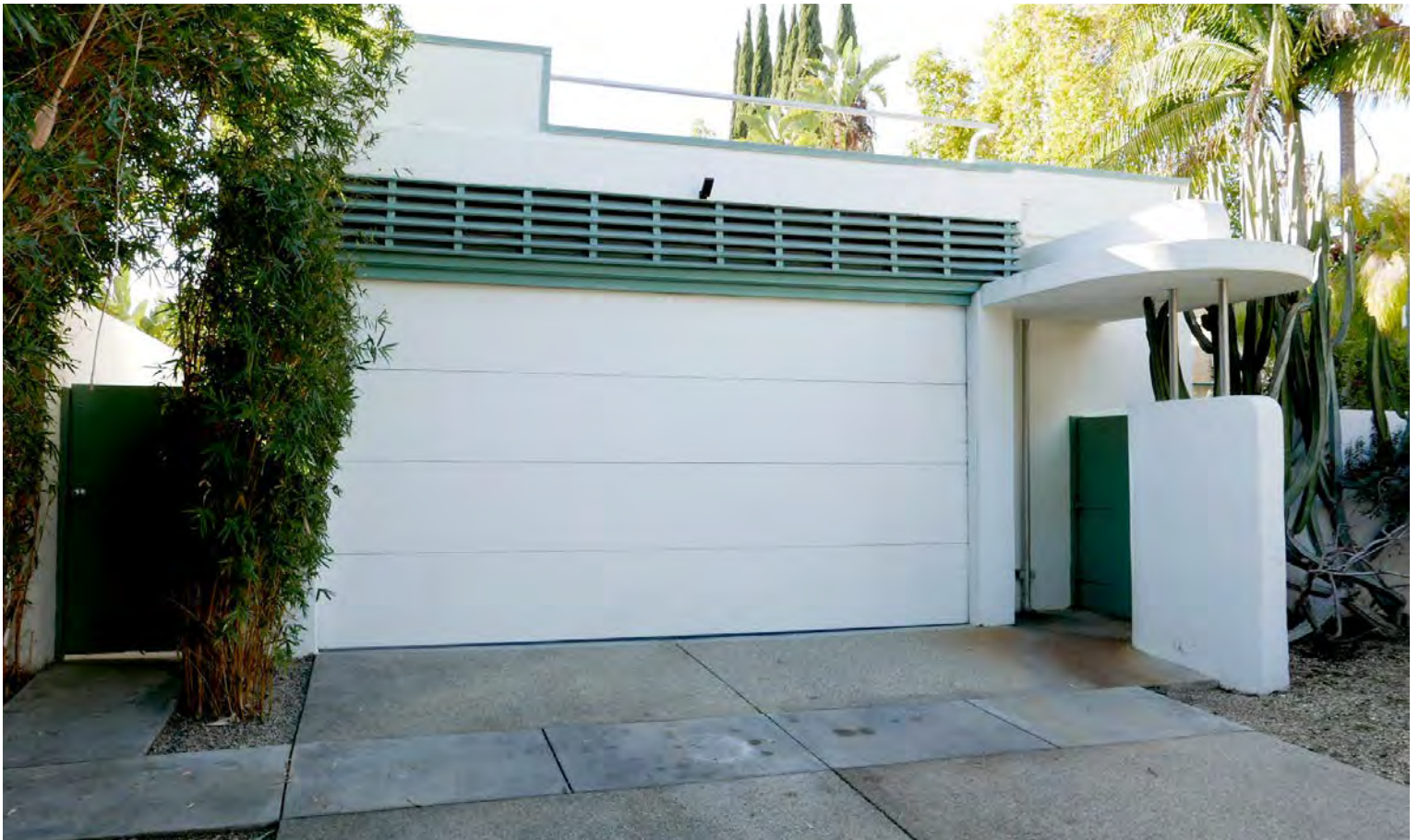
Primary (east) elevation of 947 N. Martel Ave. Garage, pergola over secondary entrance to front garden, and roof terrace with pipe railing . View west. (Luftman 2018)
