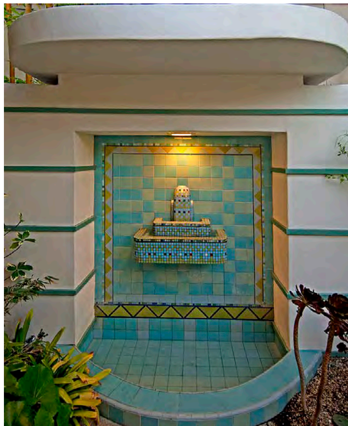
Streamline Moderne fountain detail. View north. (Everett Fenton Gidley)
