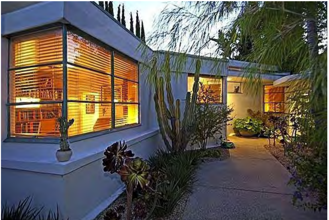
Front garden, primary entrance to 947 N. Martel Ave. North and east Façades. View west. (Everett Fenton Gidley)
