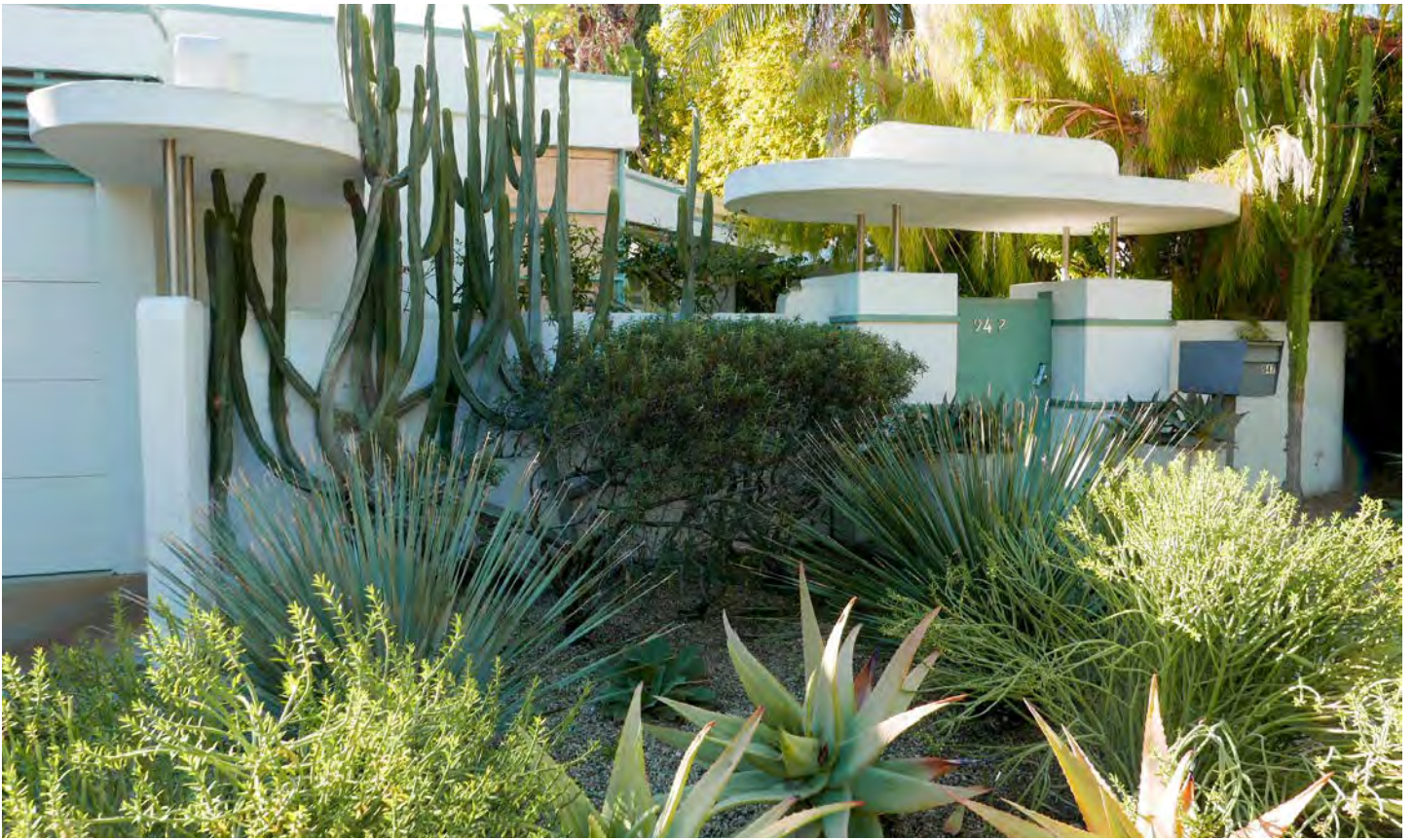
Primary (east) elevation of 947 N. Martel Ave. Pergola and garden wall details. View west. (Luftman 2018)
