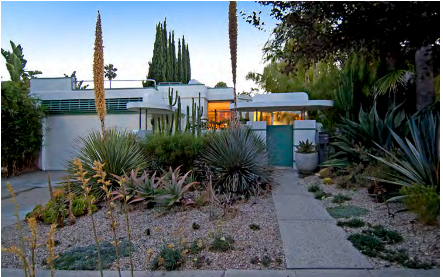
Primary (east) elevation of Wallace Beery's Hollywood Hideaway (947 N. Martel Avenue), view west. (Everett Fenton Gidley)
