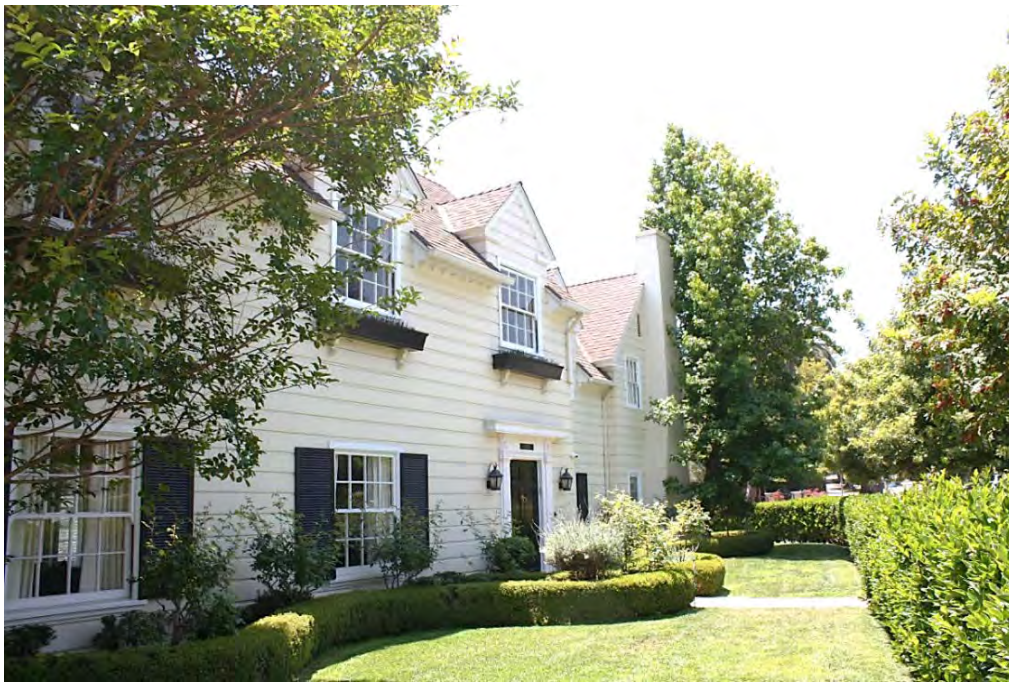
Original entrance at 5020 Ambrose Ave.: Residence/pedimented gable dormers, 8-over-8 double hung sash windows with tails, louvered shutters, window boxes/brackets second story, 6-panel door, chimney; front/north lawn, view west.
