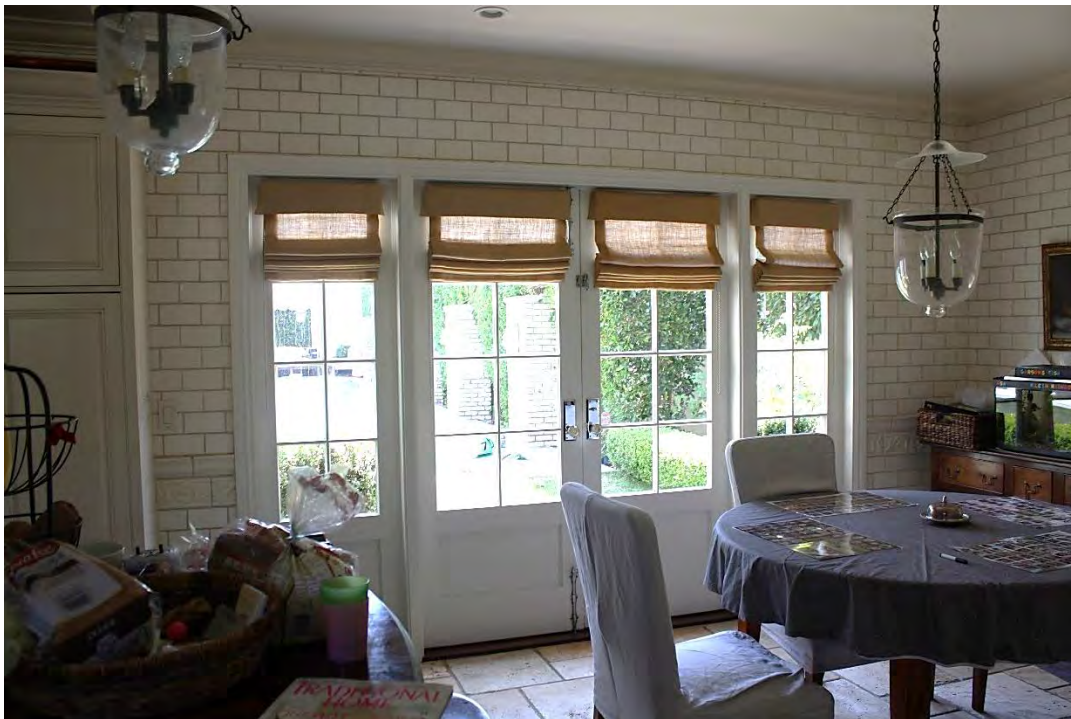
Kitchen: East doors/sidelights to pool at southeast; southeast corner, view southeast.
