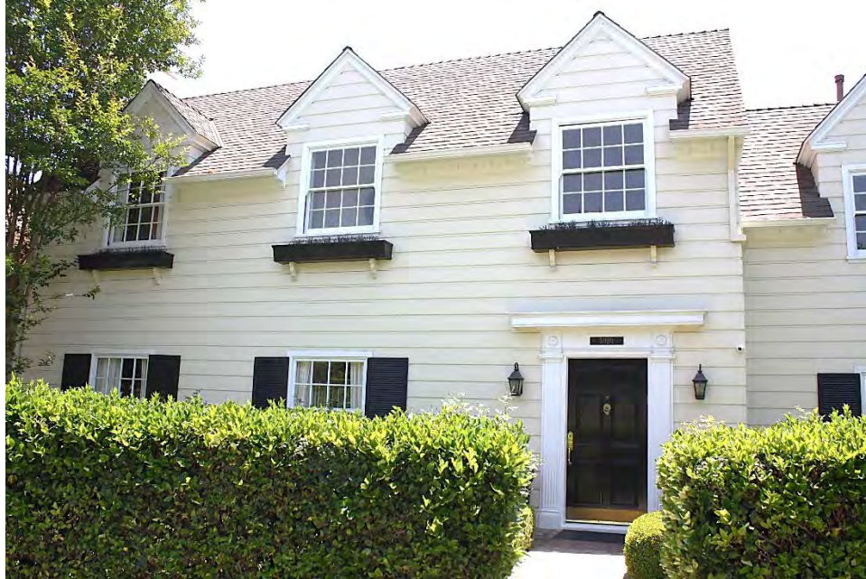
North elevation: Pedimented dormer; cornice/brackets; 8-over-8 double hung fenestration; 6-panel entry/Doric pilasters, corner posts, entablature; attached garage at east; hyphen at west, view south.
