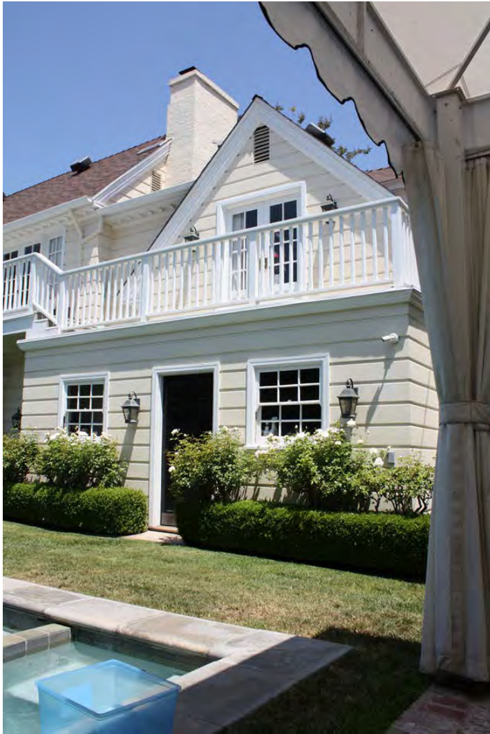
Garage, south elevation: East pedimented residence gable/chimney/vertical vents. Garage bracketed cornice. Pedimented south gable/balcony before. 6-over-6 with centered 6-panel door, view northwest.
