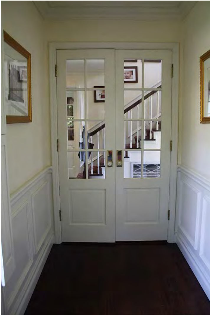
Paneled wainscoting along hall from sitting room, past dining room to Ambrose entry hall; paired, paneled 8-pane over one wood panel doors, view east.
