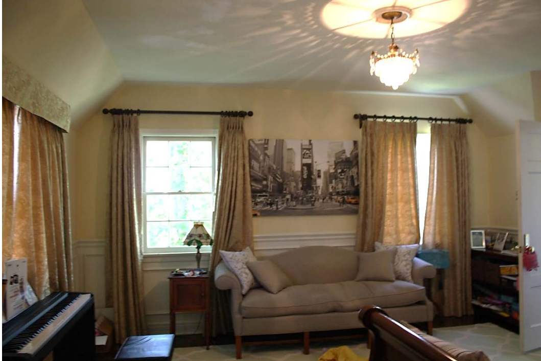
Northwest bedroom: Paneled wainscot; east 8-over-8 double hung window; south 6-over-6 double hung windows; open west entry, view south.
