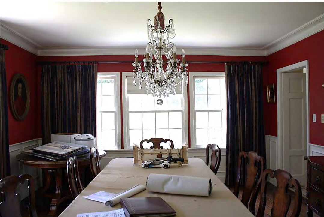
Dining room: West wall, south wall/tripartite 8-over-8 double hung fenestration; paneled wainscoting; east wall double swing 6-panel door to kitchen, view south.
