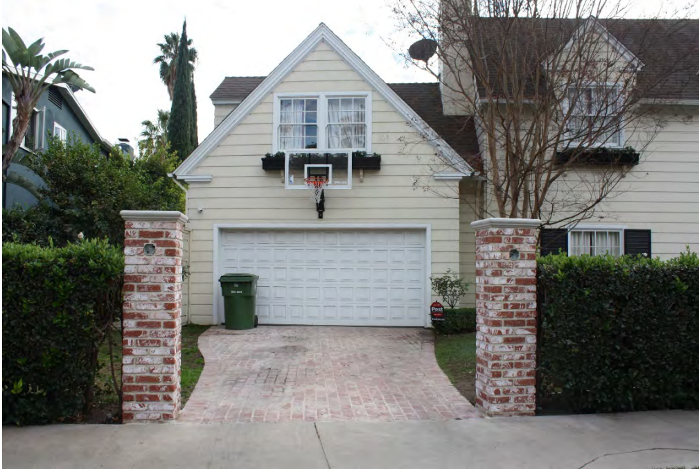
Original garage, at east end of north façade/5020 Ambrose Ave, current address; east chimney, view south. [Jan. 2018]
