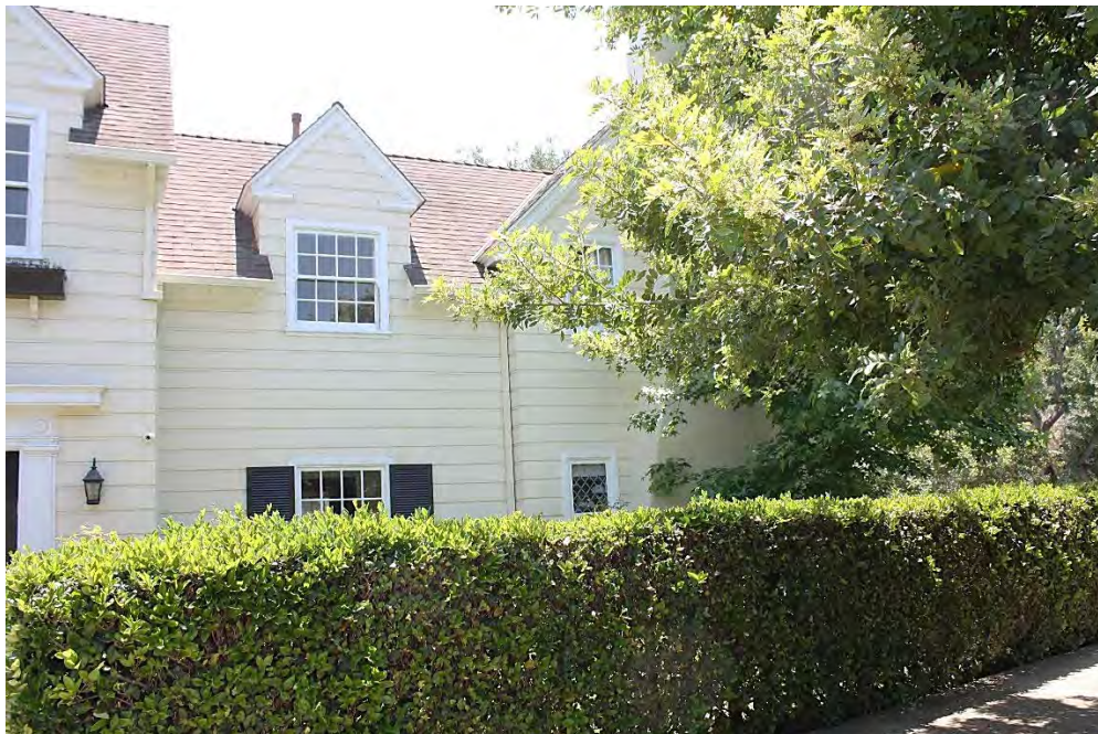
North hyphen: Pedimented dormer; cornice/brackets; 8-over-8 double hung fenestration. North elevation, west dependency: 6-over-6 fenestration either side of chimney; leaded diamond single fenestration either side of chimney on ground floor, view south.
