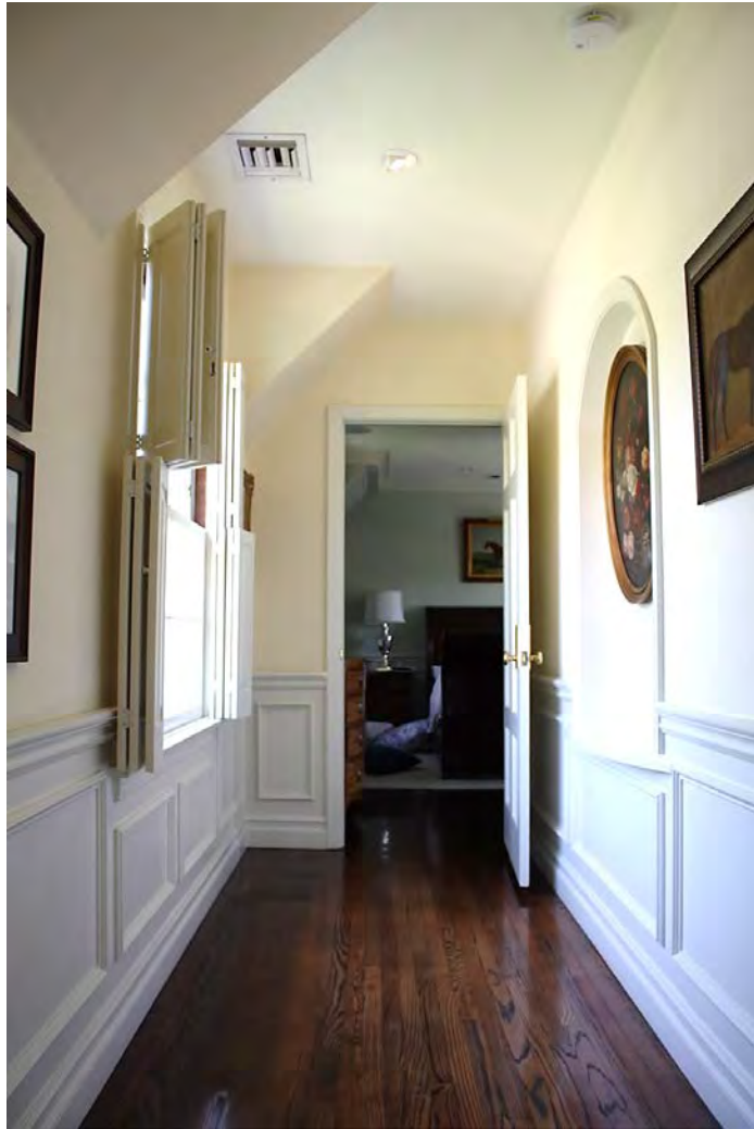
Second story west hall: Paneled wainscot; 8-over-8 double hung windows/vertically hinged folding Colonial shutters, north hall elevation; west bedroom, 6-panel door; curved grotto at hall south elevation, view west.
