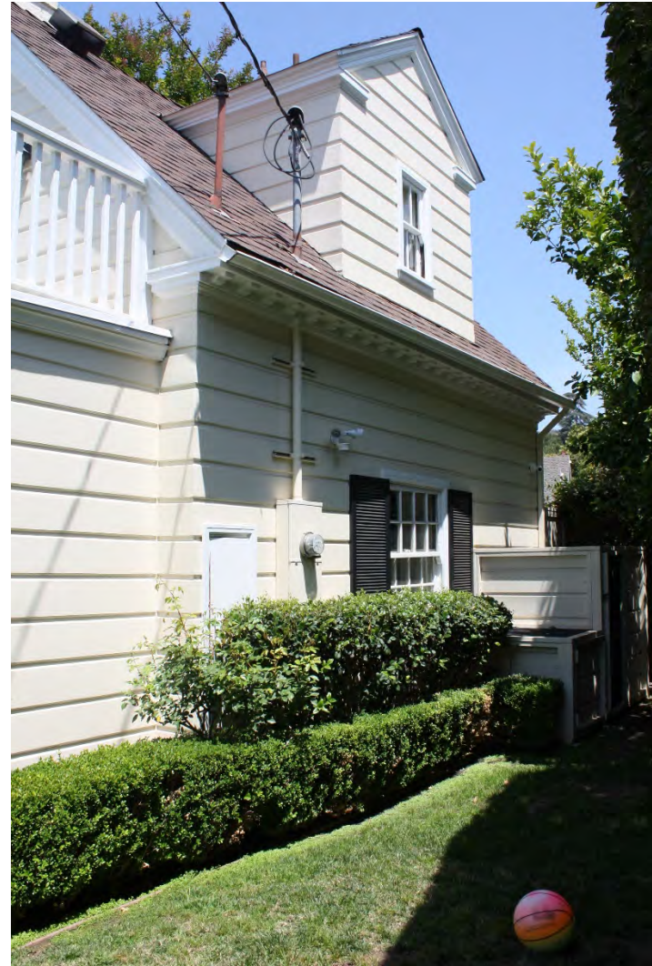
Garage, east elevation: Pedimented dormer above bracketed cornice, 8-over-8 double hung window/louvered shutters, view northwest.
