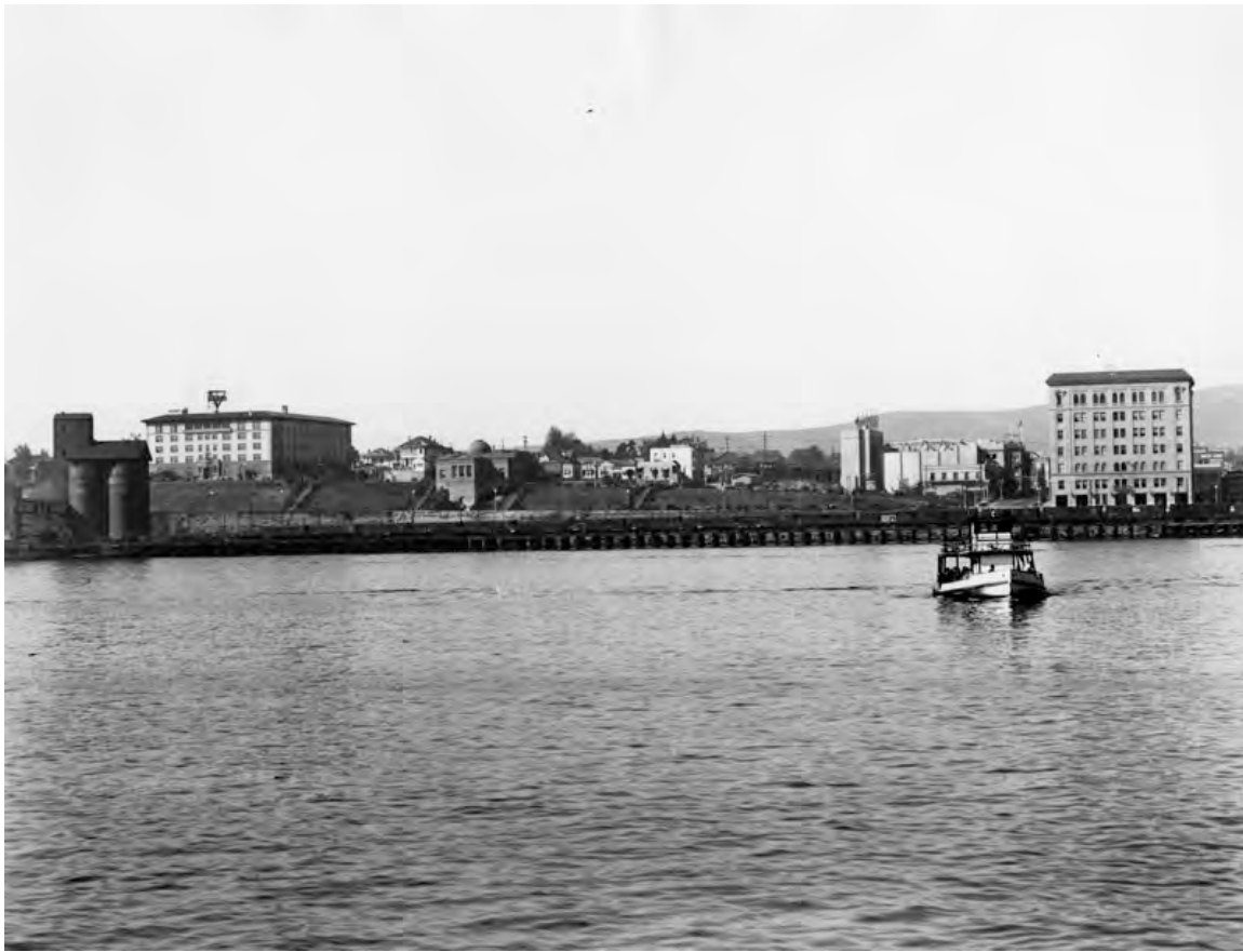
Photo D1: Army and Navy YMCA (left), viewed from the Main Channel of the Port of Los Angeles, c. 1930. Los Angeles Public Library
