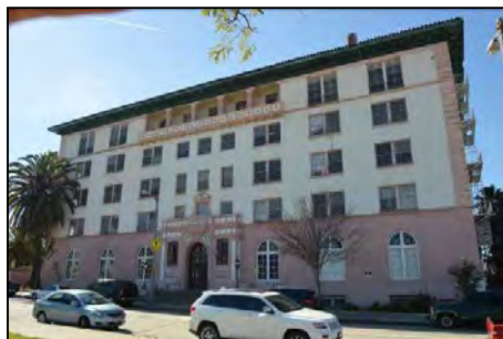
East (primary) elevation along S. Beacon St., view looking southwest (HRG, 2019)
