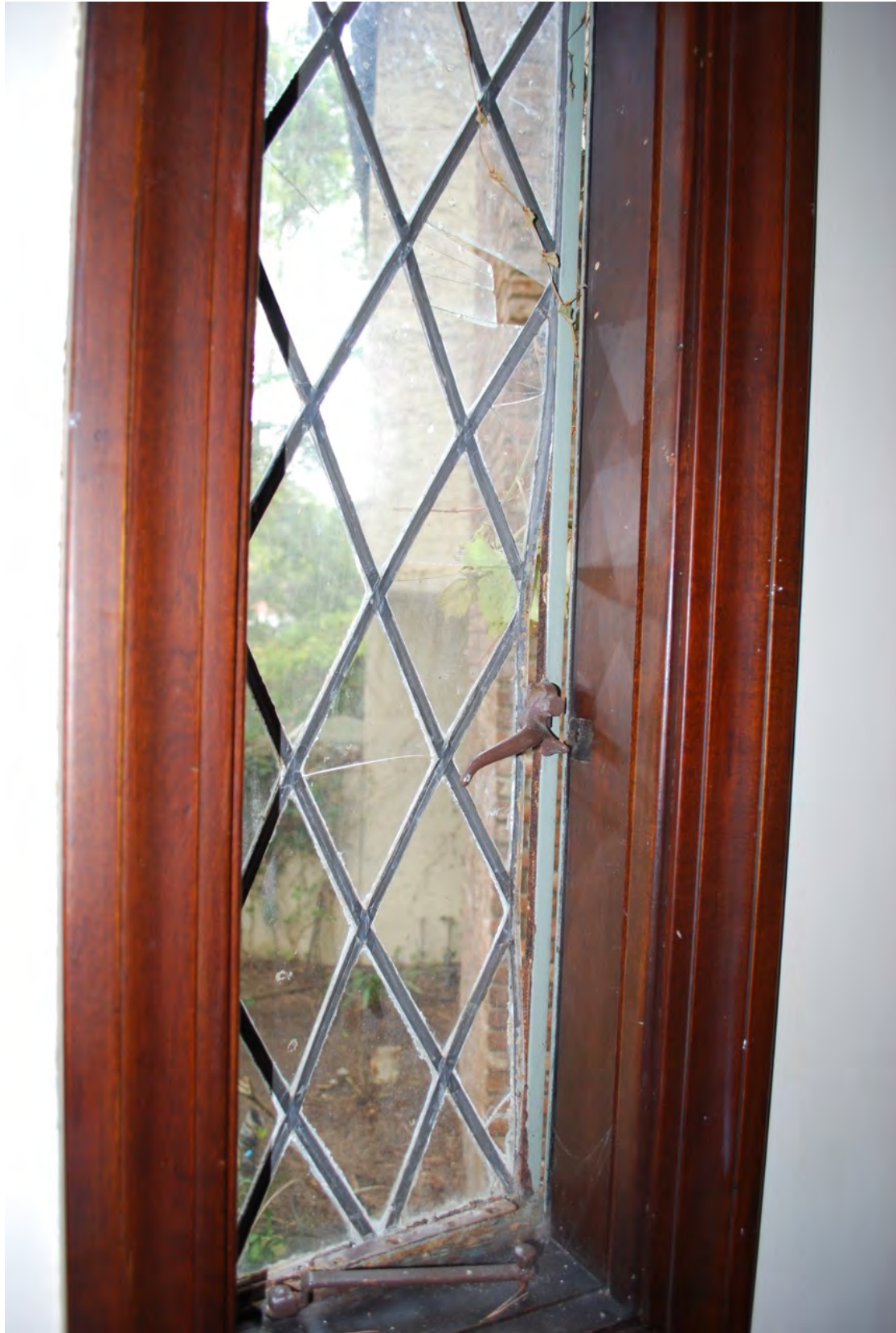
Figure 15 Leaded glass casement window showing damage, 2017. Photo credit: V.Withers
