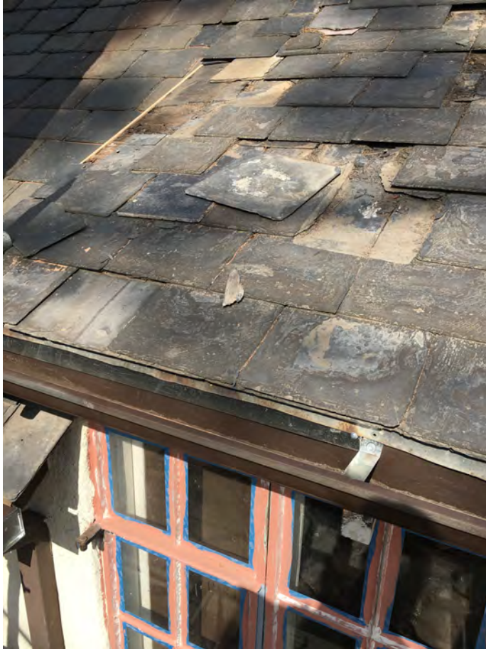
Figure 9 Slate roof condition (detail), 2017. Photo credit: Stuart Gulland
