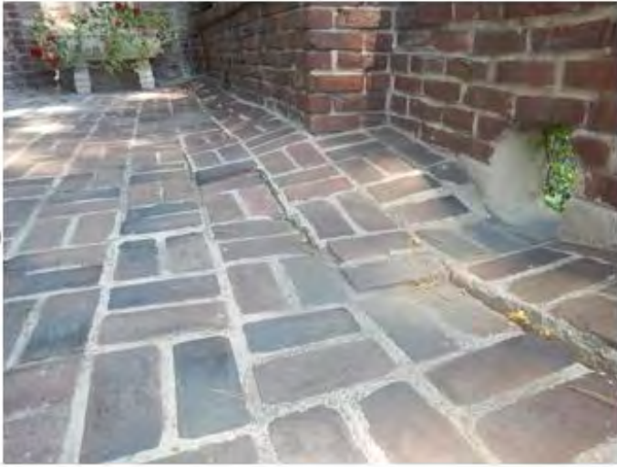
Figure 13 Front Terrace with subsidence of substrate, 2017. Photo credit: Stuart Gulland
