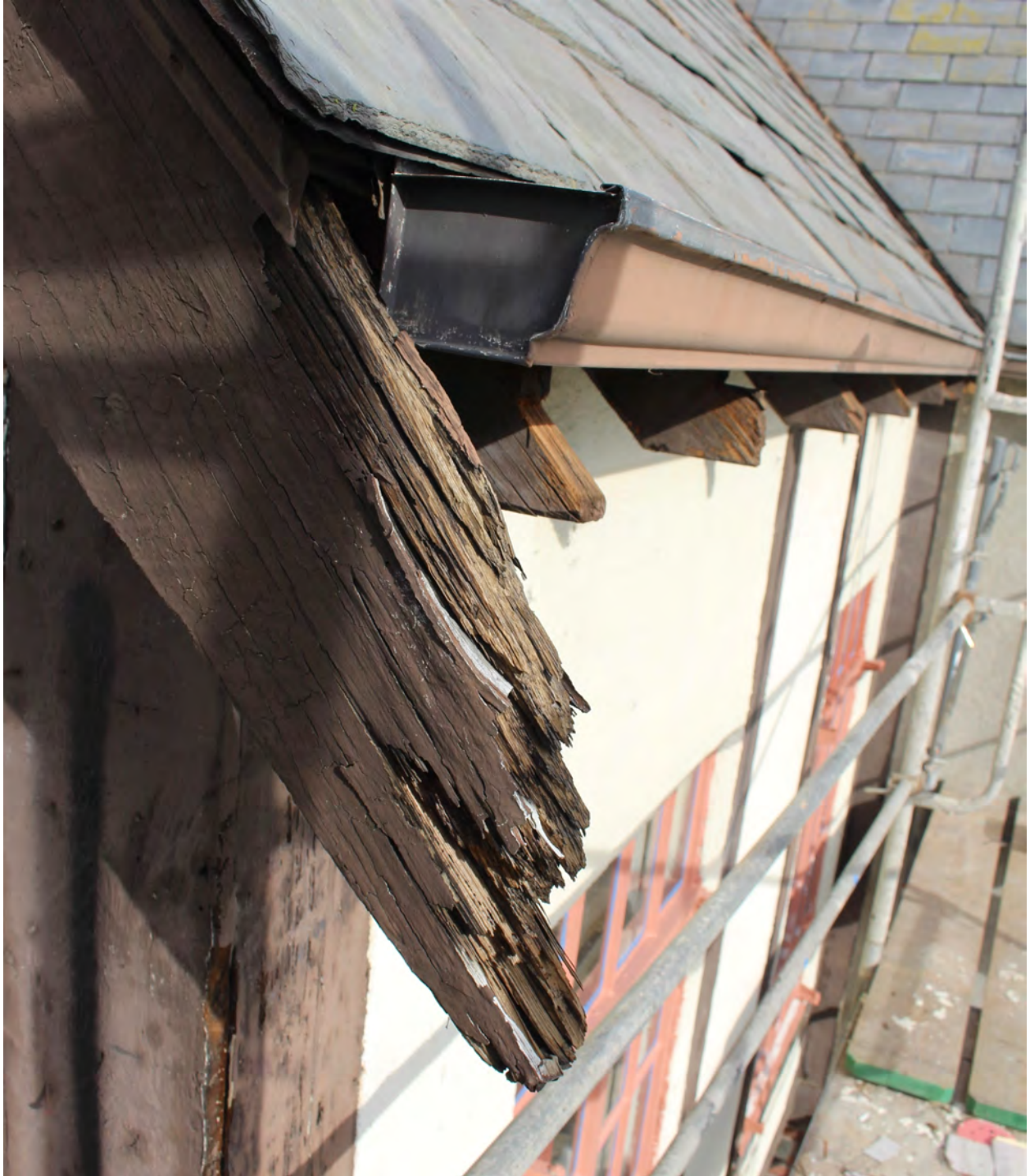
Figure 11 Exposed architectural wood elements suffering from deterioration, 2017. Photo credit: Stuart Gulland
