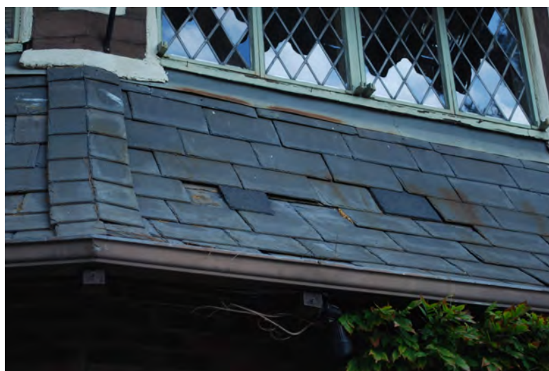
Figure 8 Slate roof detail showing missing slates, 2017. Photo credit: V.Withers
