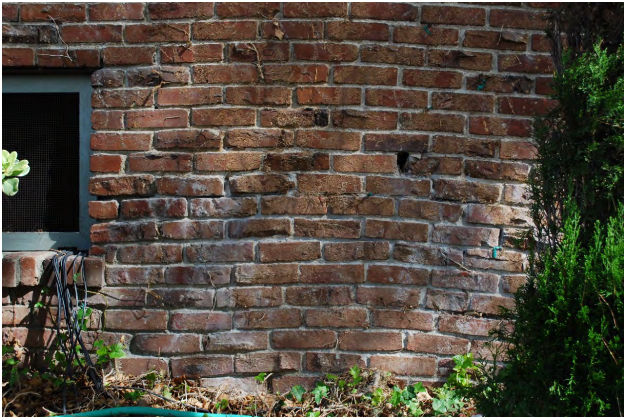
Figure 14 Representative brick wall, showing repair mortars, 2017. Photo credit: V. Withers
