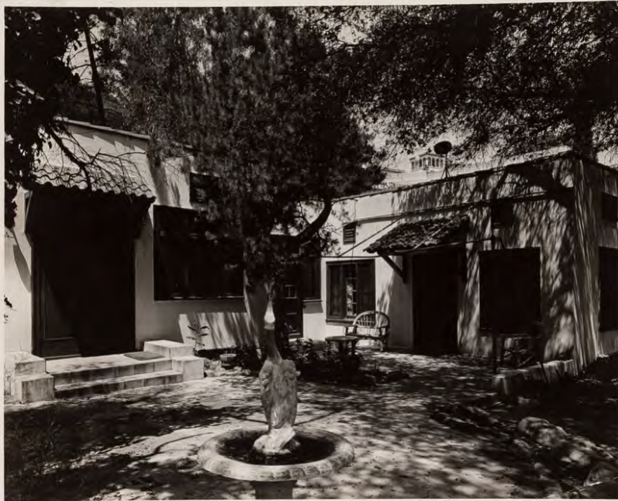
Former classroom building from the patio
