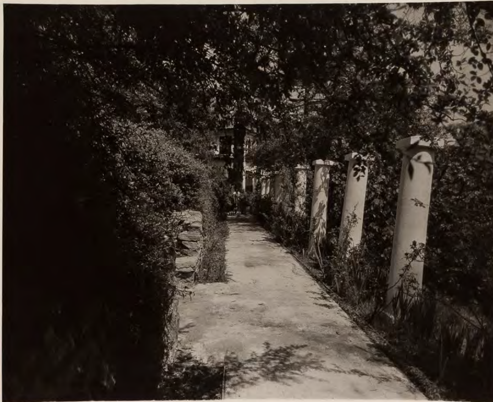
Colonnade to the south of the house
