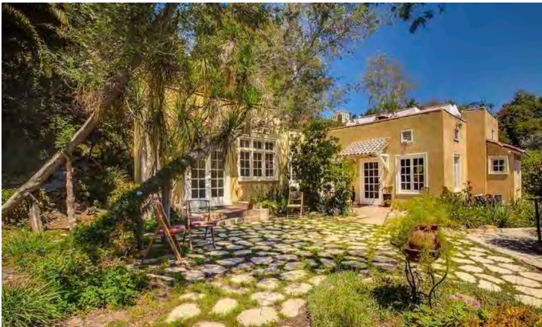
Guest house, former classroom building
