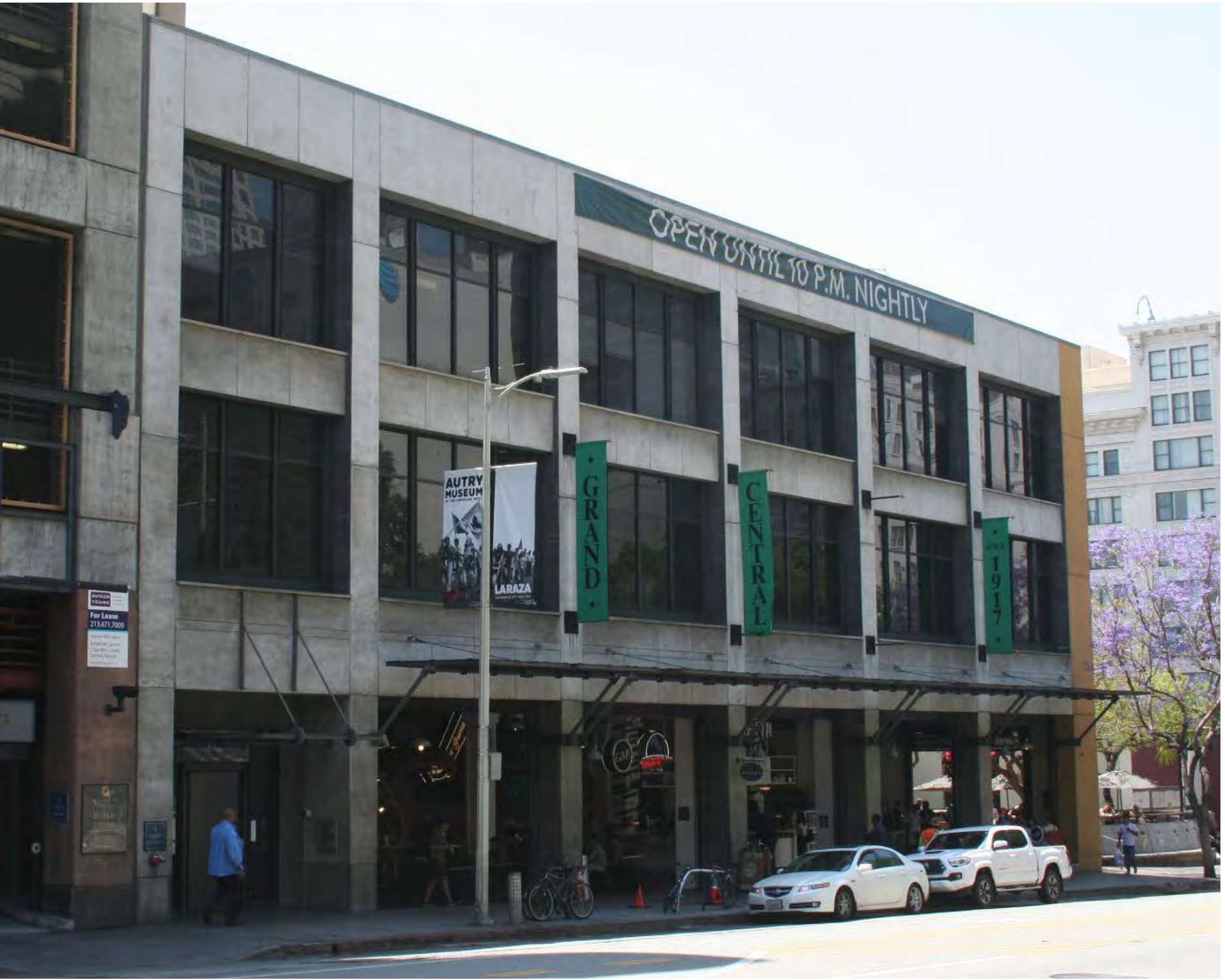
Laughlin Annex/Lyon Building, view of west elevation. (GPA Consulting, July 2018)
