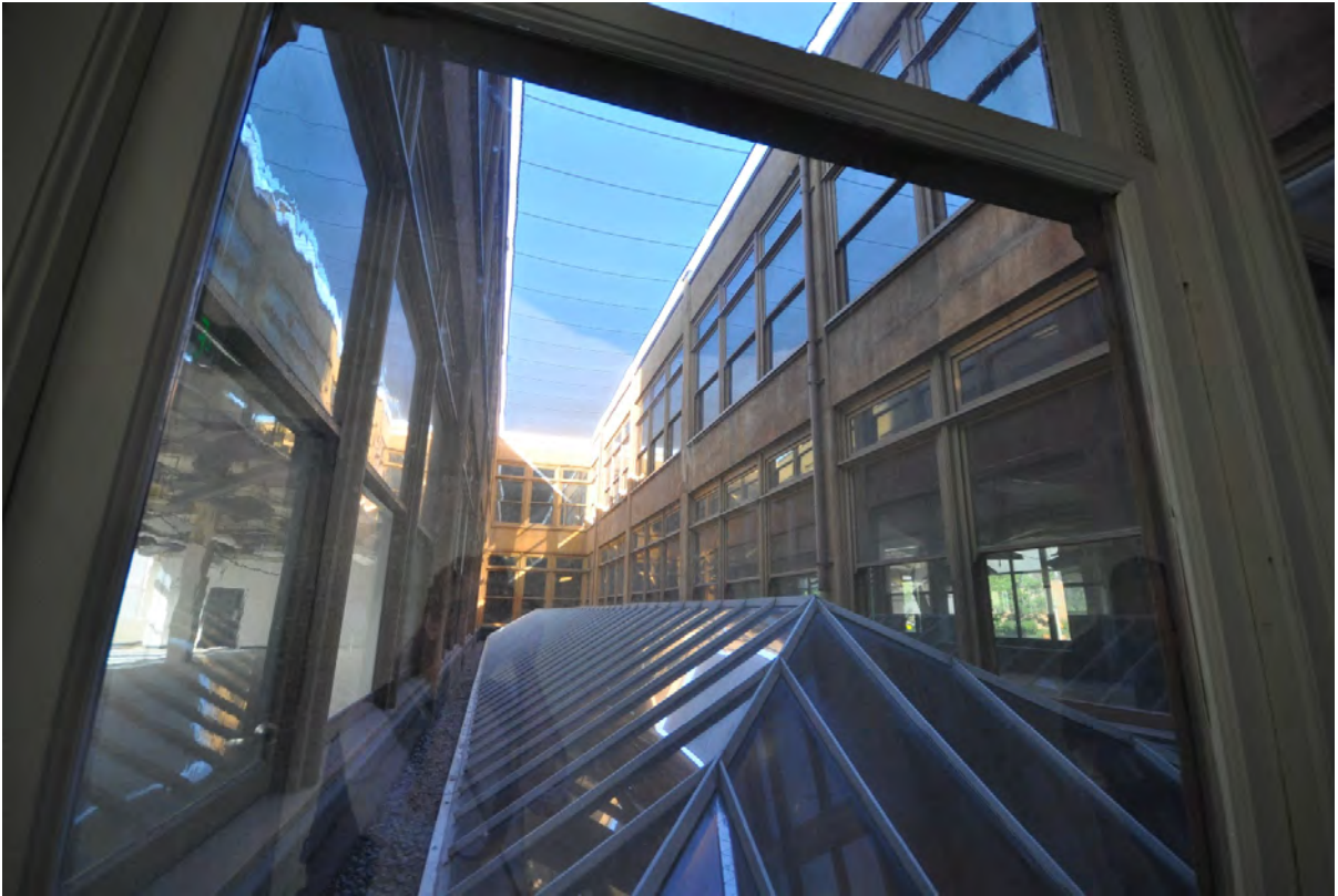
Laughlin Annex, view of light well. (GPA Consulting, July 2018)
