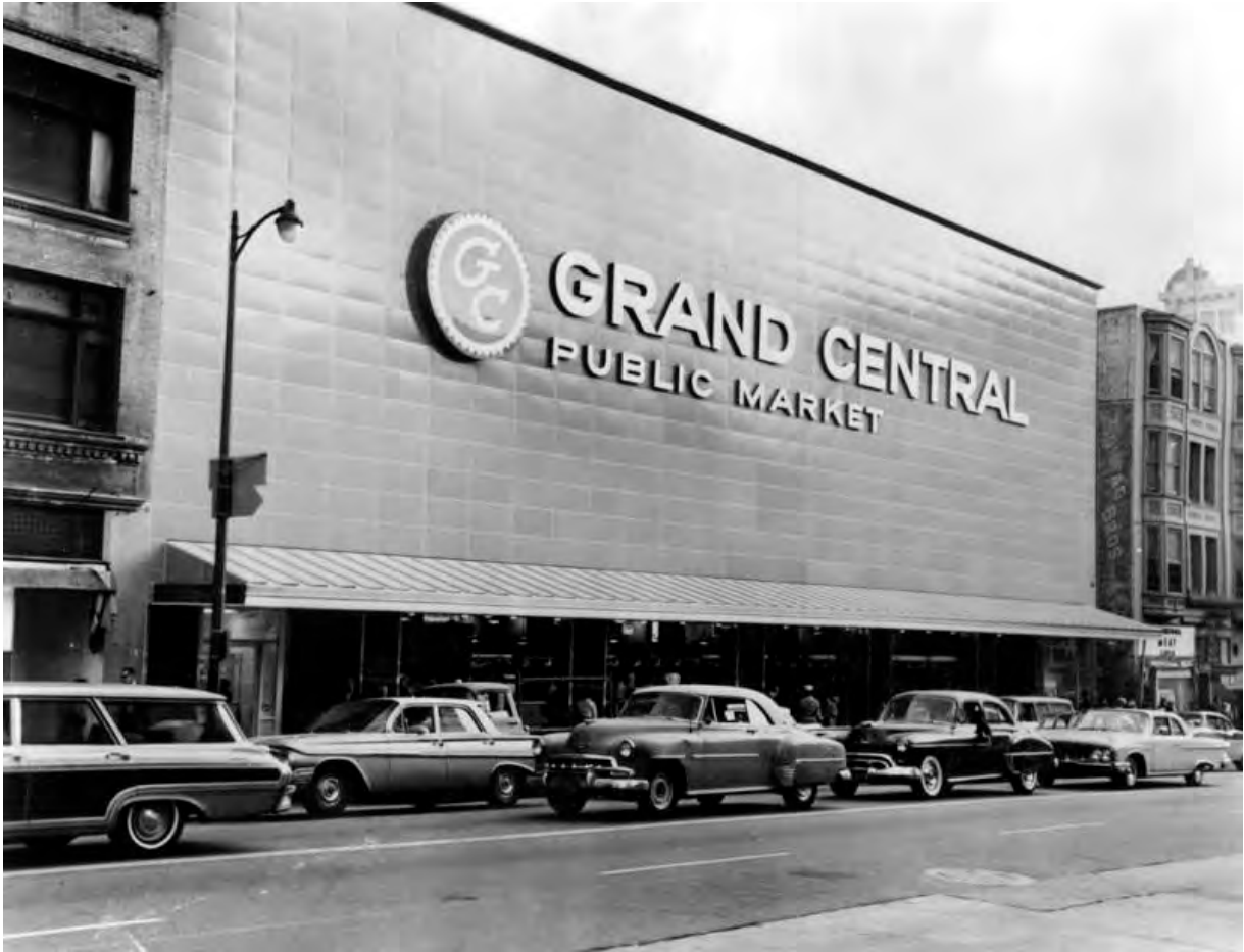
Hill Street elevation of Grand Central Market (Laughlin Annex) with new metal façade, 1962. (Los Angeles Public Library Digital Photo Collection)
