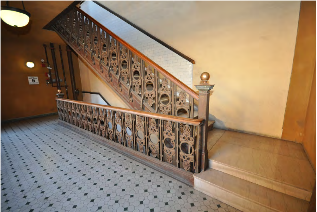
Homer Laughlin Building, view of original stair at north end of building. (GPA Consulting, July 2018)
