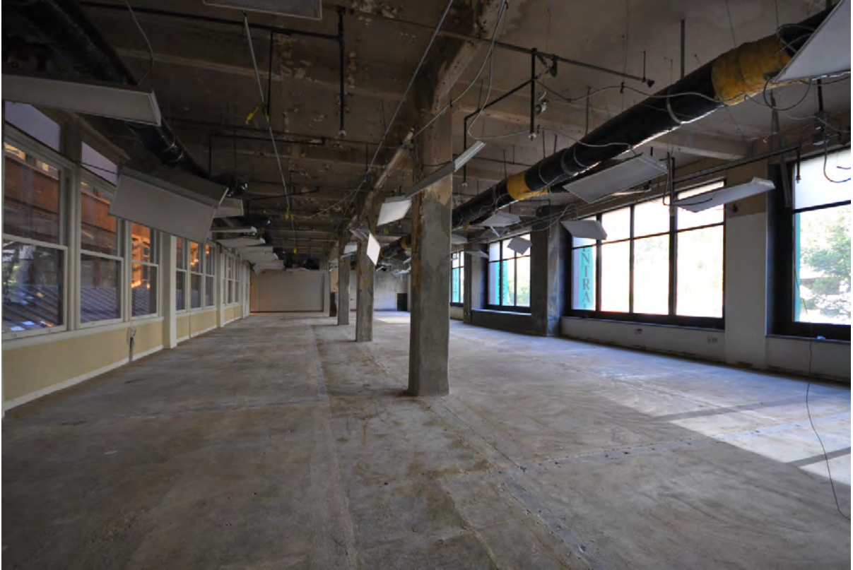
Laughlin Annex, view of typical upper-floor office space. (GPA Consulting, July 2018)
