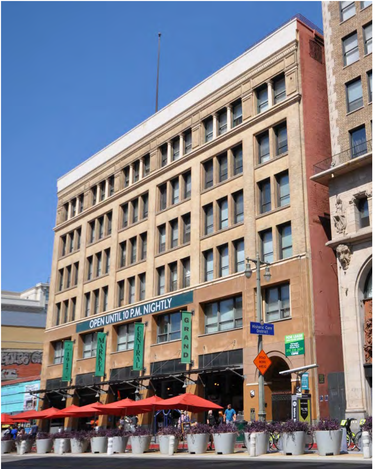
Homer Laughlin Building, view of east elevation. (GPA Consulting, July 2018)
