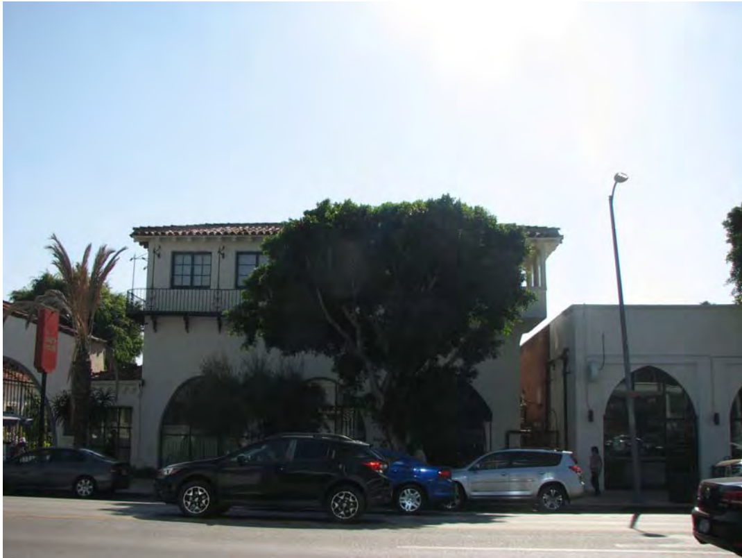
Fred C. Thomson Building, front facade, 6526-40 Sunset Boulevard, May 30, 2017, (Charles J. Fisher photo)
