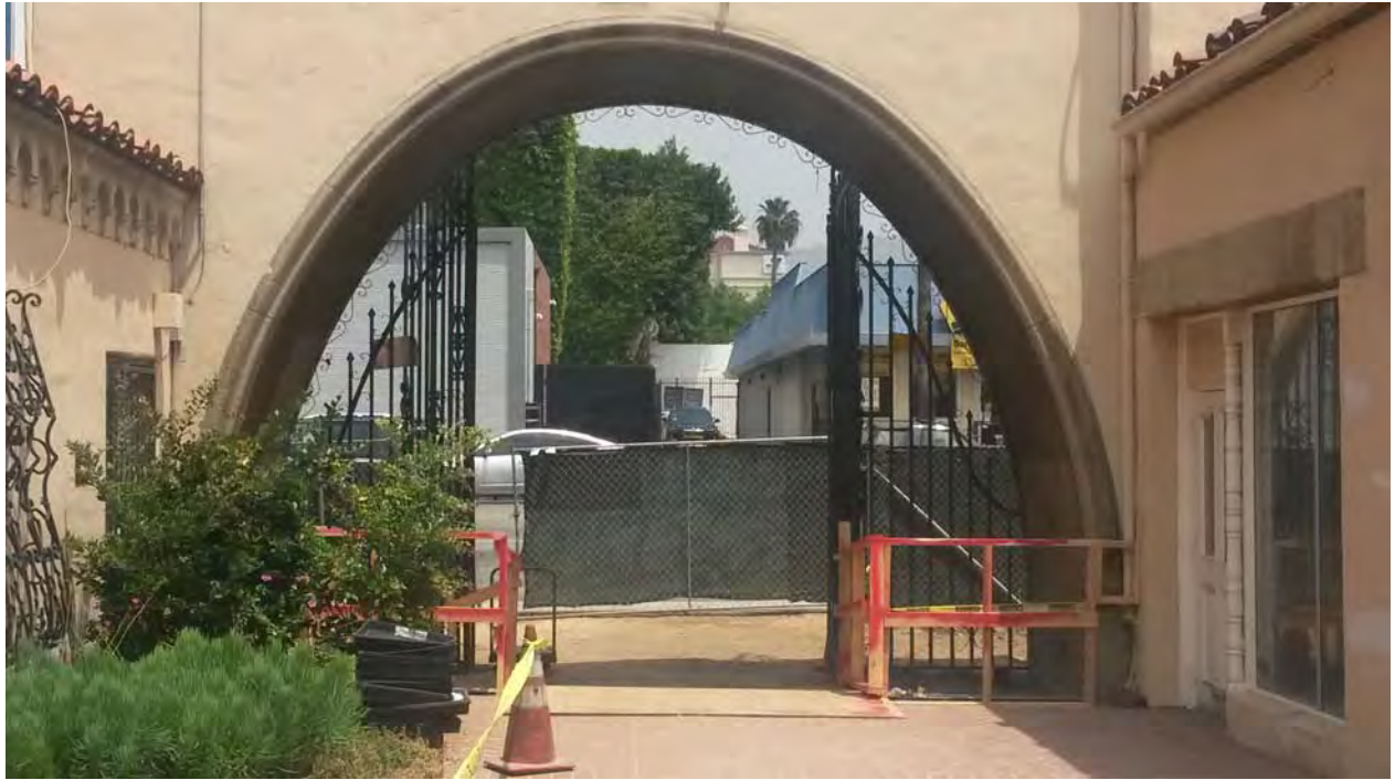
Fred C. Thomson Building, looking out arch, 6526-40 Sunset Boulevard, May 30, 2017, (Charles J. Fisher photo)
