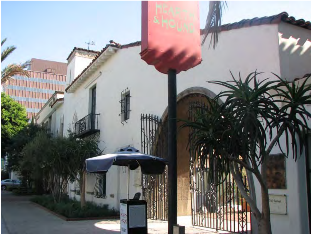
Fred C. Thomson Building, front arched entry, 6526-40 Sunset Boulevard, October 24, 2018, (Charles J. Fisher photo)
