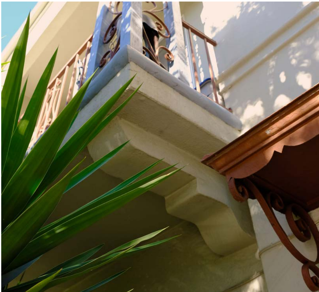
Giant corbels support the three balconies on the west façade. (Luftman 2019)
