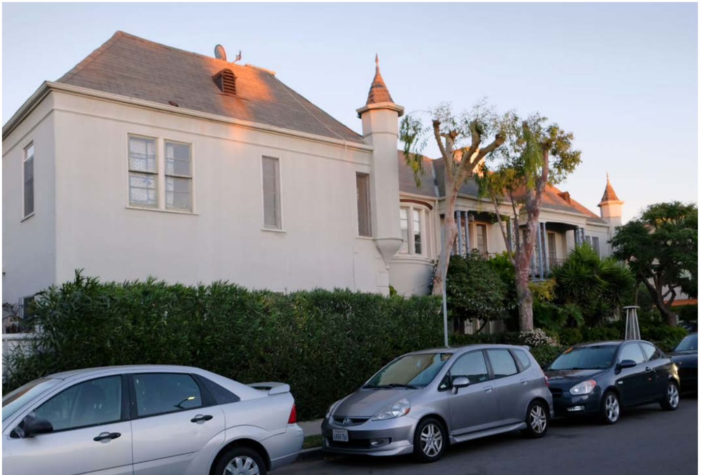
View southeast of the west façade.(Luftman 2019)
