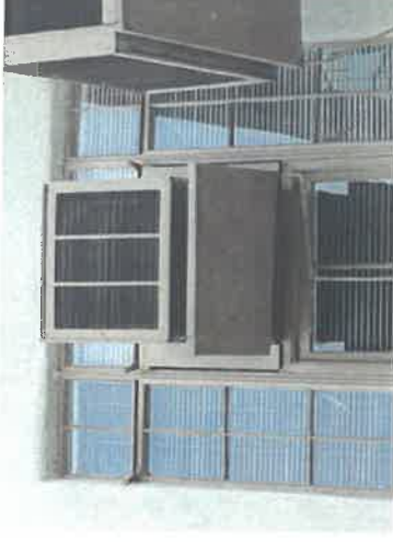
STEEL CASEMENT WINDOW WITH AIR CONDITIONERS
