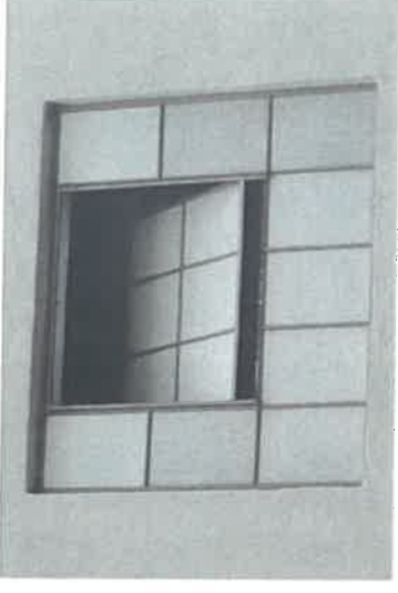
STEEL PIVOT WINDOW WITH BACK PAINTED GLASS
