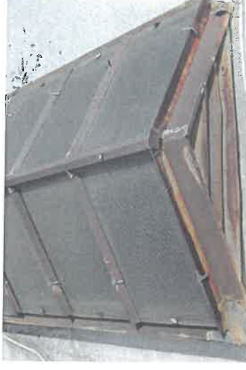
TYPICAL RUSTED SKYLIGHT
