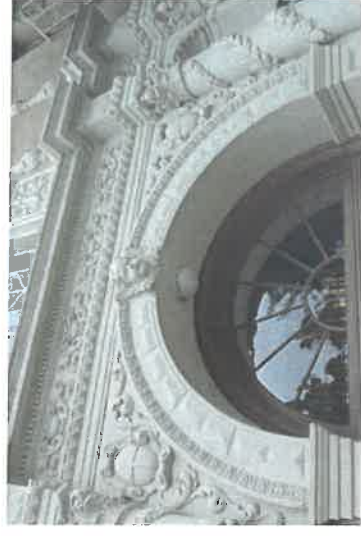
CAST CONCRETE ENTRANCE DETAIL
