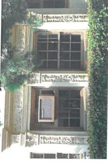
WOOD DOUBLE HUNG WINDOW IN CAST SURROUND
