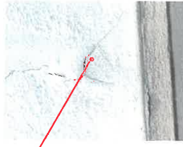
SUSPECTED WATER DAMAGE OF CEMENT PLASTER
