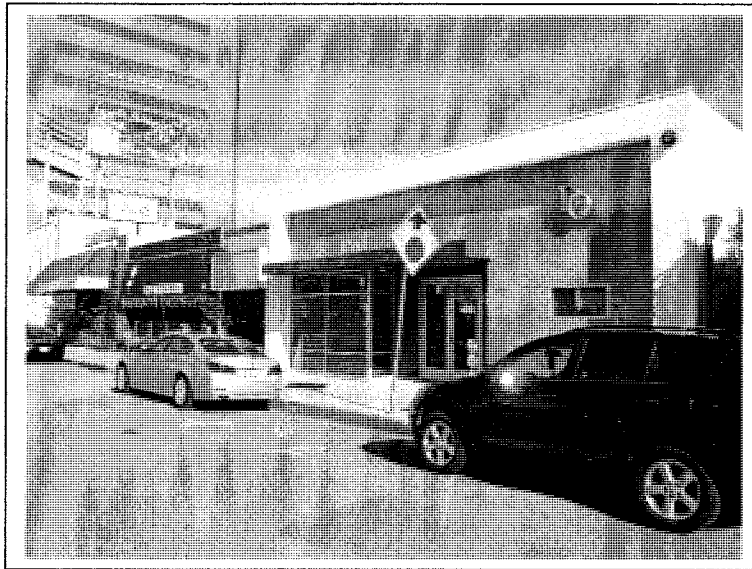
Picture (7). Property north of the Subject Site (Commercial Area / Retail Stores)
