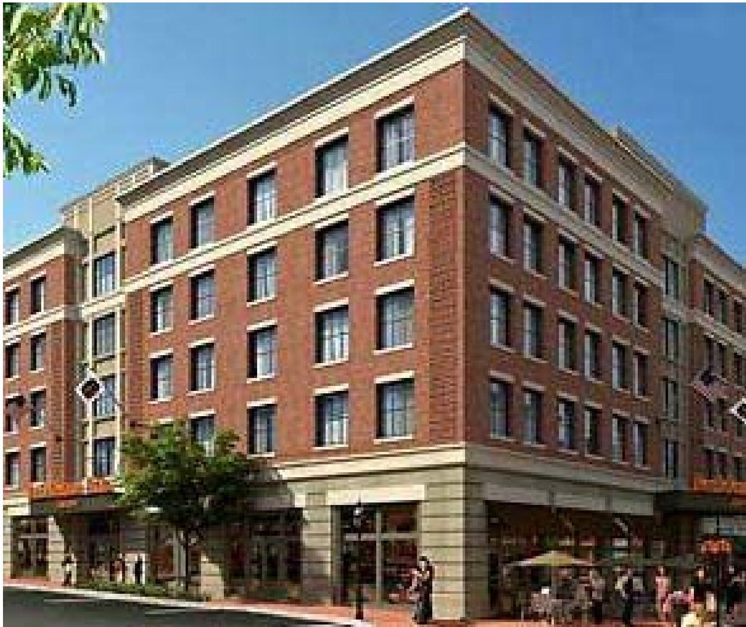
4.05 - GFRC DECORATIVE BANDS @ ROOFLINE AND 7TH FLOOR
