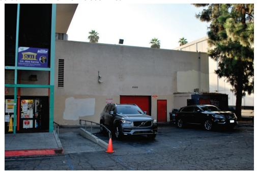
The west elevation of the northern building wing has also undergone numerous alterations and no longer resembles its original appearance. The elevation is clad in stucco and features modern signage and aluminum frame glass doors with fixed sidelights. A metal awning projects from the elevation wall above the entrance (Figure 21).
