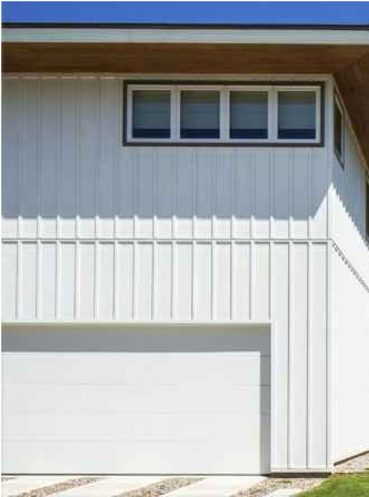
BOARD AND BATTEN EXTERIOR CLADDING SCALE: NTS
