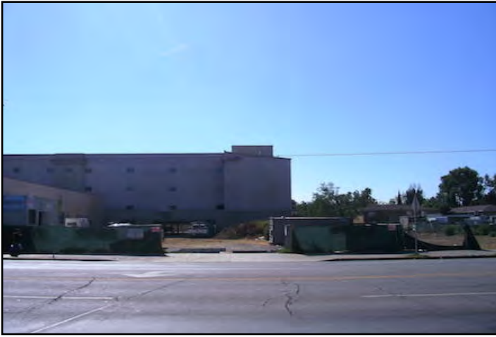
View 1: From the north side of Victory Boulevard, looking south at the Project Site.
