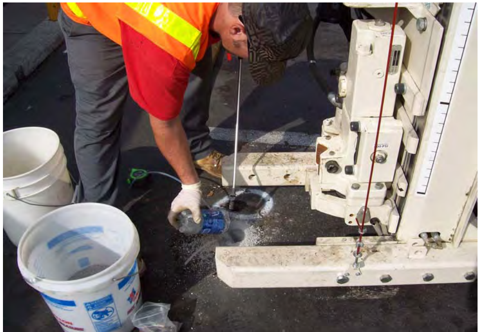
Photograph No. 4: SAE installing soil vapor probes in soil boring B11
