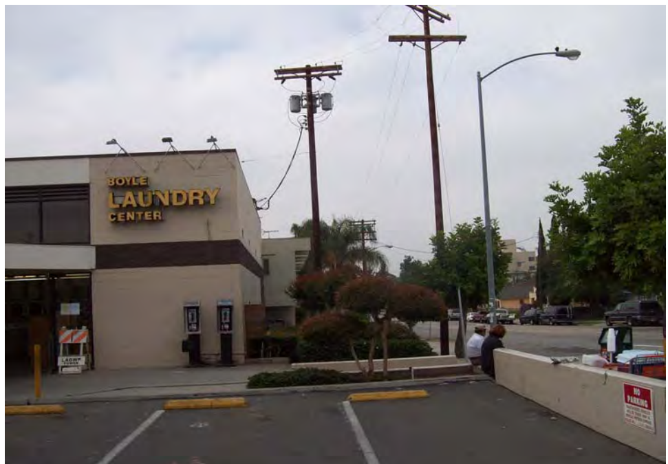
Photograph No. 4: Pole-mounted transformers located at the southwestern corner of the site.
