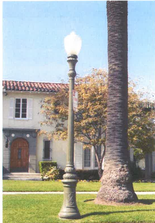
Figure 16: Windsor Square custom streetlight installed in Tract No. 1390, refitted with single acorn globe. Found along Plymouth, Windsor, Lorraine and Irving Boulevards, between 3 rd Street and Wilshire Boulevard. February 2002.
