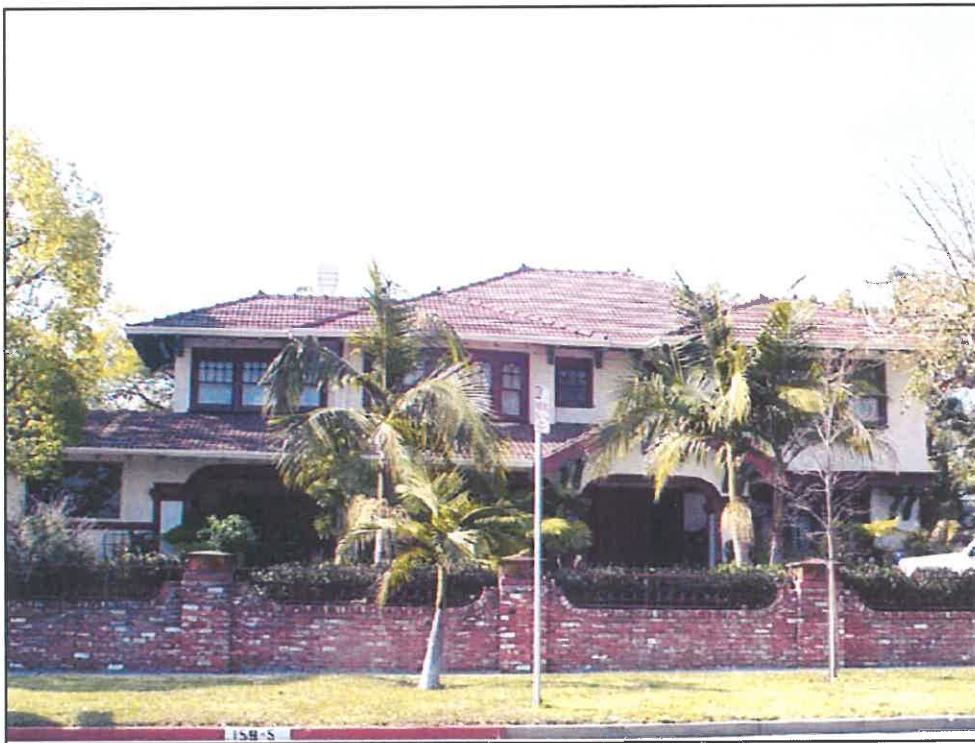
Figure 33: Mission Revival Residence, 159 South Van Ness Avenue, built 1912.
