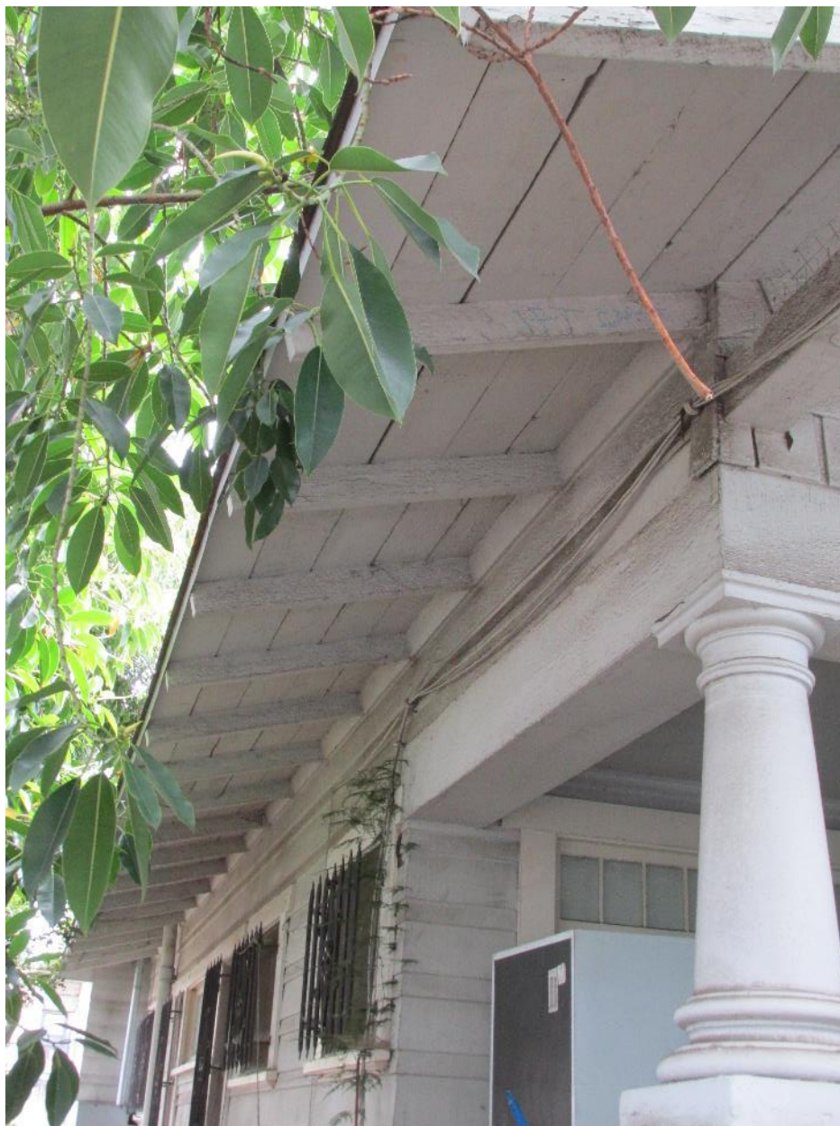
Figure 20. Front and Western Façade. Note the concrete porch support, the exposed rafters, and metal bars on western façade windows.
