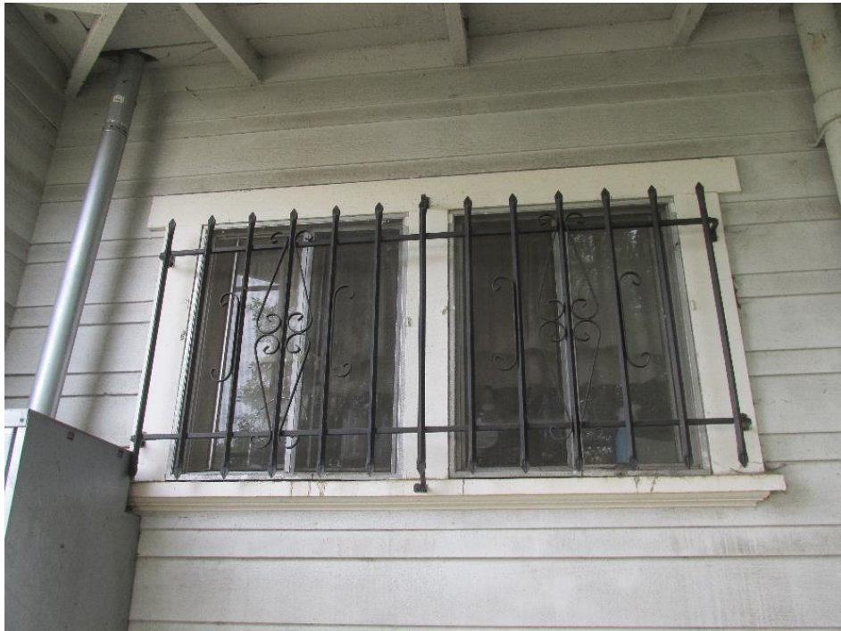
Figure 27. Western Façade Windows (cont). Close up of altered windows, modern aluminum framed.
