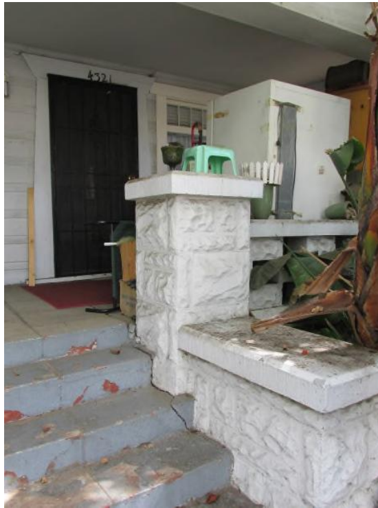
Figure 2. Front Porch 4321-4323 Burns Avenue. Note the concrete block used for railing detail.
