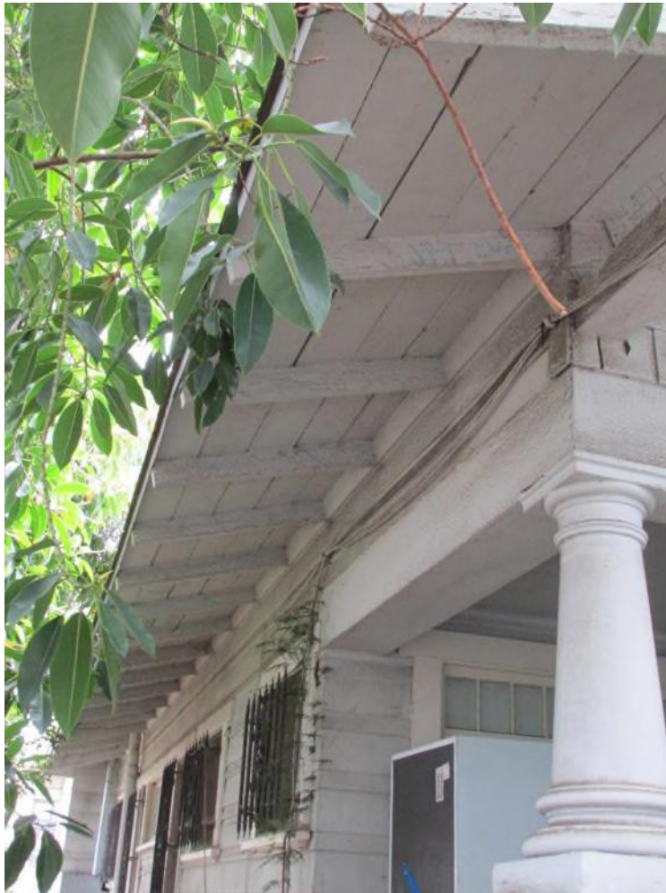
Figure 4. Front and Western Façade. Note the concrete porch support, the exposed rafters, and metal bars on western façade windows.
