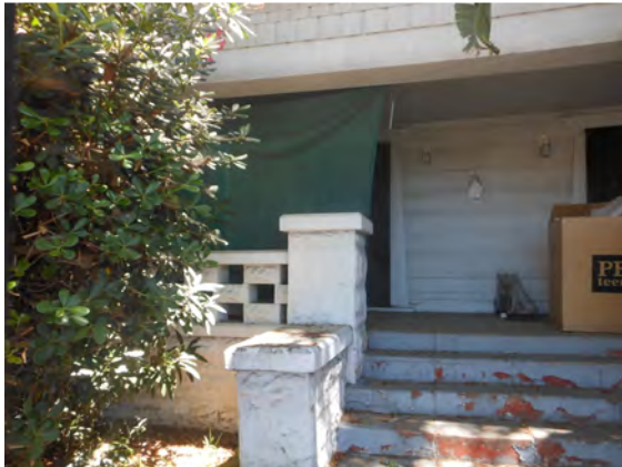
Front porch piers (without columns) and entry doors under porch
