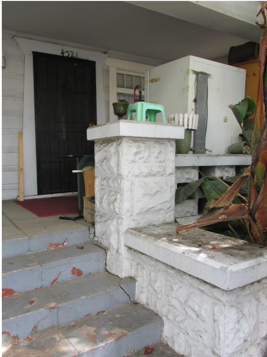
Figure 18. Front Porch 4321-4323 Burns Avenue. Note the concrete block used for railing detail.
