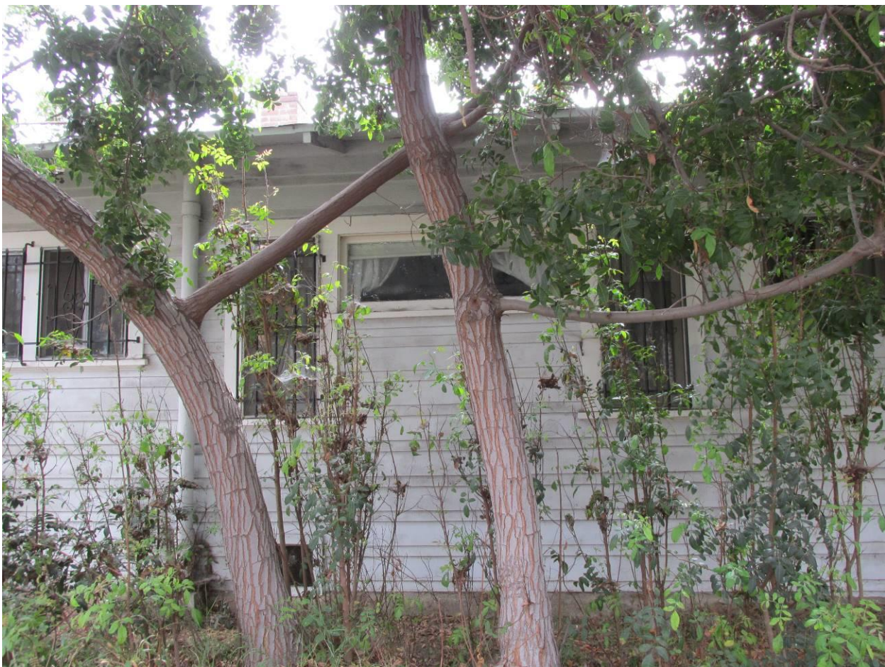
Figure 23. Western Façade Windows. Overgrown trees and brush obscure much of the buildings façades; nevertheless, it is still possible to see a mixture of modern aluminum framed and original windows behind the trees and security bars.
