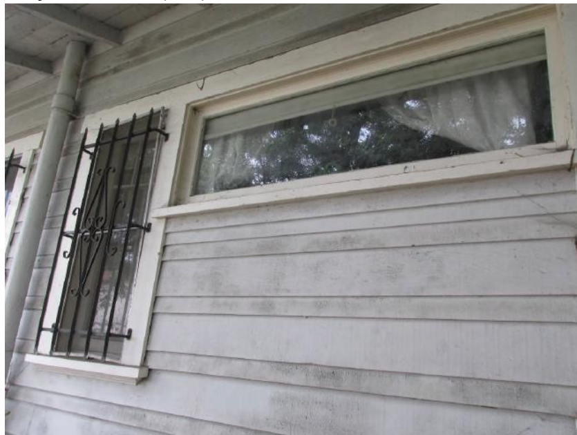
Figure 9. Western Façade Windows (cont). Close up of original fixed horizontal window.
