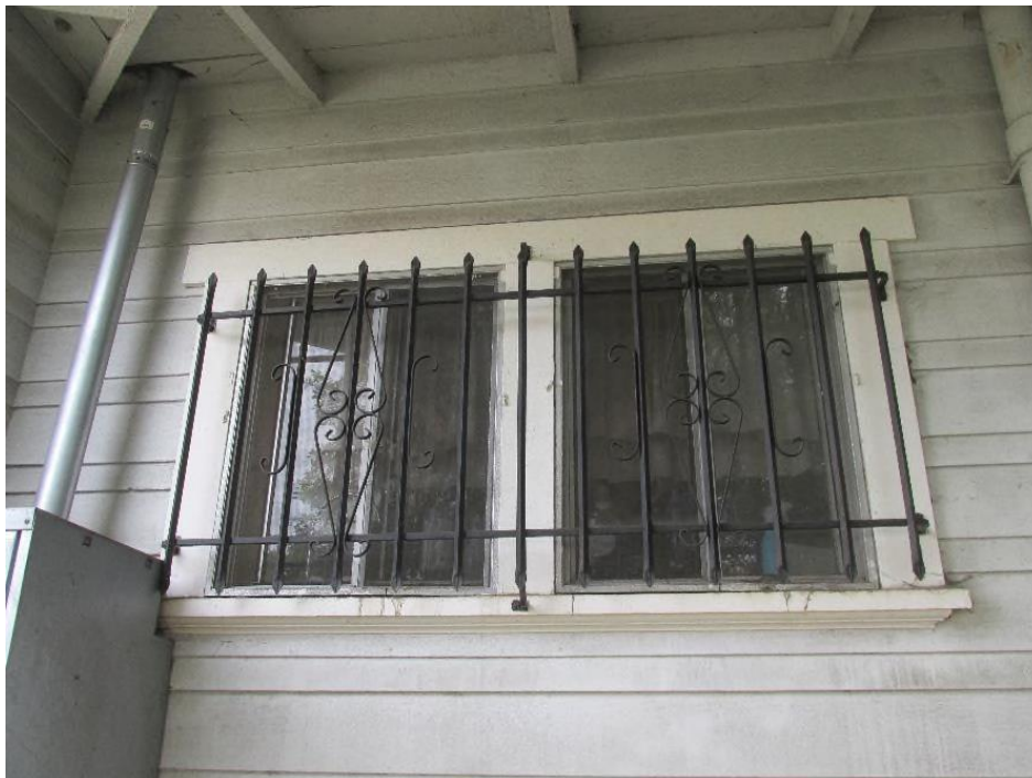
Figure 11. Western Façade Windows (cont). Close up of altered windows, modern aluminum framed.
