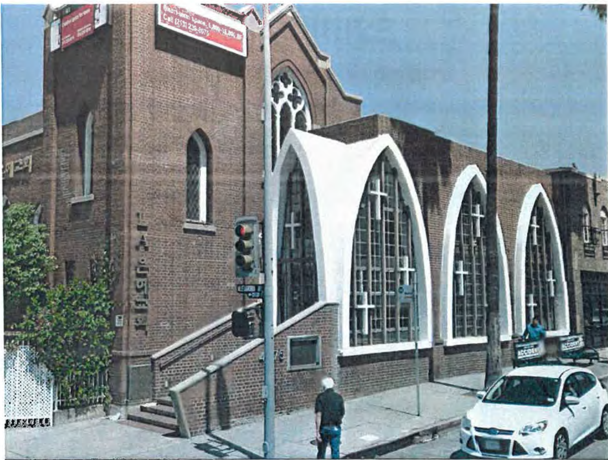
Figure 3. Southwest Elevation of the Existing Building.
