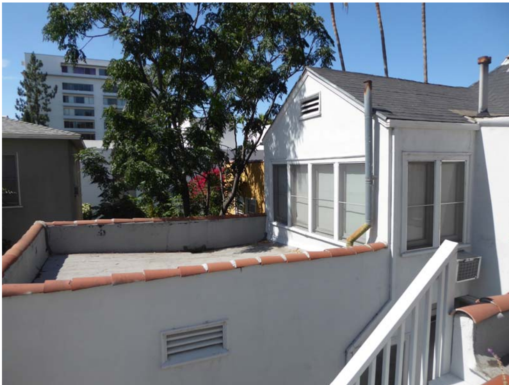
Figure 7: Partial second floor above south rear wing for unit 1920 with updated double-hung windows, facing southwest.
