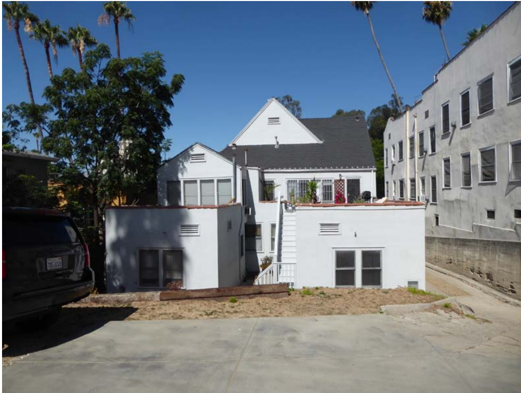
Figure 6: East façade from parking area at rear of the property, facing west.
