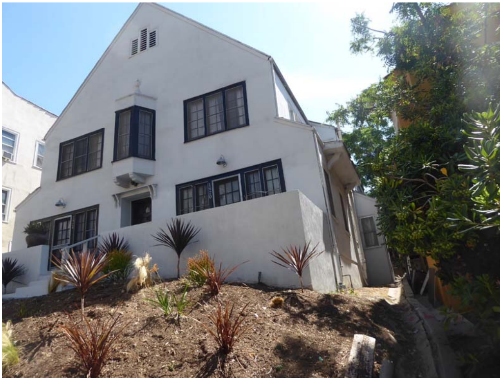
Figure 3: Spanish Colonial Revival brackets at entrance and canopy on south façade, lower-pitched roof at first floor adjacent to main gable.
