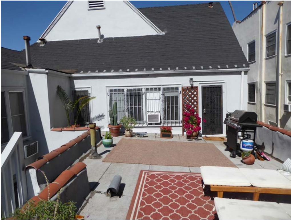
Figure 8: East façade at second floor, facing west-southwest.
