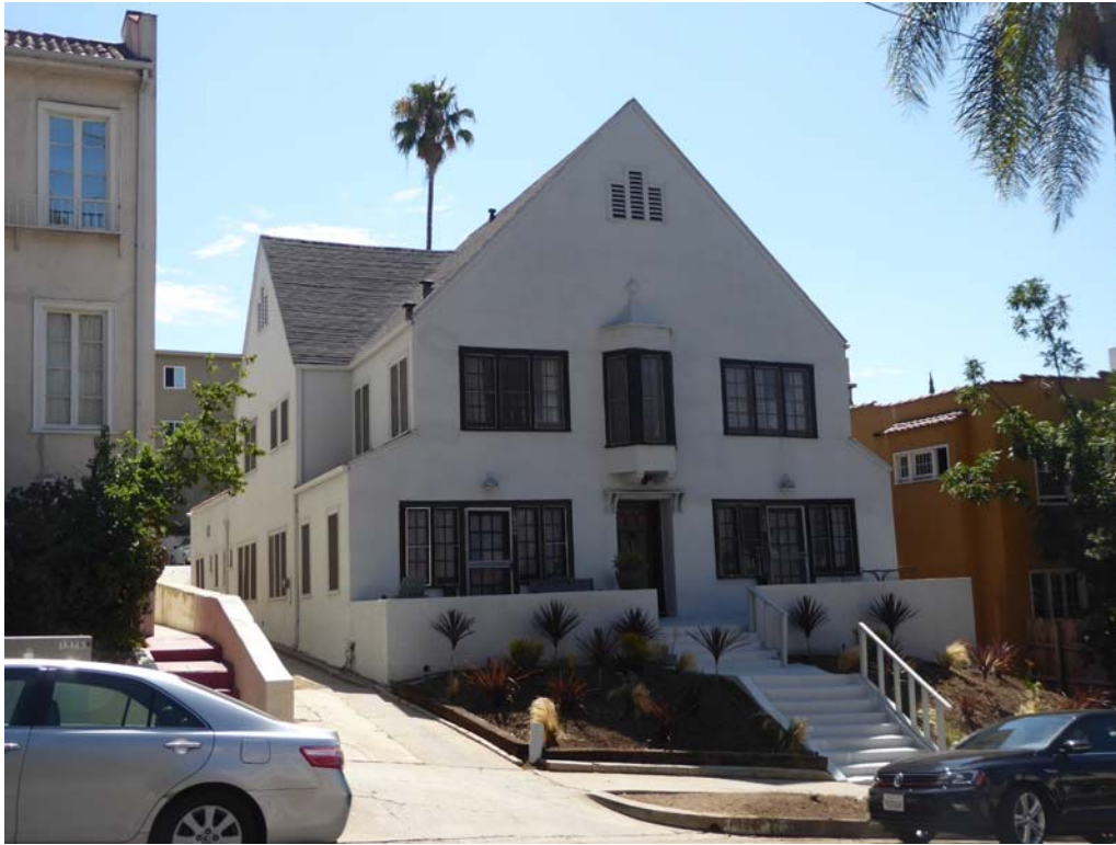
Figure 2: North and west façades, facing southeast.
