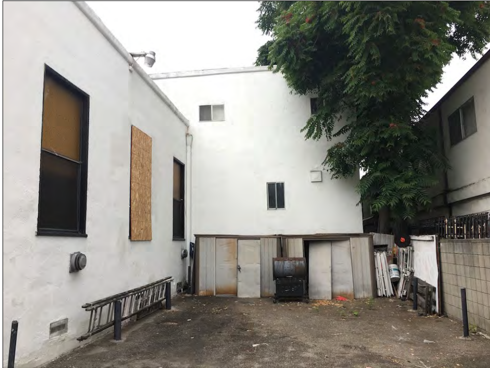
Figure 4: Subject property, west elevation (left) and north elevation (right), from surface parking lot located west of front portion of building, view south (McGee, 2017)
