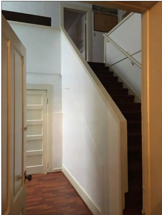
Figure 33: Subject property, interior, 1st floor, west stair to 2nd floor, door to day care at left, view southwest (McGee, 2017)
