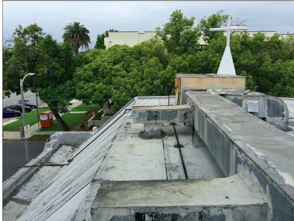
Figure 12: Subject property, roof, view north (Dan Stein, 2017)
