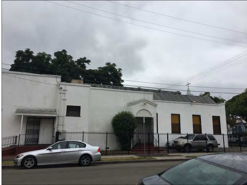
Figure 7: Subject property, east elevation, view northwest (McGee, 2017)
