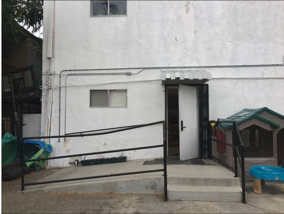
Figure 9: Subject property, south elevation, from rear yard, view north (McGee, 2017)
