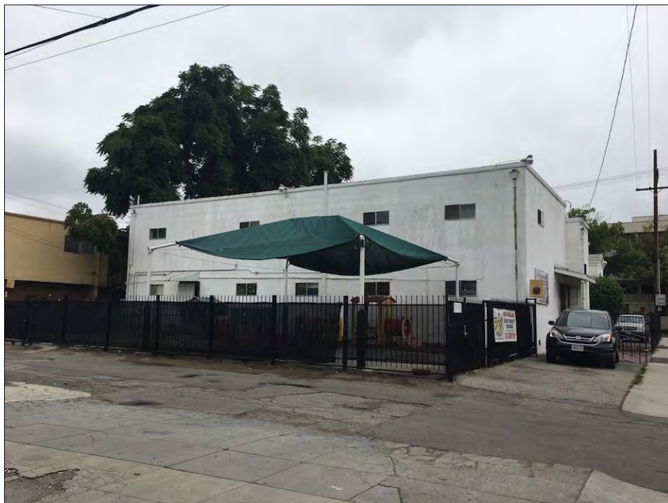
Figure 8: Subject property, south elevation (left) and east elevation (right), view northwest (McGee, 2017)
