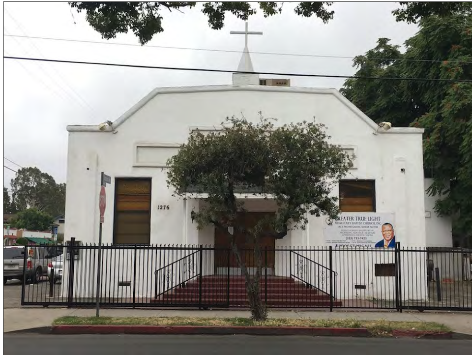
Figure 1: Subject property, north façade, view south (McGee, 2017)
