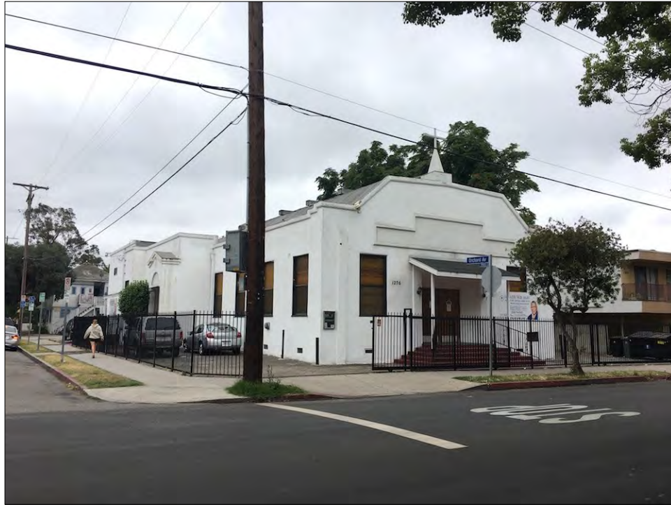
Figure 5: Subject property, north façade (right) and west elevation (left), view southwest (McGee, 2017)
