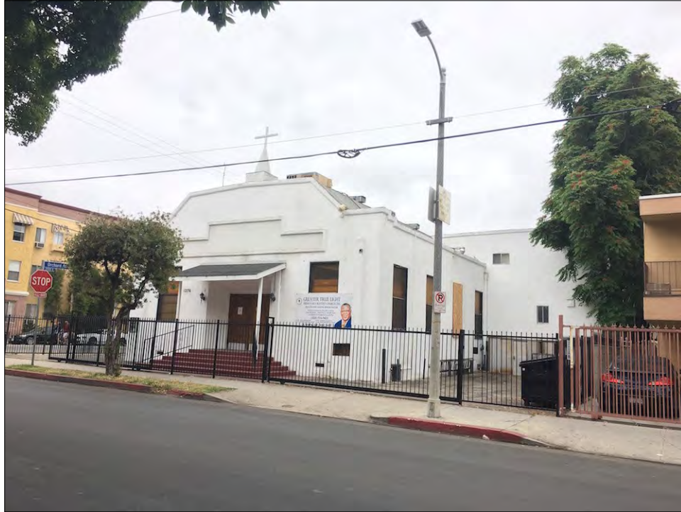
Figure 3: Subject property, north façade (left), west elevation (right), view southeast (McGee, 2017)
