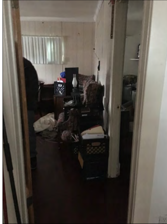
Figure 38: Subject property, interior, 2nd floor, office (typical) (McGee, 2017)
