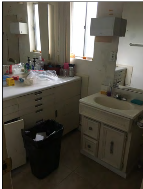
Figure 37: Subject property, interior, 2nd floor, restroom (typical) (McGee, 2017)
