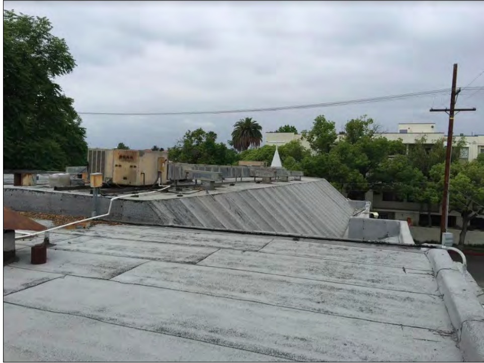
Figure 11: Subject property, roof, view northwest (Dan Stein, 2017)
