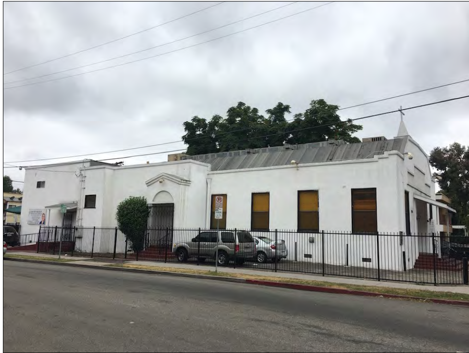
Figure 6: Subject property, north façade (far right) and east elevation (center), view southwest (McGee, 2017)
