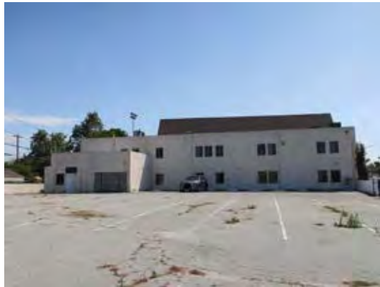
West façade, overall view east (ARG, 2018).
