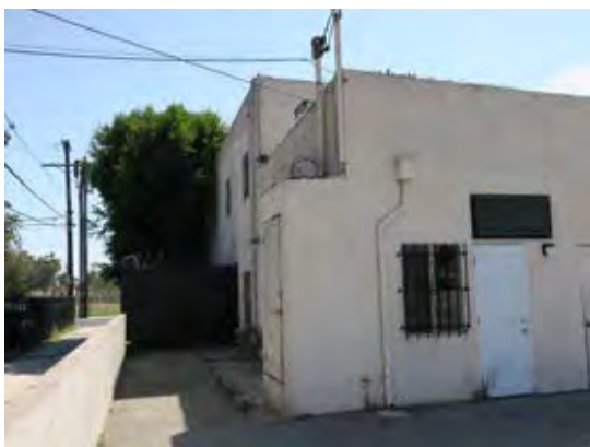
North façade, overall view southeast (ARG, 2018).
