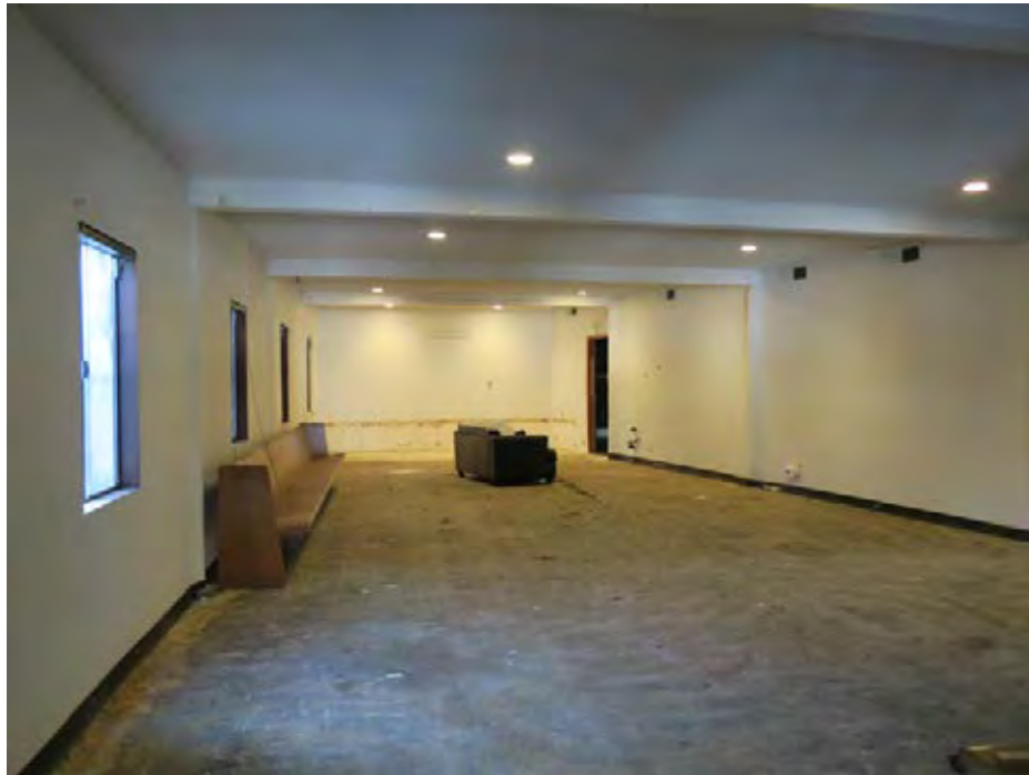
View east in the first-floor assembly room (ARG, 2018).
