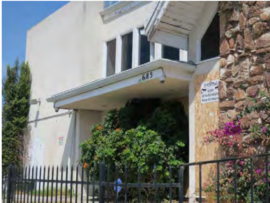
View northwest at the education wing south façade (ARG, 2018).
