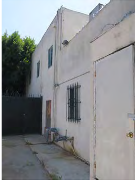
View of the north façade fenestration (ARG, 2018).
