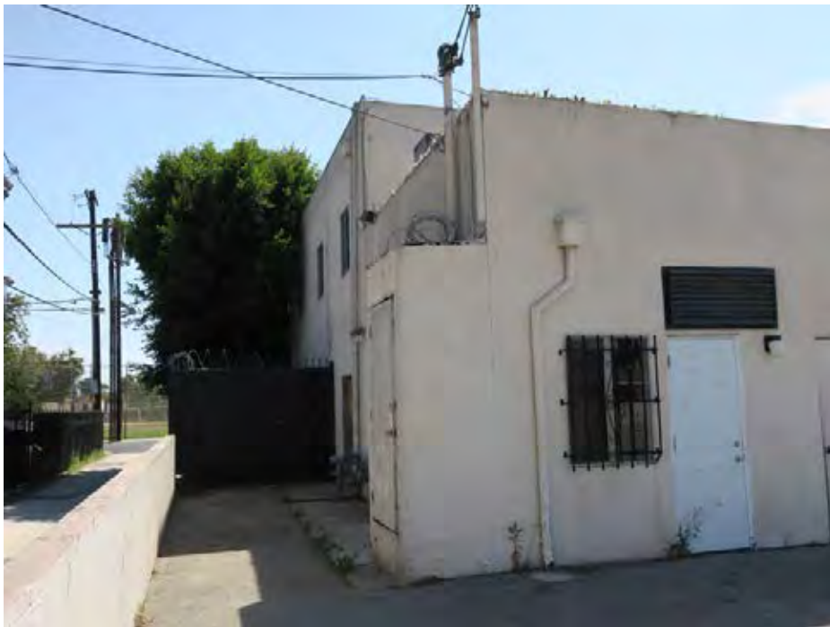
North façade, view east (ARG, 2018).
