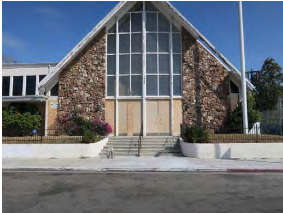
View north at the sanctuary south façade (ARG, 2018).
