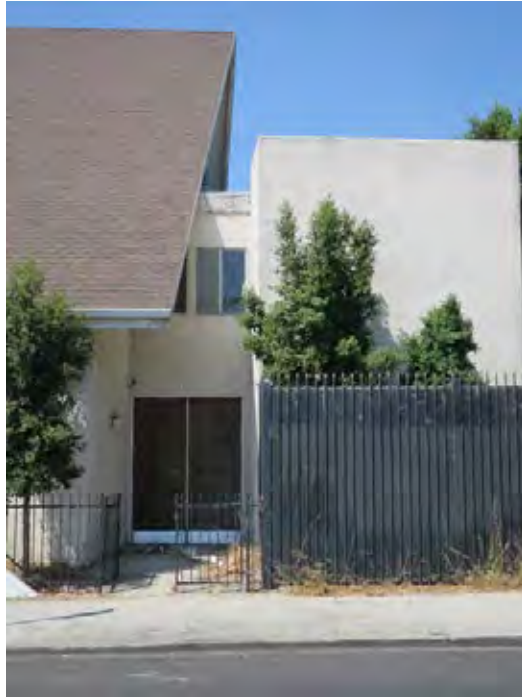
Secondary (east) façade, view west at northern education wing (ARG, 2018).
