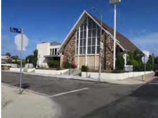
Primary south façade, overall view northwest (ARG, 2018).
