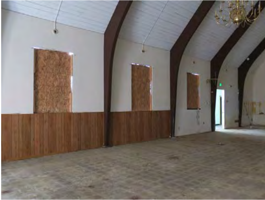
Sanctuary main room, view northwest (ARG, 2018).
