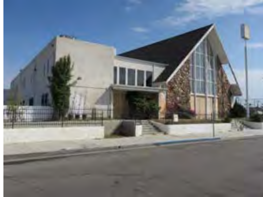
Primary south façade, overall view northeast (ARG, 2018).
