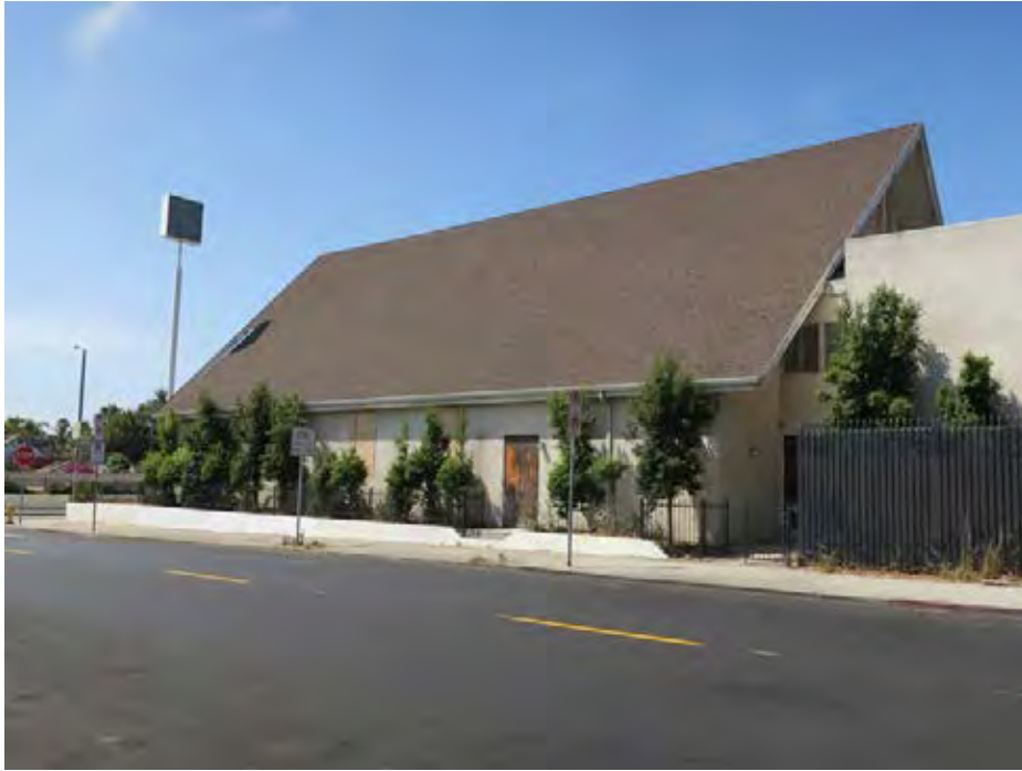
Secondary (east) façade, view southwest (ARG, 2018).
