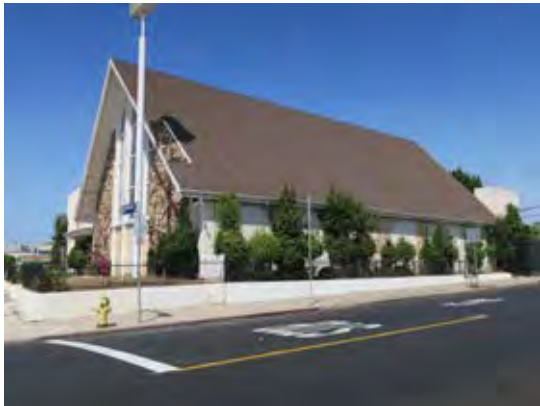
Secondary, east façade, overall view northwest (ARG, 2018).
