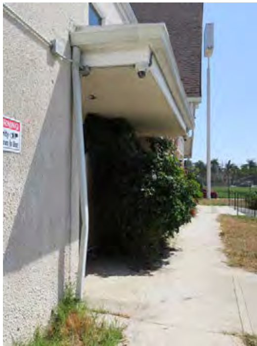
View east at education wing, secondary entrance canopy and walkway (ARG, 2018).
