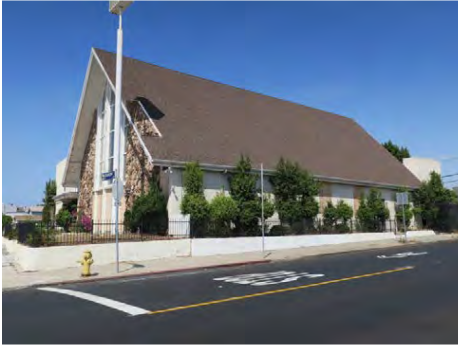
Secondary (east) façade, overall view northwest (ARG, 2018).
