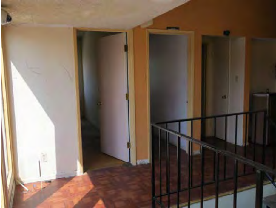
View west in the south second-floor corridor (ARG, 2018).
