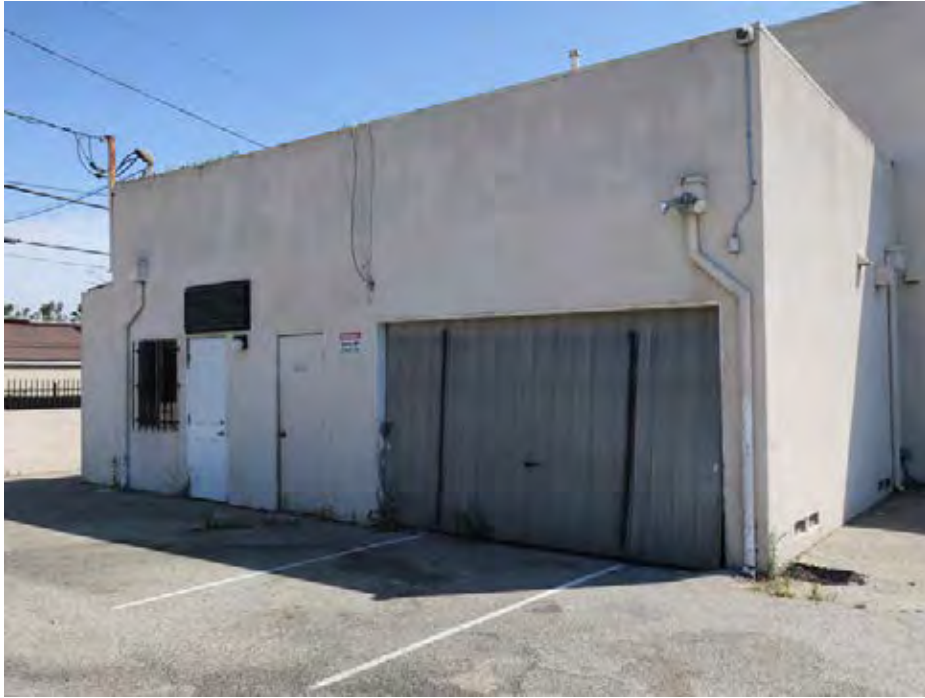
West façade, view northeast at small square addition and garage (ARG, 2018).
