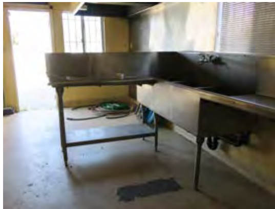
Kitchen, view west (ARG, 2018).
