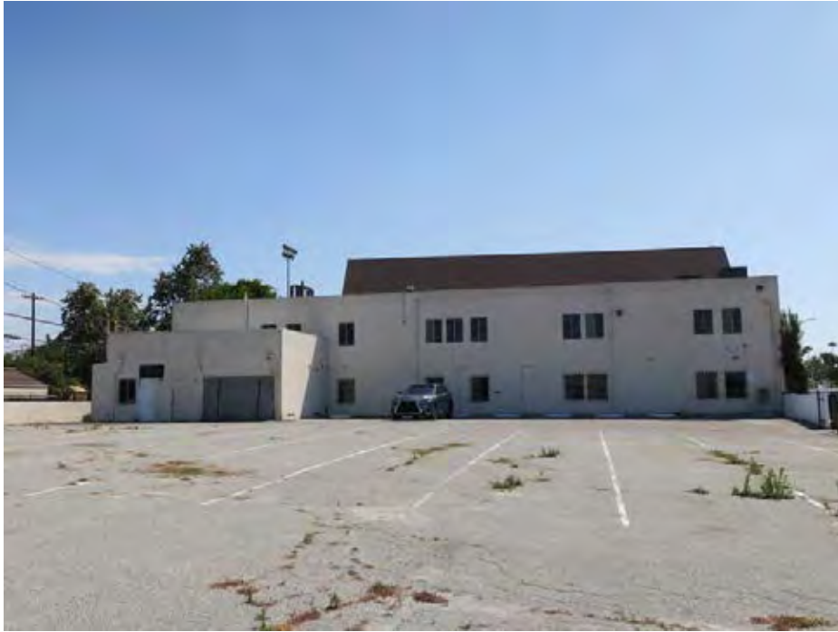
West façade, overall view east across the parking lot (ARG, 2018).
