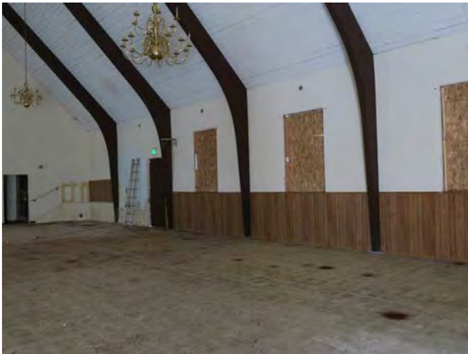
Sanctuary main room, view northeast (ARG, 2018).
