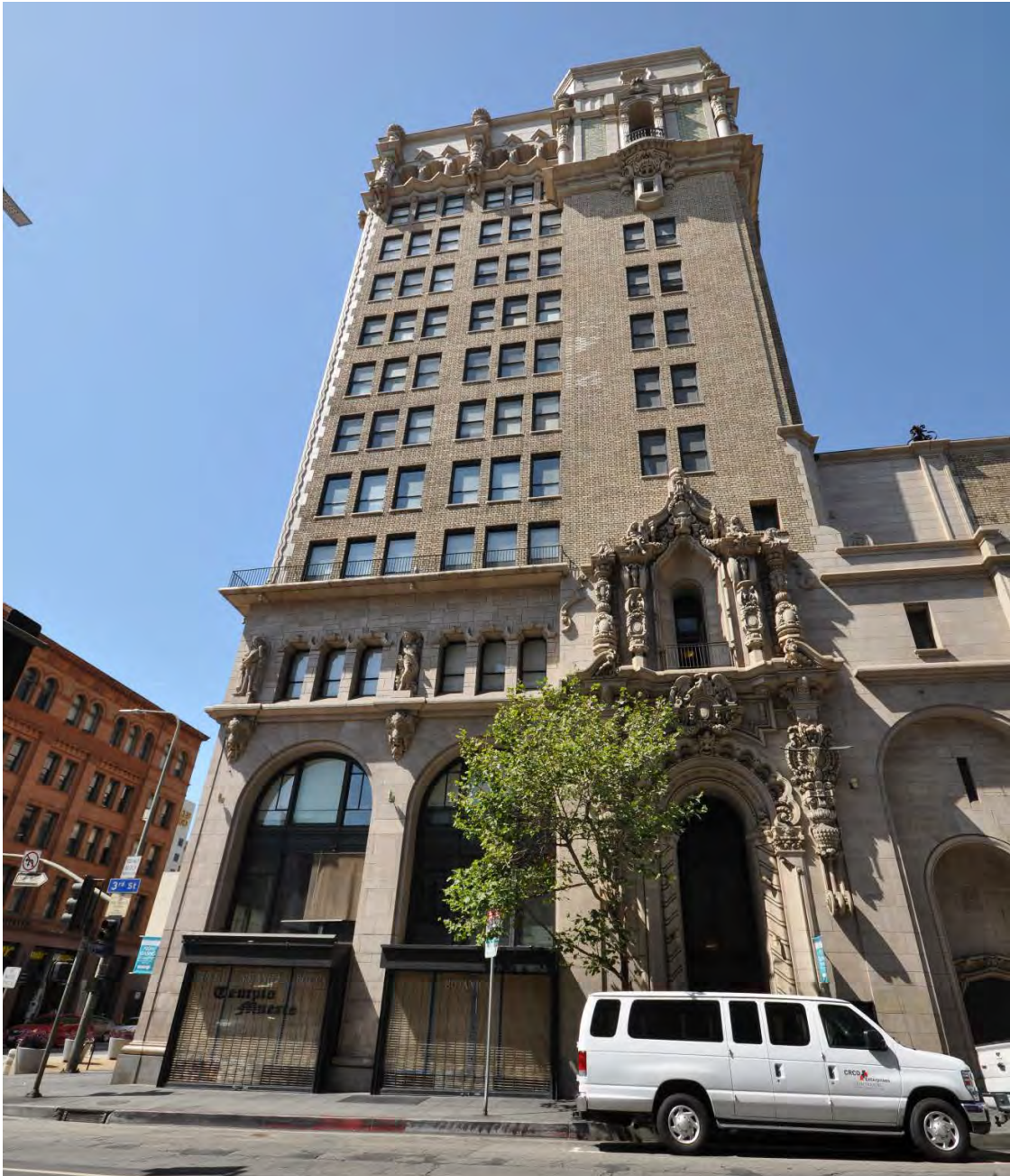
Million Dollar Theater, view of office (now apartment) portion of north elevation. (GPA Consulting, July 2018)
