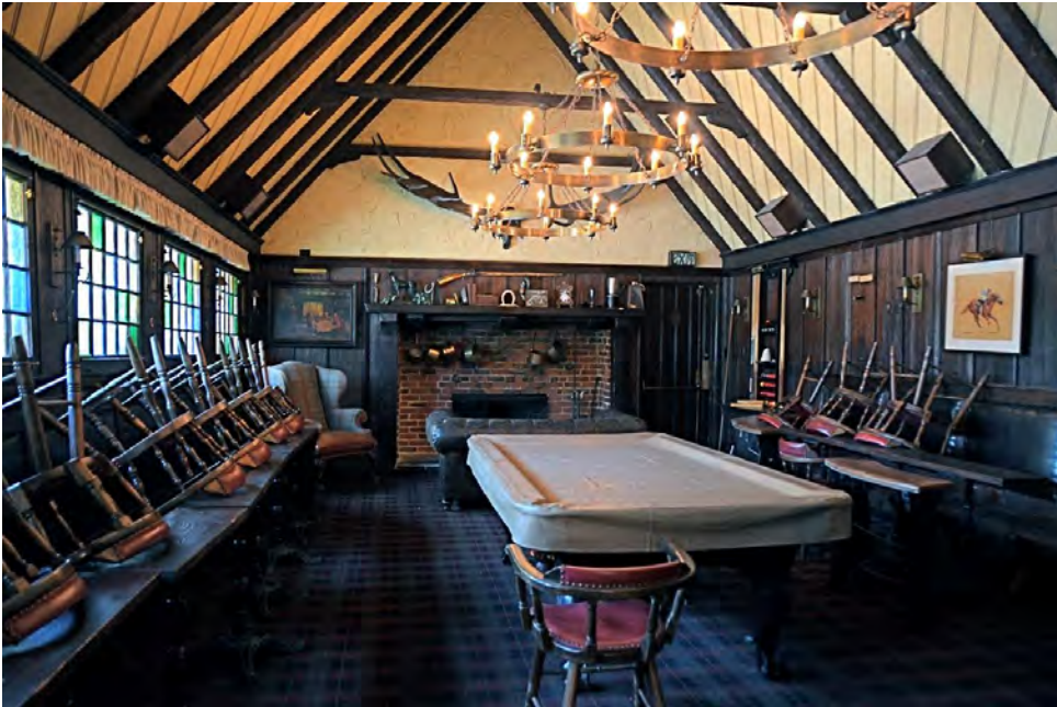
Dining room with exposed rafters, exposed tie beams, and burnished wall panels, view east (ARG, 2018).
