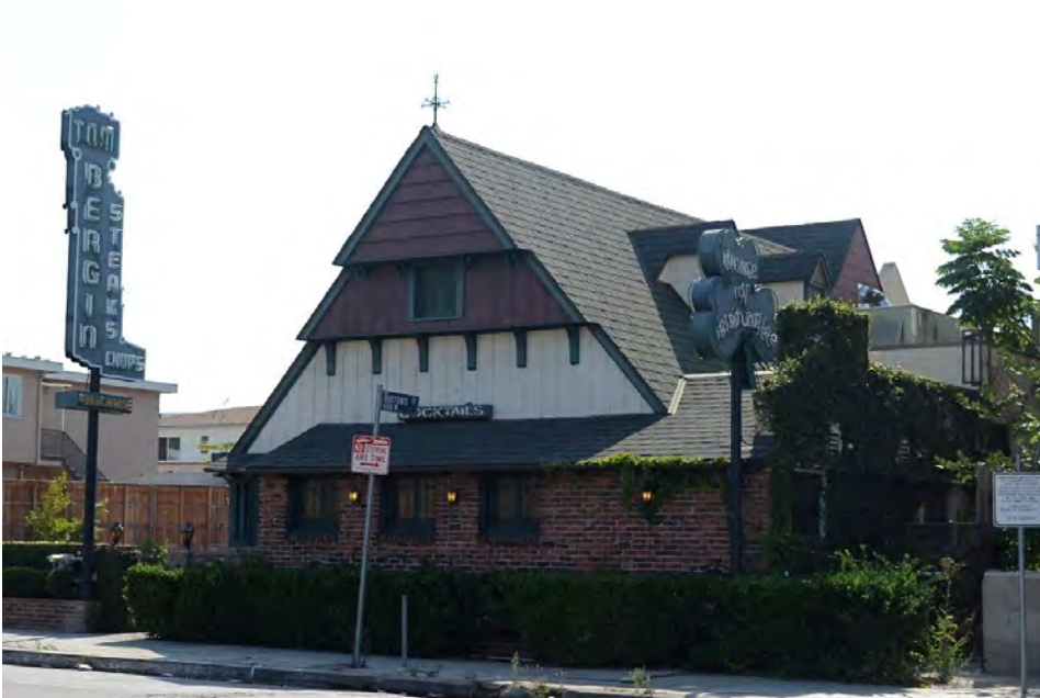
West elevation, view northeast (ARG, 2018).
