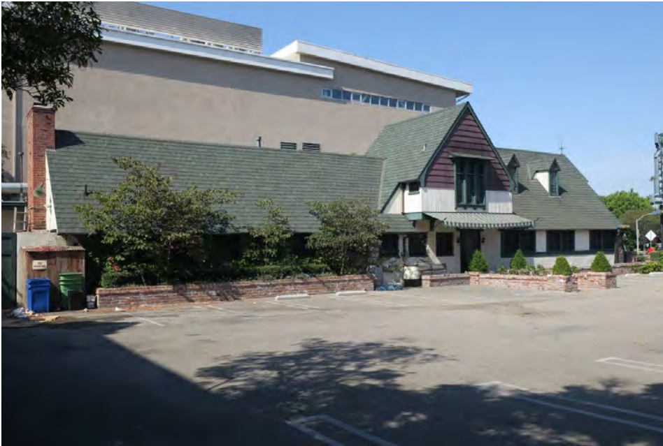
Primary (north) elevation, view southwest (ARG, 2018).
