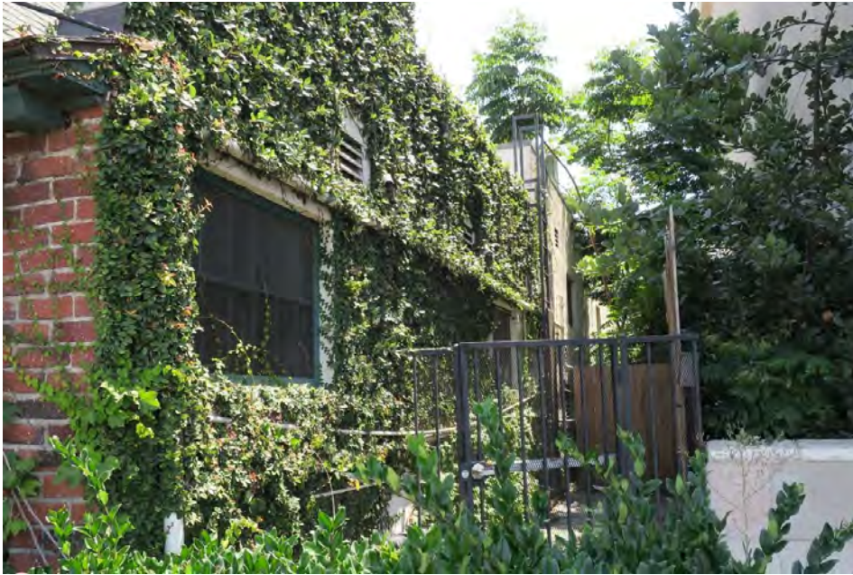
South elevation, view northeast (ARG, 2018).
