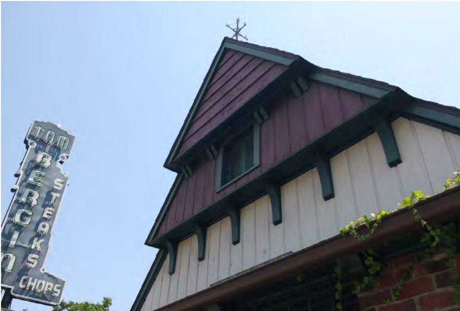
West elevation, detail of jettied gable and decorative brackets (ARG, 2018).
