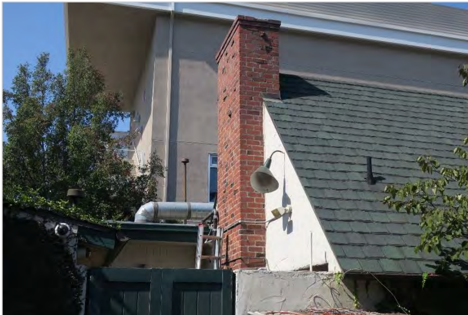
East elevation and chimney, view southwest (ARG, 2018).
