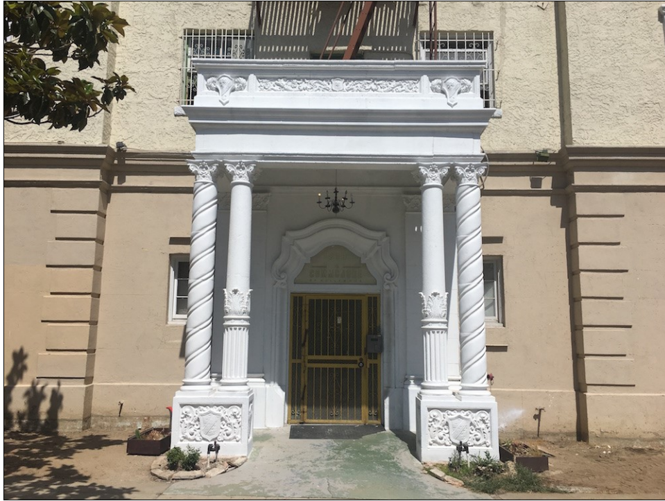
Figure 3: Commodore Apartments, west elevation, entrance detail, view east (source: Snow, 2018)
