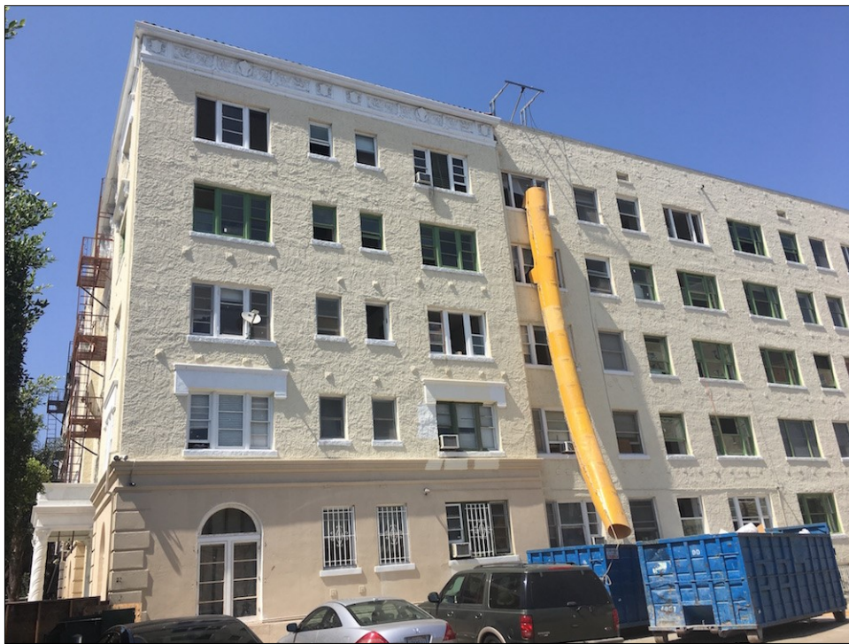
Figure 4: Commodore Apartments, south elevation, view northeast (source: Snow, 2018)
