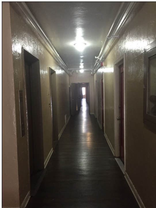
Figure 7: Commodore Apartments, interior, 1st floor corridor, view east (source: Snow, 2017)
