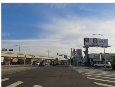
Figure 13 – View of Project site and Expo Line from the intersection of Gateway Blvd and Exposition Blvd, looking east
