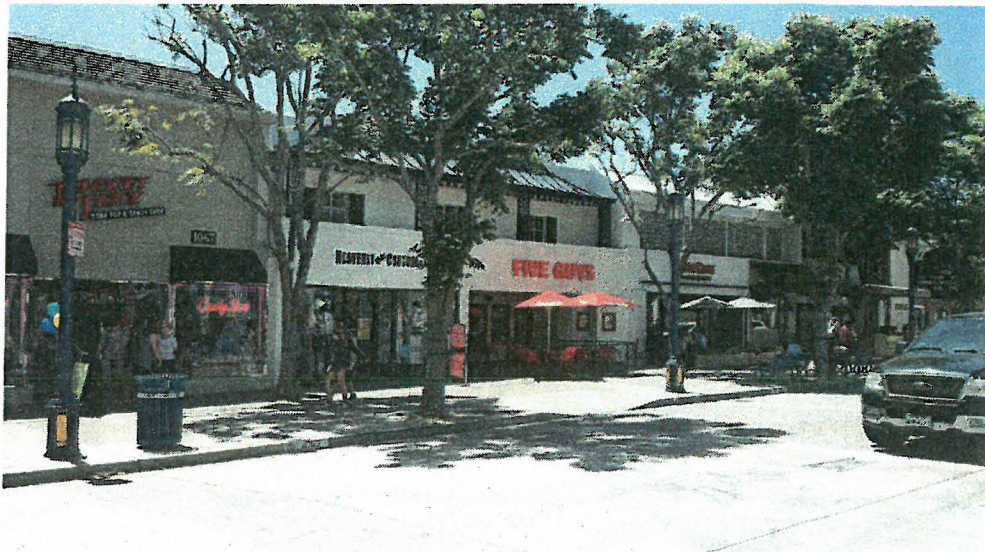
2. Subject site and abutting properties
