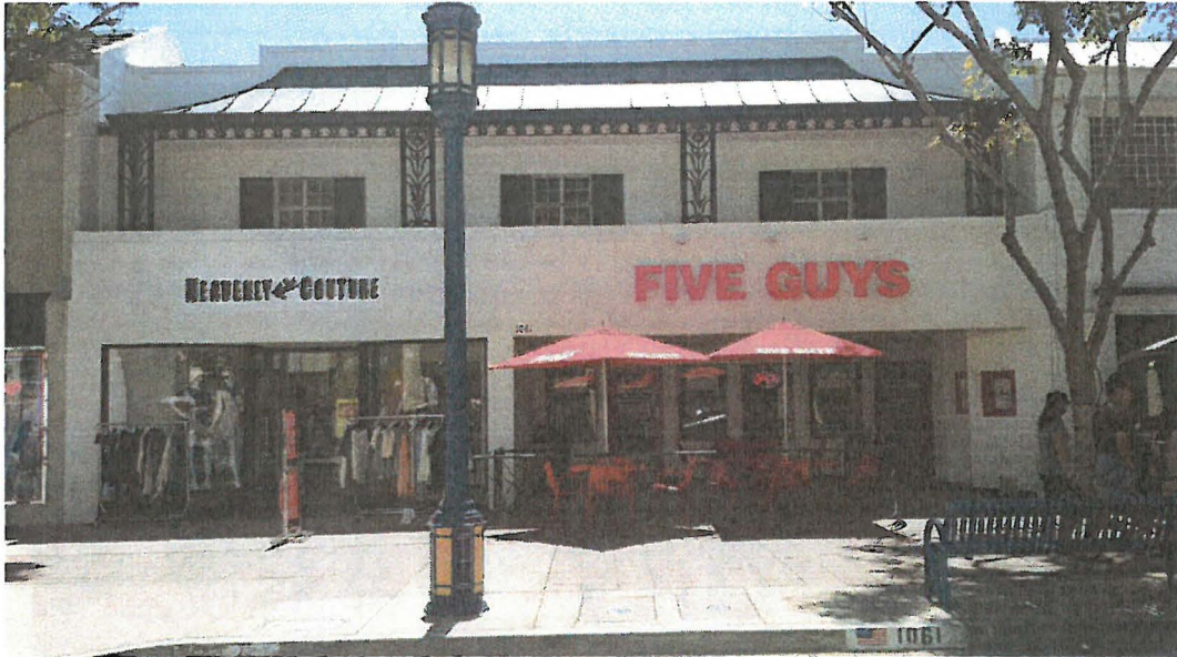
3. Front view of subject site
