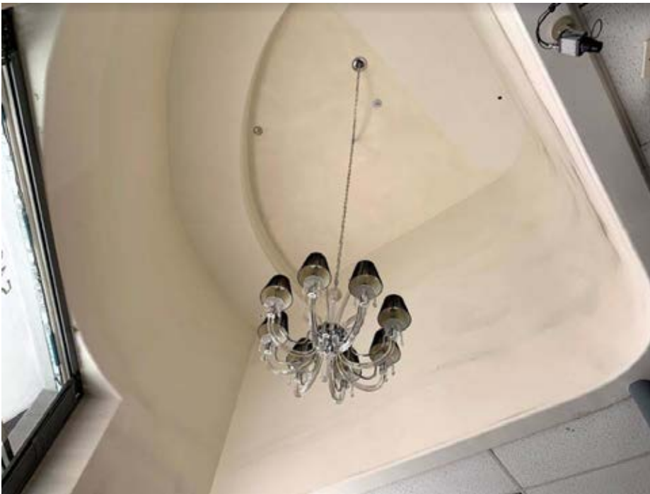
Detail of curved wall and tray ceiling at primary entrance (Steven Luftman, 2020)
