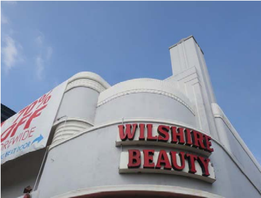
Primary (south) façade, detail of rounded corner, articulated parapet, and roof tower (ARG, 2020)
