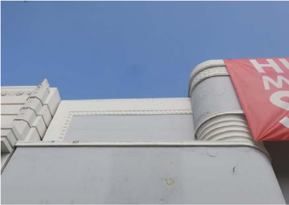
Primary (south) façade, detail of parapet, rounded corners , and grooved moldings (ARG, 2020)
