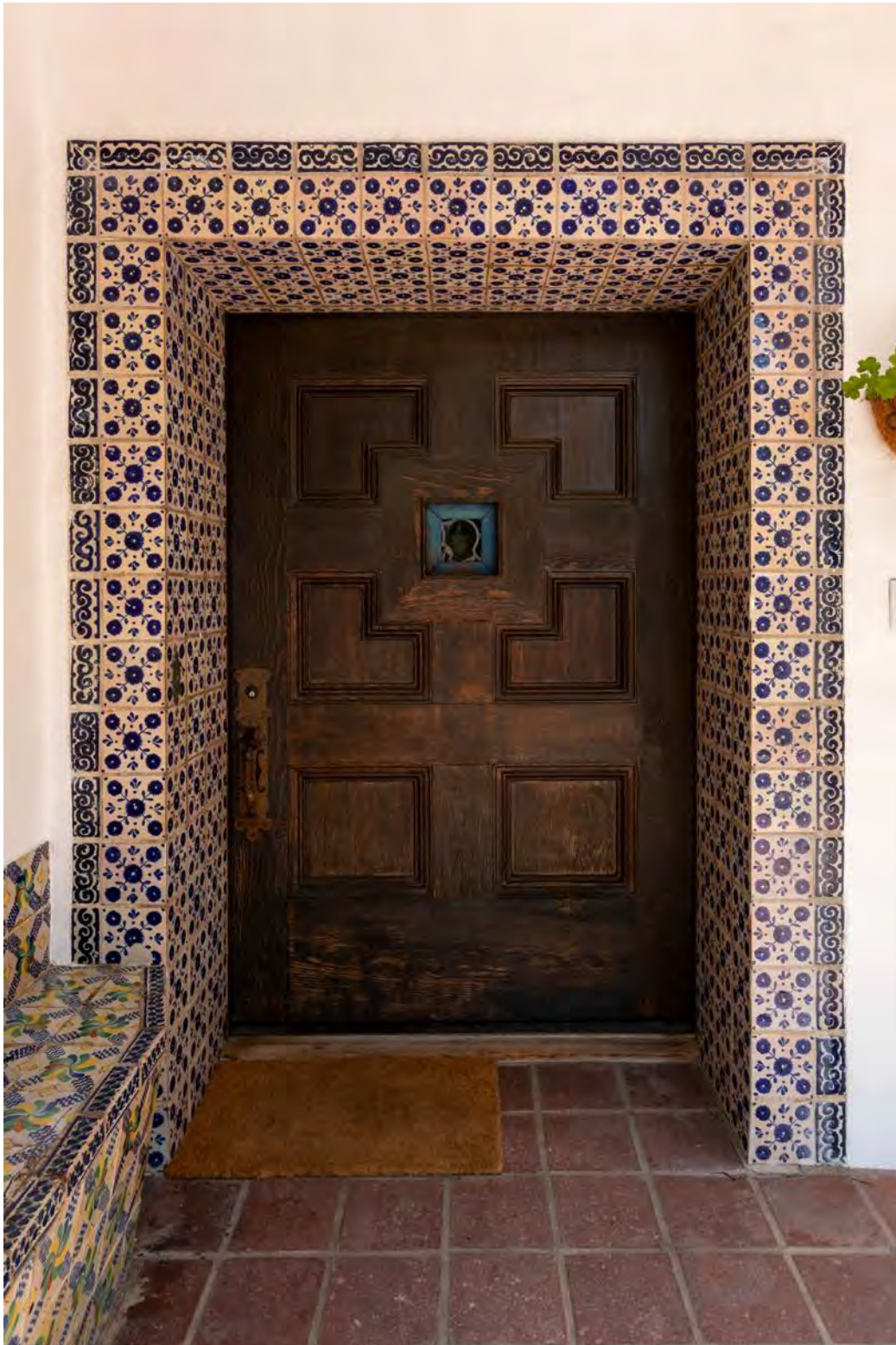
Primary entrance door, view looking north.
