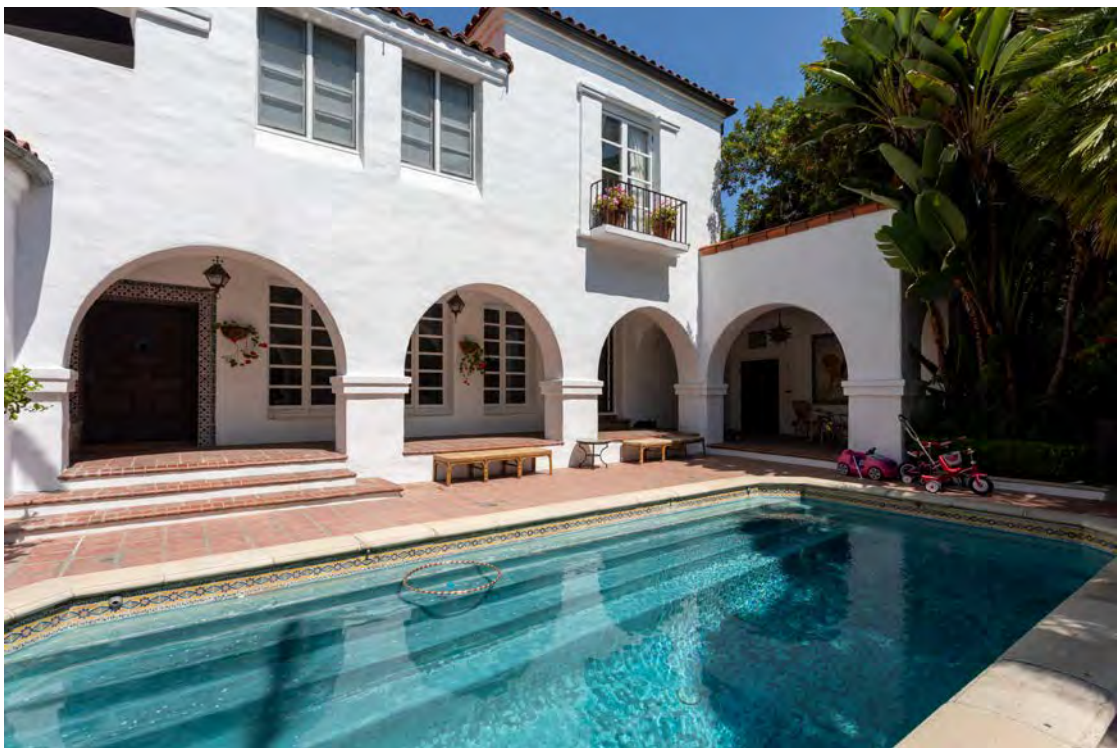
Primary (south) façade, view looking northeast.
