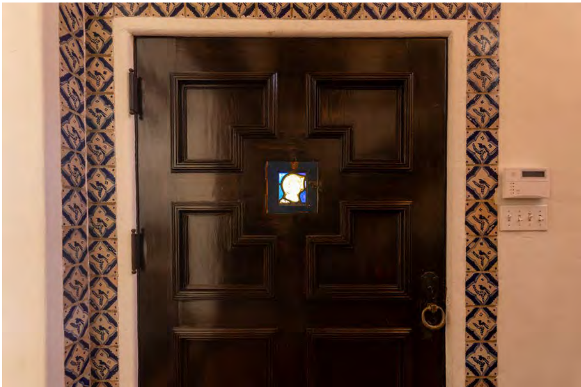
Primary entrance door.
