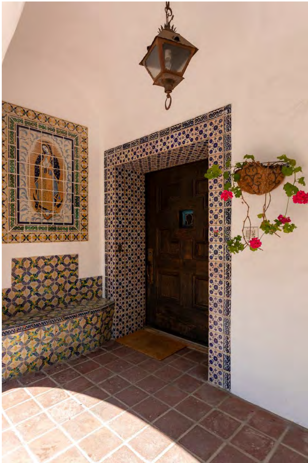
Primary entrance, view looking northwest.
