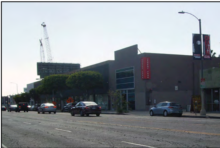
View 5: From the east side of La Brea Avenue, looking southwest at the Project Site.
