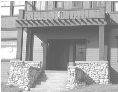
Riverrock helps define this porch.
