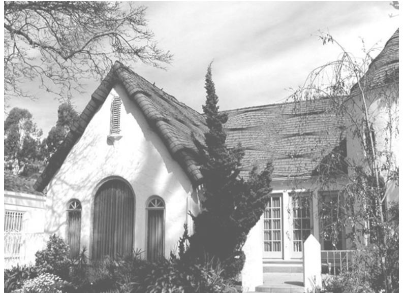
Built-up faux thatch shingle roof
