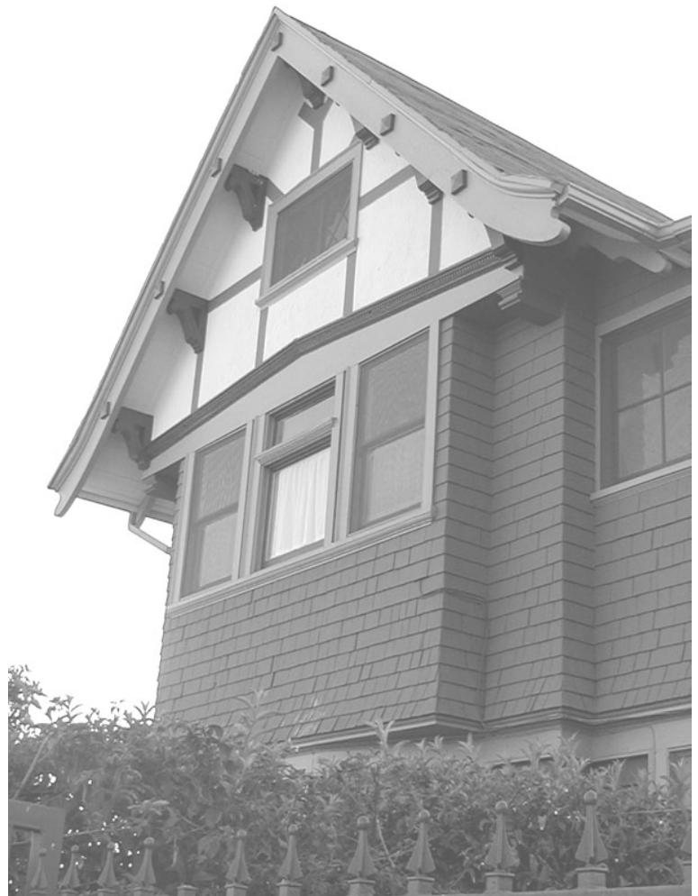
Stucco, half-timbering, and wood shingle
