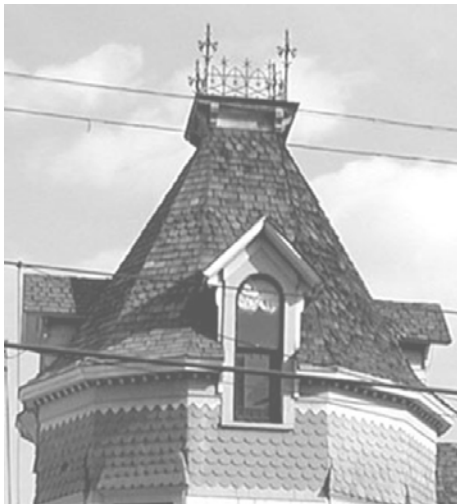
This roof combines decorative ironwork and decorative wood shingles.
