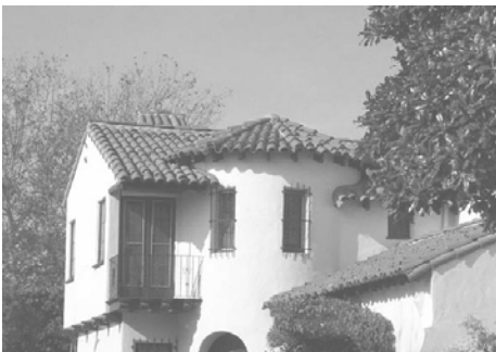
Complex roof plan with terra-cotta tile
