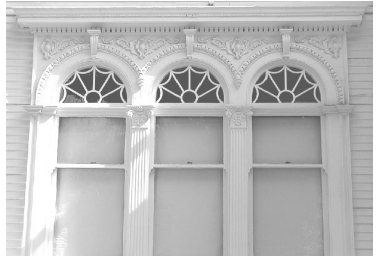
Triple double-hung one-over-one wood windows with decorative fan lights
