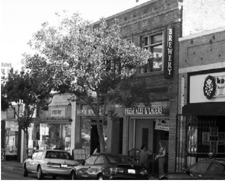
Appropriate new signage on historic commercial structures.
