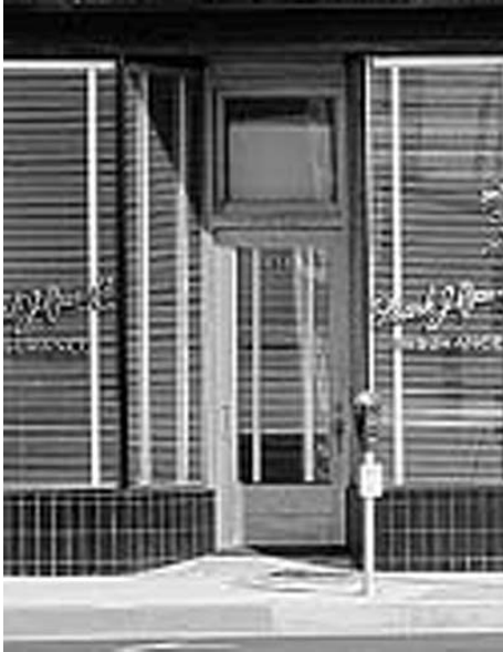
Glazed door with transom above.
