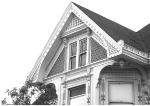
Important elements of your historic roof that must be preserved include the roof form, the eave and cornice design, and any decorative or structural details which contribute to the style of your house.
