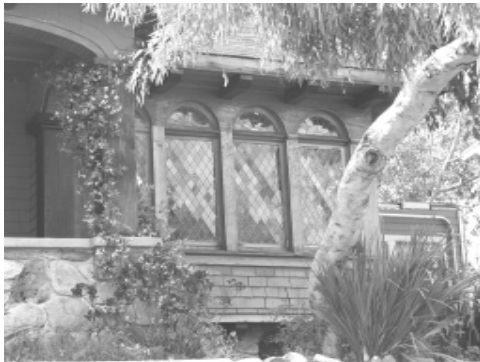
Preserve the materials and design of historic windows and their surroundings, including hardware.
