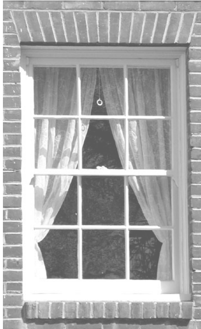
Six over six wood double-hung window
