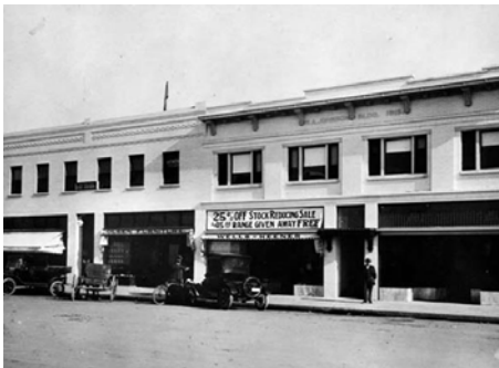
Cornice details help distinguish commercial buildings.
