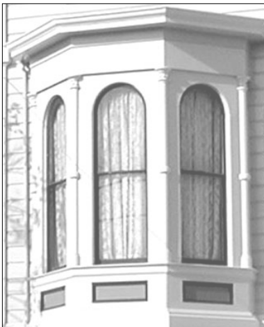
Rounded-top double-hung wood bay windows
