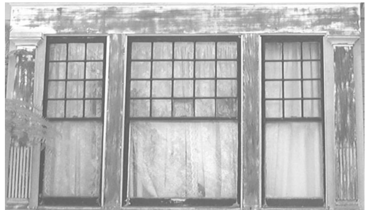
Twenty-over-one wood double-hung window flanked by two twelve-over-one double-hung windows
