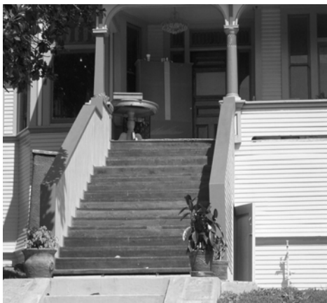
Original steps should be preserved. If the steps are so deteriorated they need replacement, they should be replaced utilizing the historic material.
