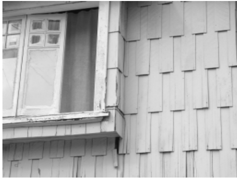
Wood siding is generally smooth sawn and not textured.
