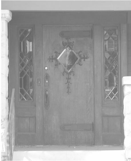
Loss of this door and its sidelights would have a negative effect on the character of this house.
