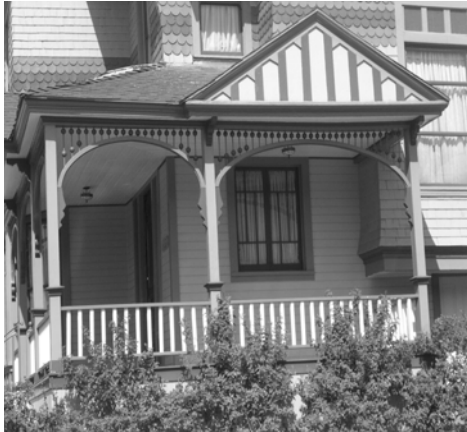
Decorative details that help to define a historic porch should be preserved. These include balusters, balustrades, columns, and brackets.
