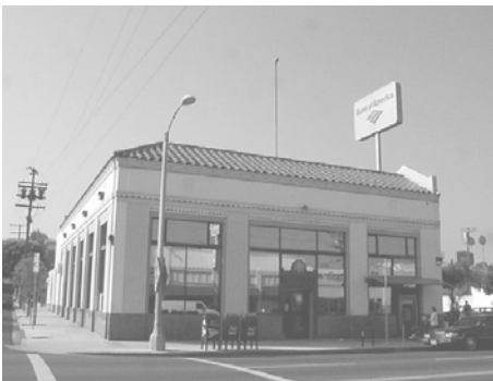
Filling in storefront windows dramatically changes the character of a commercial building
