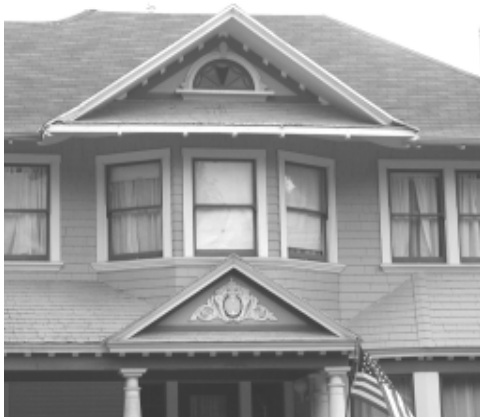
Original architectural features shall be preserved.
