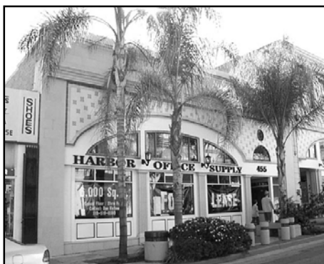
Replacing traditional historic windows with aluminum sliding windows like these is inappropriate.
