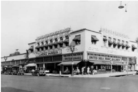
Historic signage was located primarily in the band above the storefront windows.
