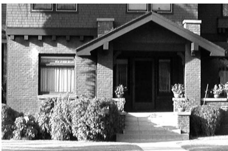
This Craftsman porch is dominated by its strong roof-line.
