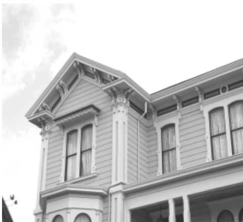
Architectural Detail of the Foy House
