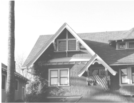
Complex multi-gabled roof with composition shingle
