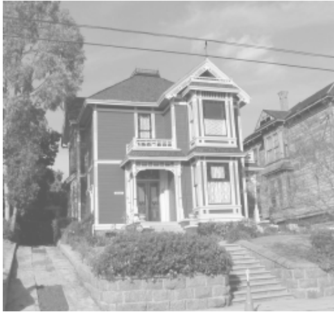
Historic stone retaining walls and steps.
