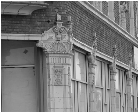
Glazed terra cotta tile detail was common in the early twentieth century on commercial buildings.
