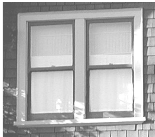
Paired double-hung wood windows
