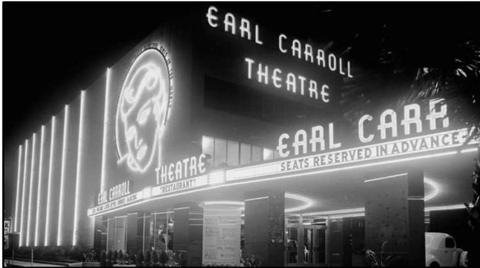
Earl Carroll Theatre Preservation and Façade Restoration Overview
