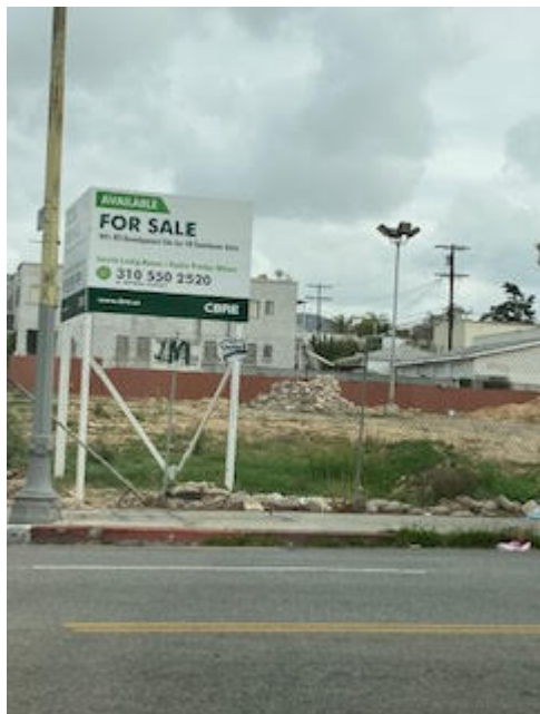
Photographs of 4 apartment construction sites on Hollywood Blvd between Hillhurst and Edgemont
